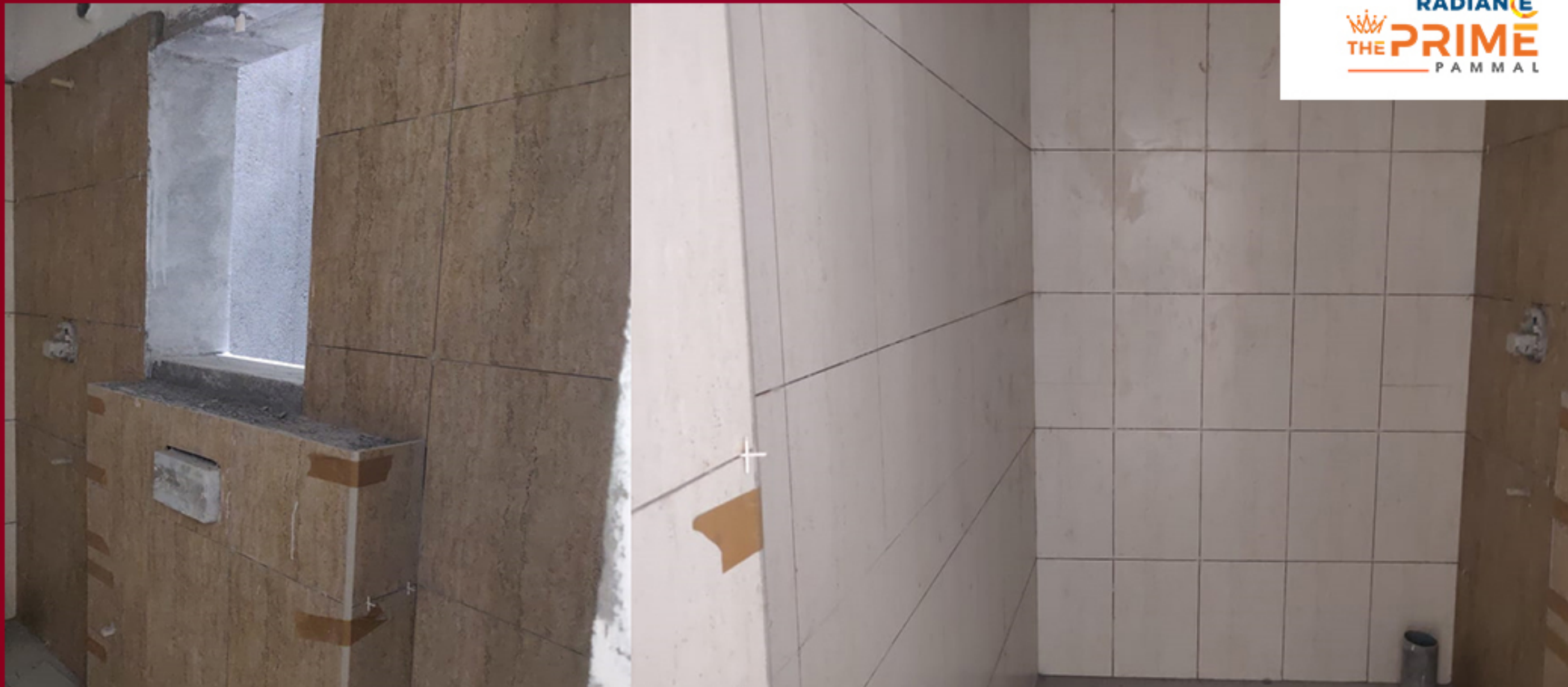
BLOCK 3 -CLUSTER H UP TO 2ND FLOOR TILE WORK IN PROGRESS
