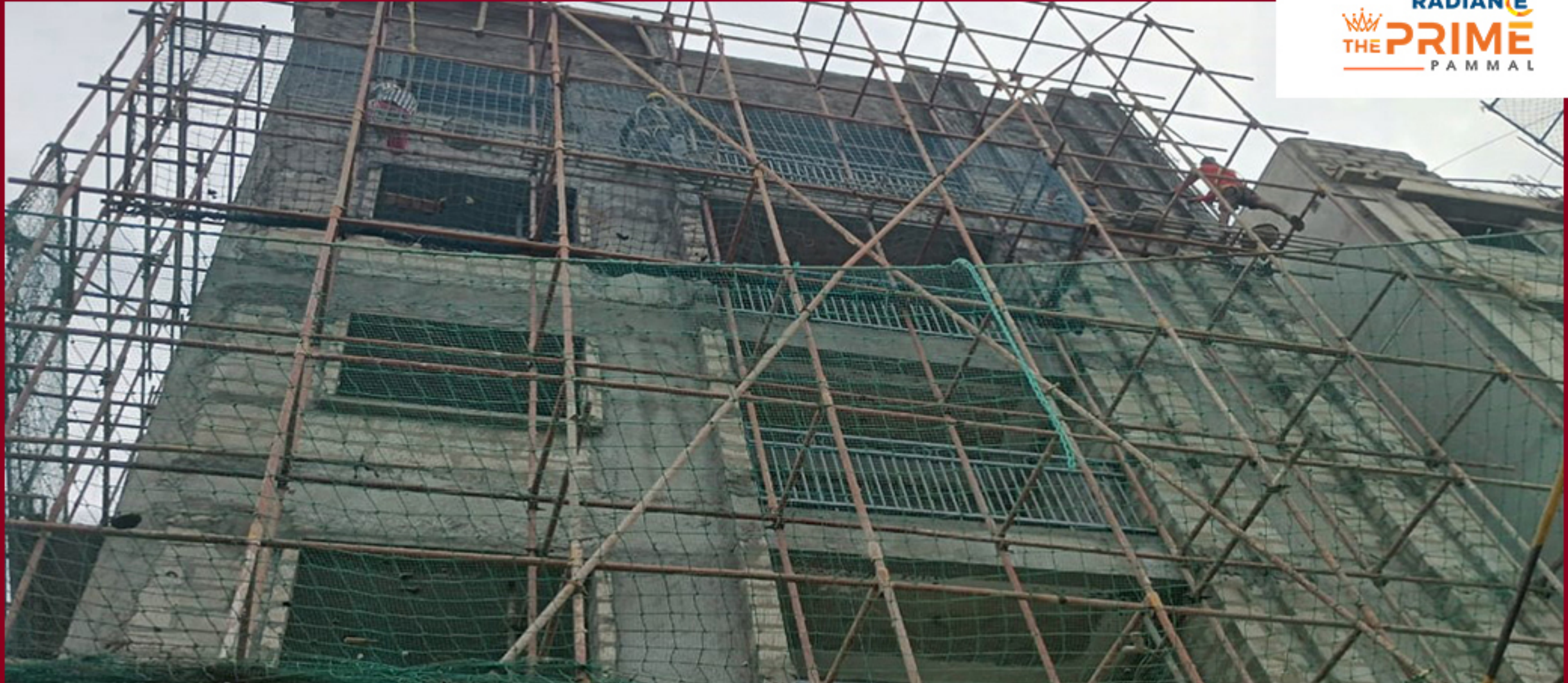
BLOCK 1 - CLUSTER D SOUTH SIDE EXTERNAL PLASTERING WORK IN PROGRESS
