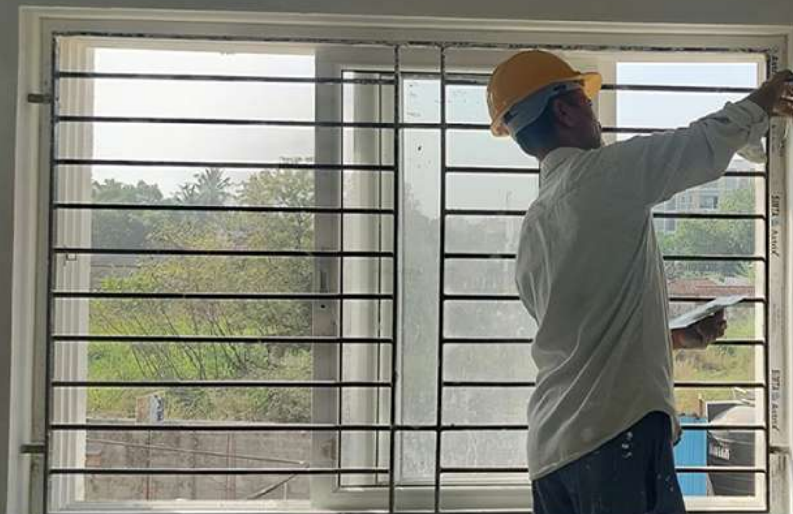
Block 1 –Cluster D Touchup Work In Progress
