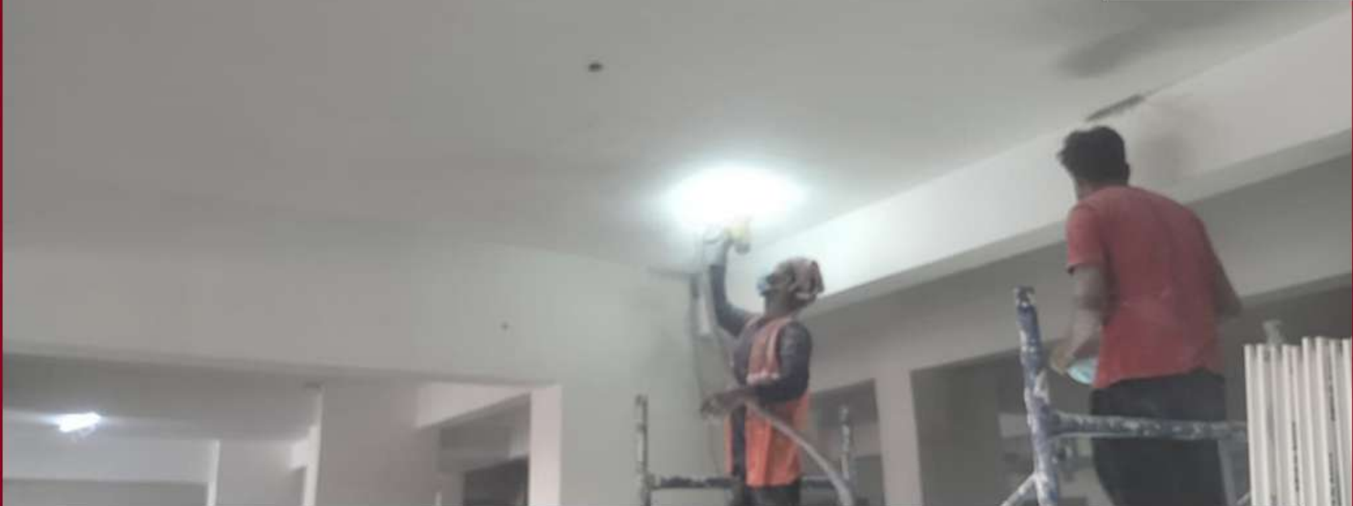
Block 1 Stilt Floor Painting Work In Progress
