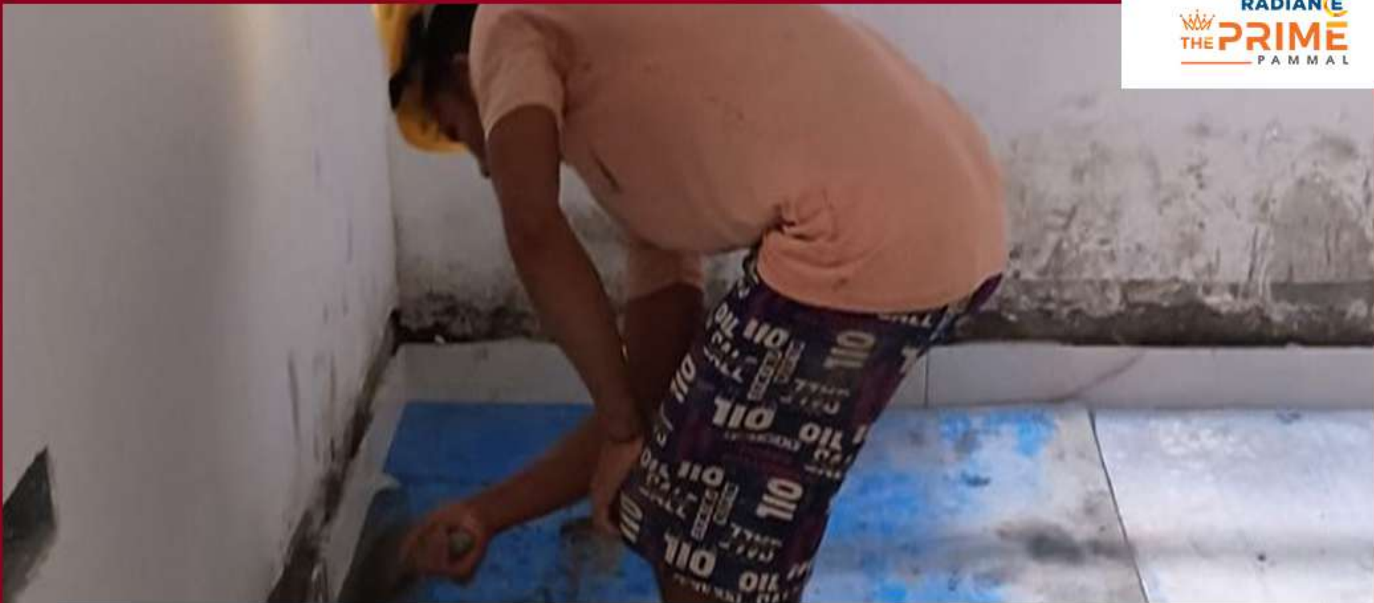
Cluster E Above Skirting Plastering Work in Progress
