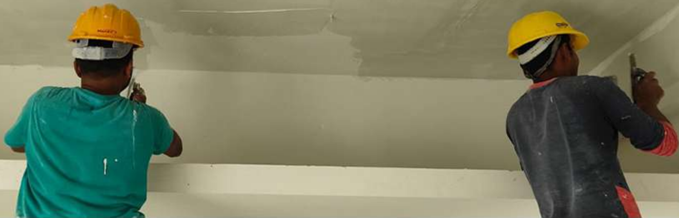
Block 1 –Cluster A Putty work In Progress
