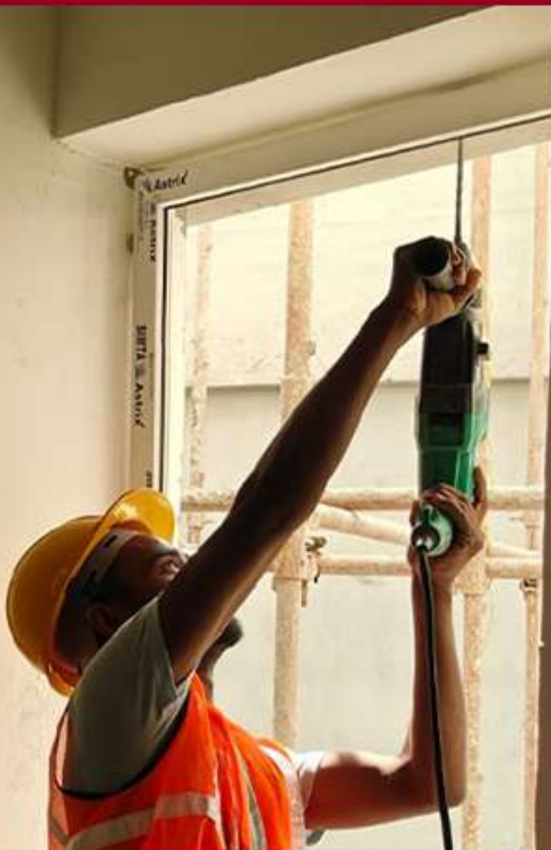
Block 1 –Cluster A UPVC Fixing work In Progress
