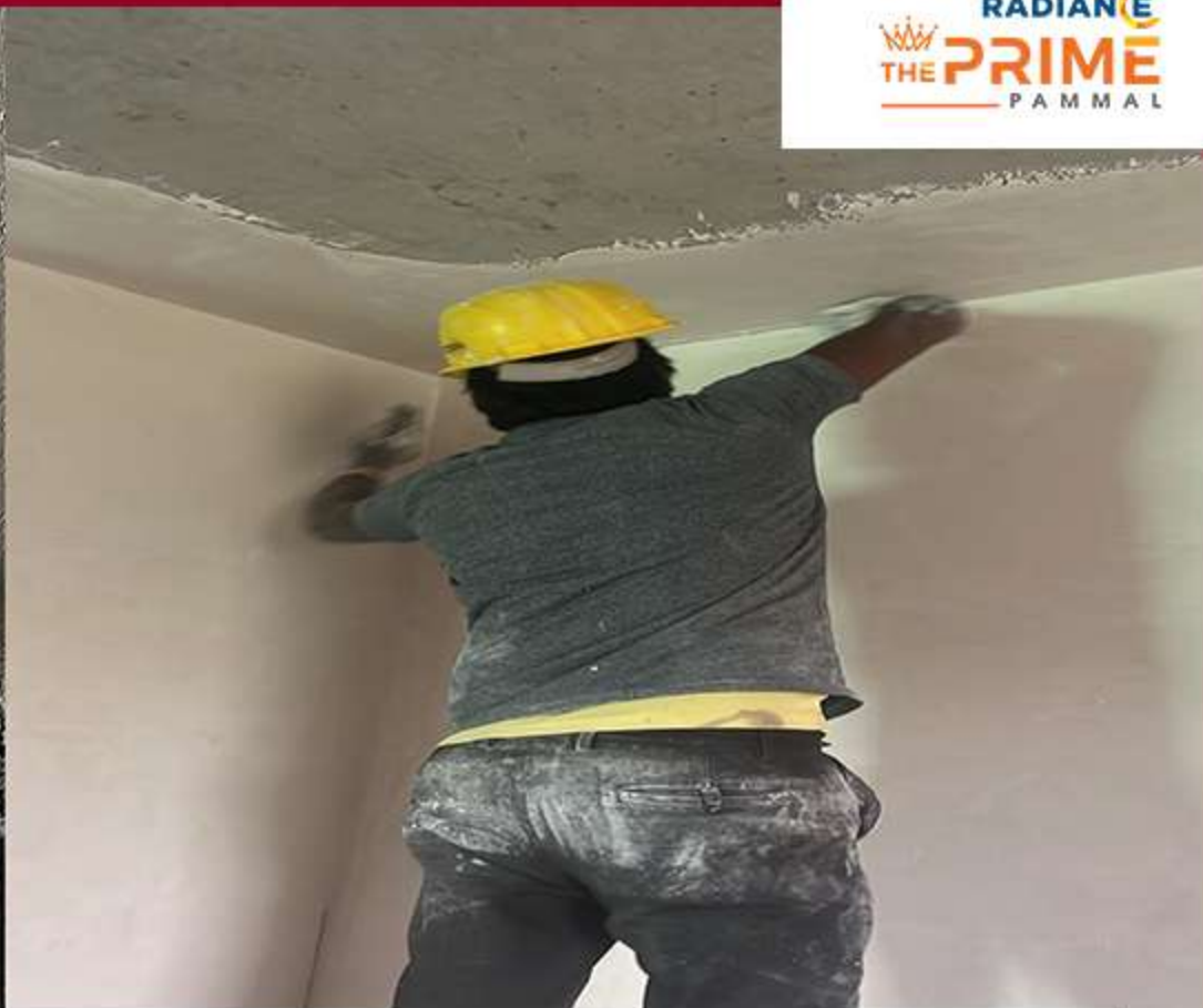
Block 1 – cluster a internal plasteringwork in progress.
