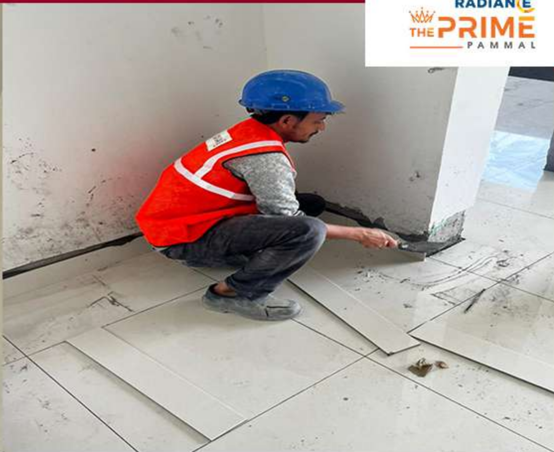
Block 1 – cluster B tile work in progress.
