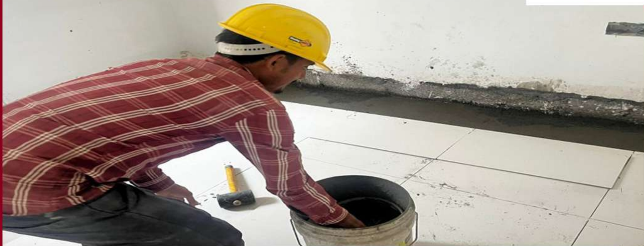
Block 1 – cluster b 1st floor tile work in progress.
