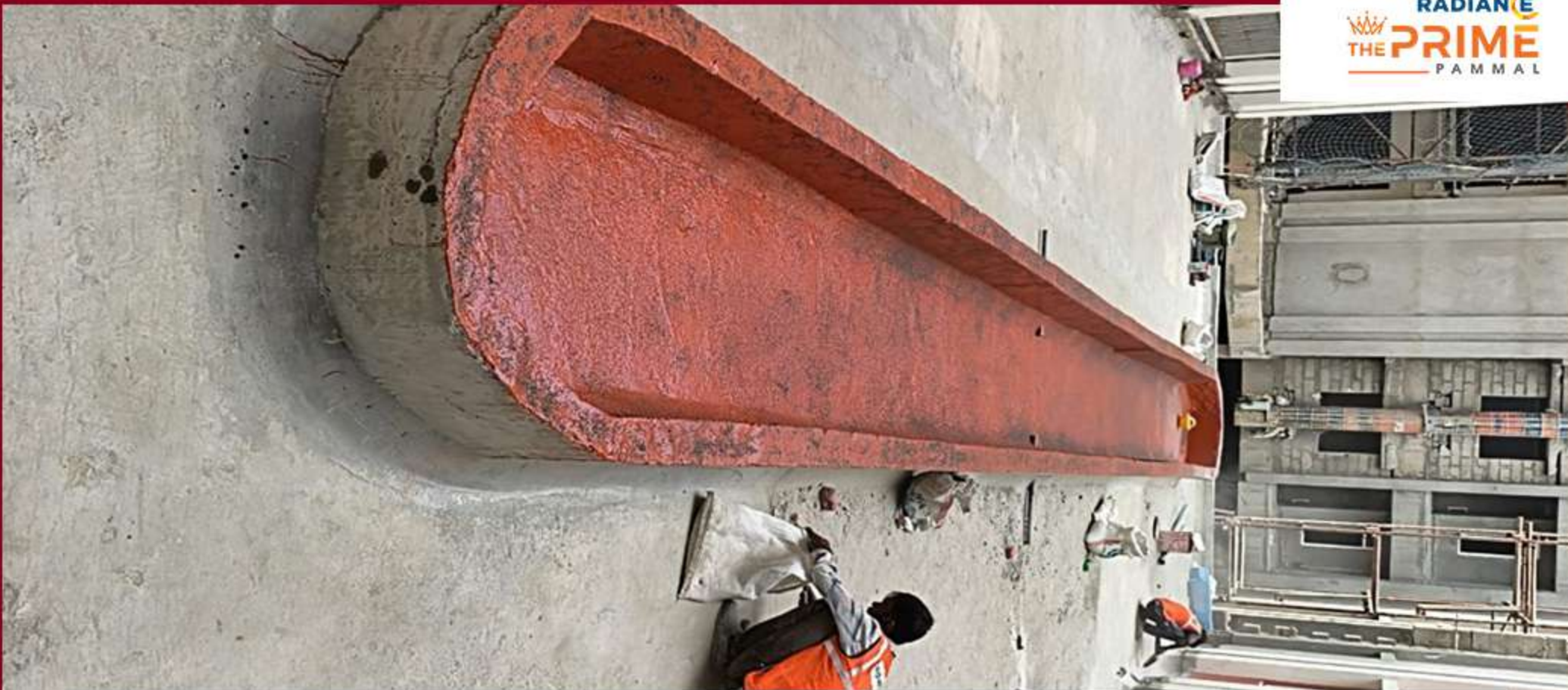
Block 3 – Cluster H & J podium waterproofing work in progress.
