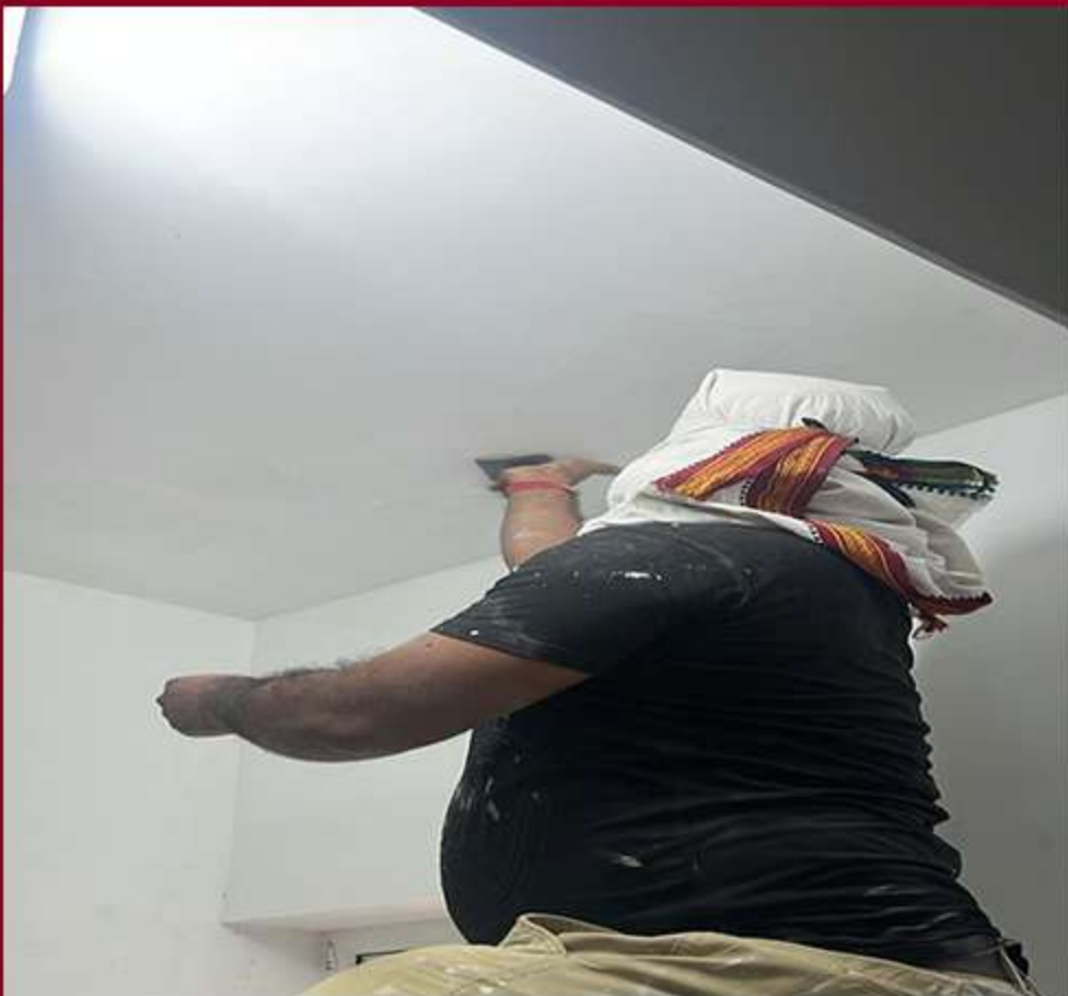
Block 1 – cluster a putty work in progress.
