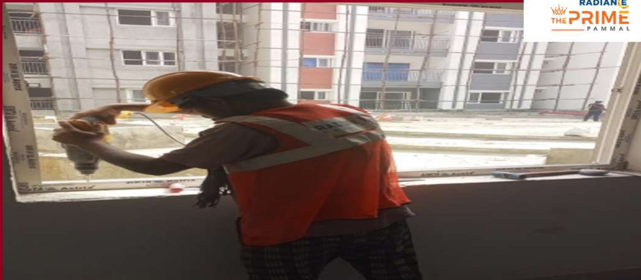
Block 1 – Cluster C upvc window fixing work in progress.
