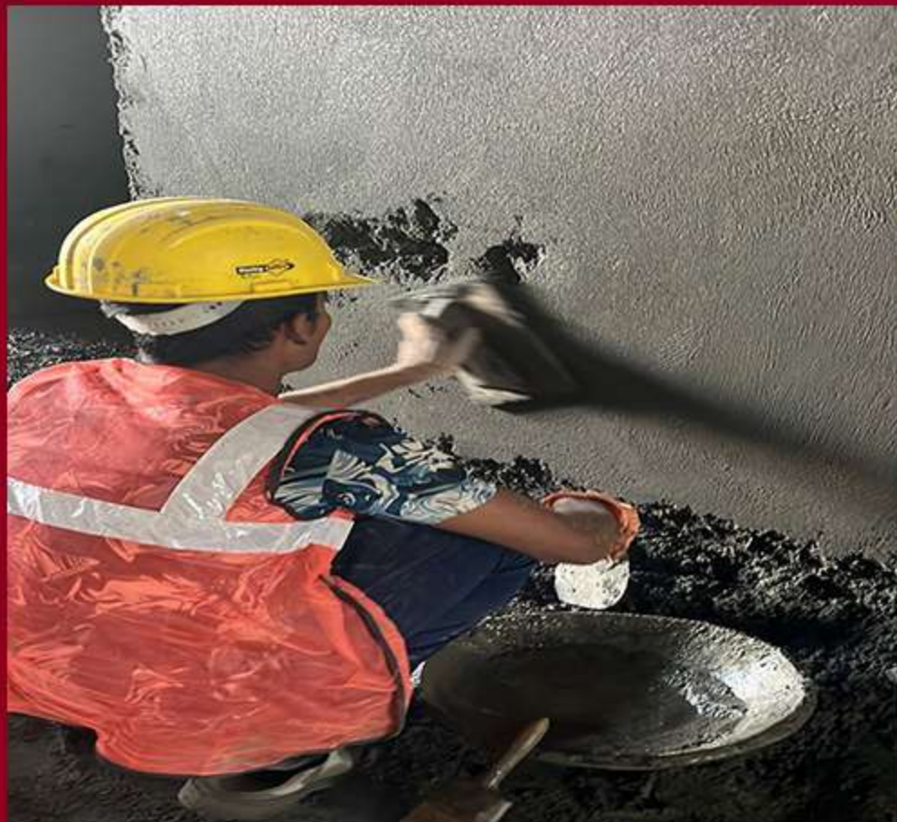
Block 1 – cluster a internal plasteringwork in progress.
