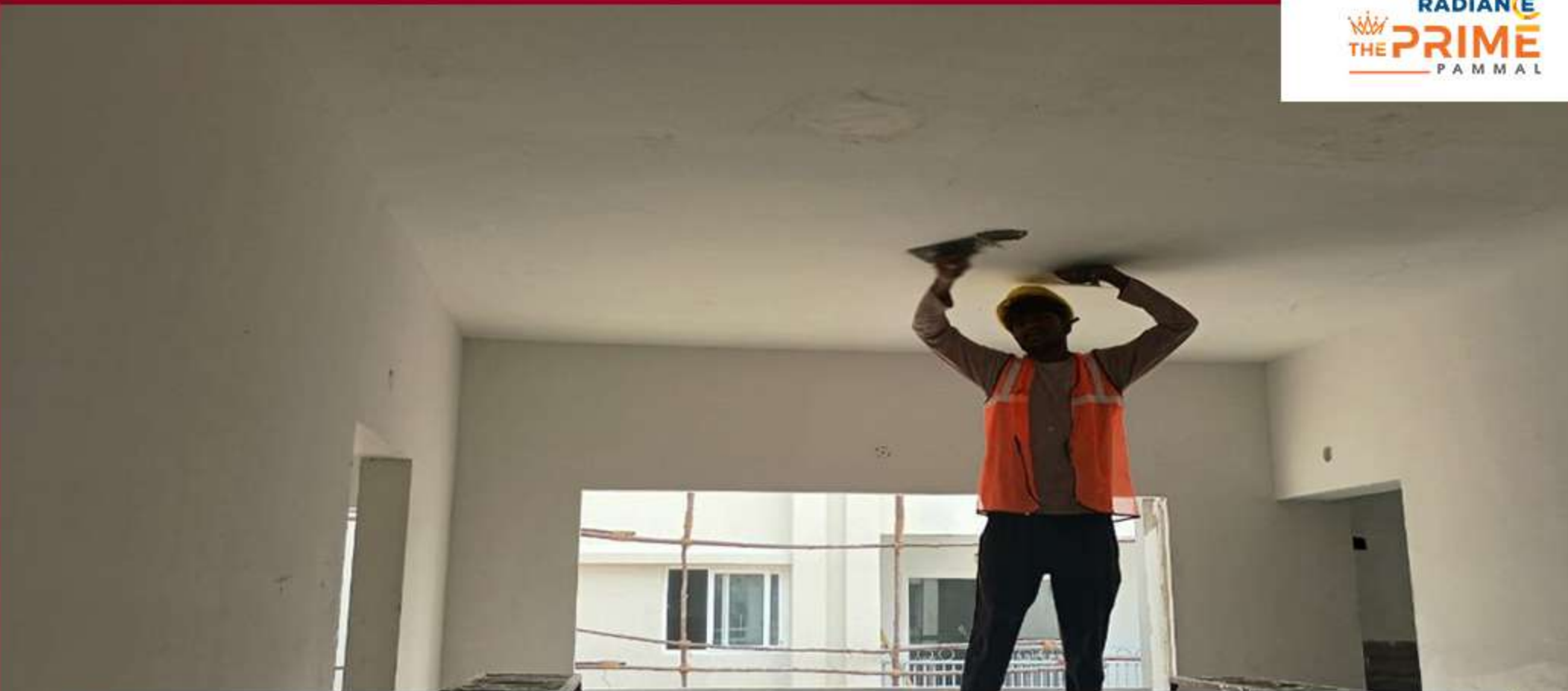
Cluster e ceiling & wall putty work in progress.
