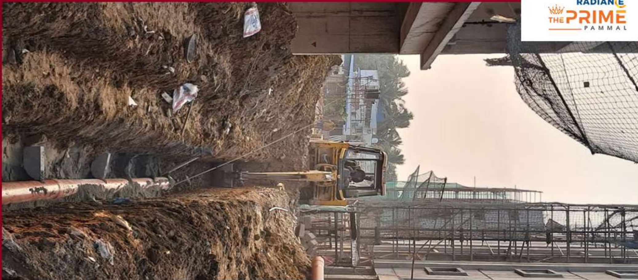
External sewage pipe laying work in progress.
