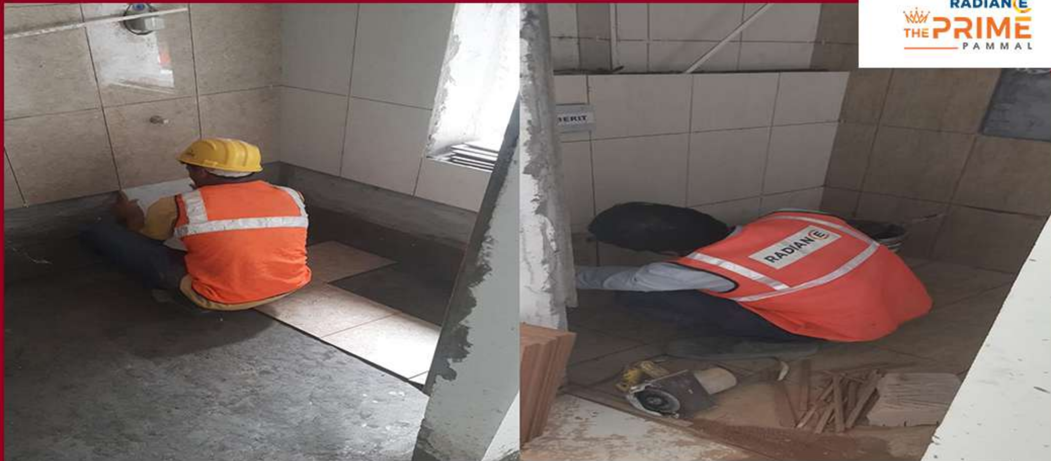
Block 1 – Cluster D Tile Laying Work In Progress.
