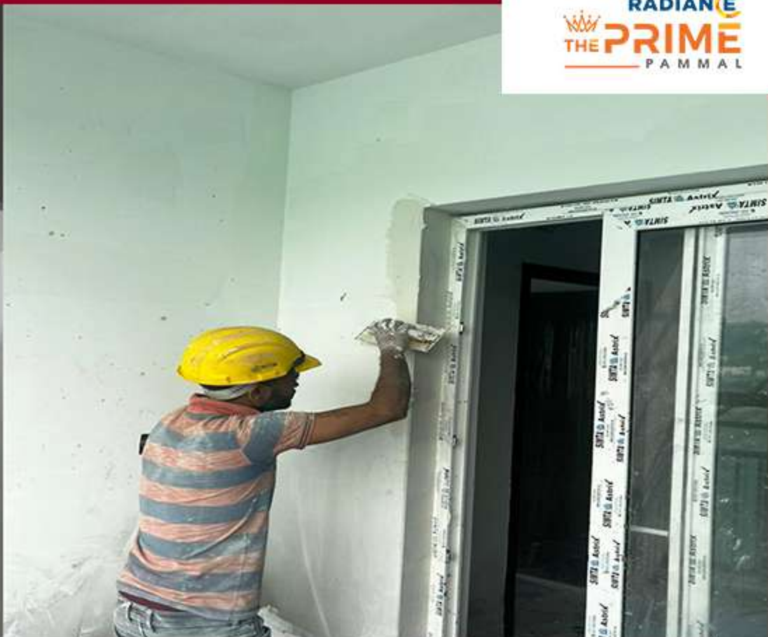
Block 1 – cluster a putty work in progress.
