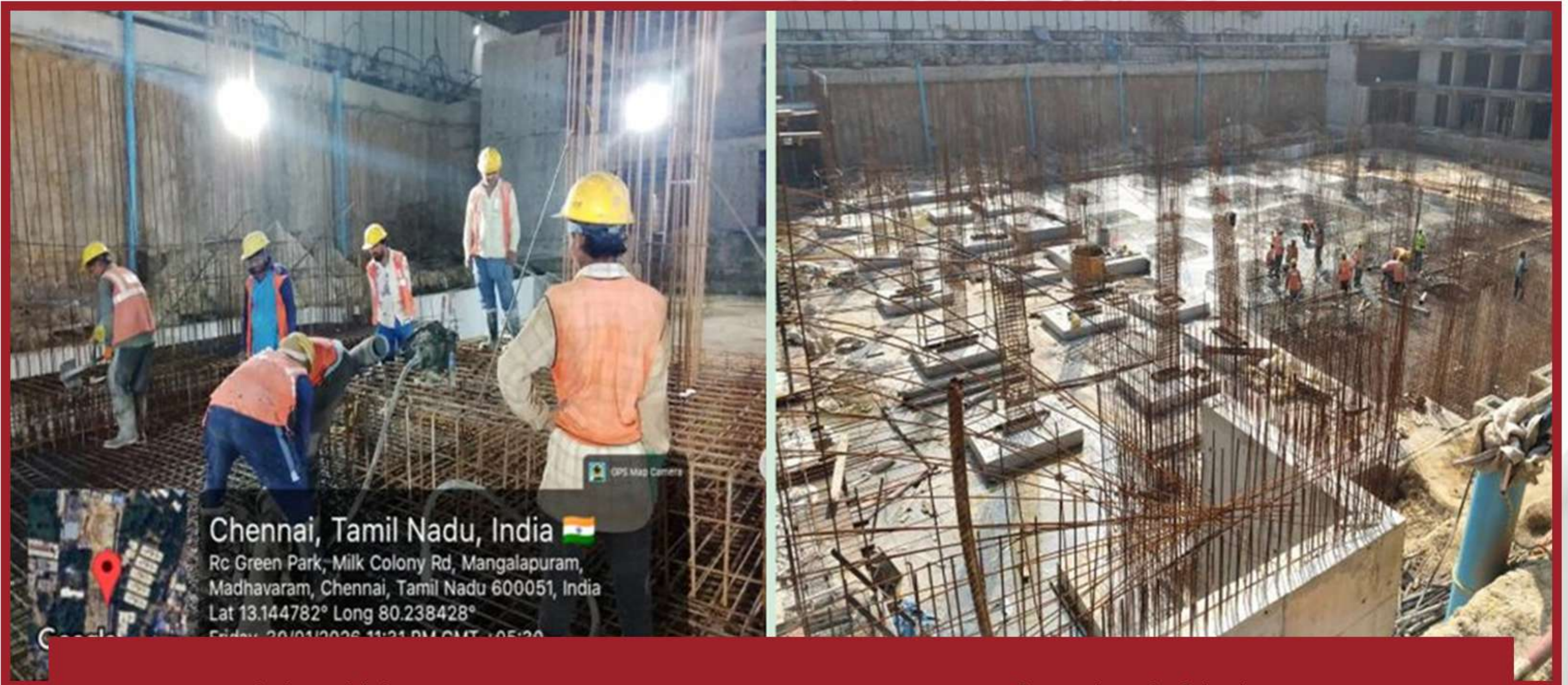
Block D / Club house –excavation COMPLETED & RAFT PCC COMPLETED waterproofing works and raft-level rcc WIP
