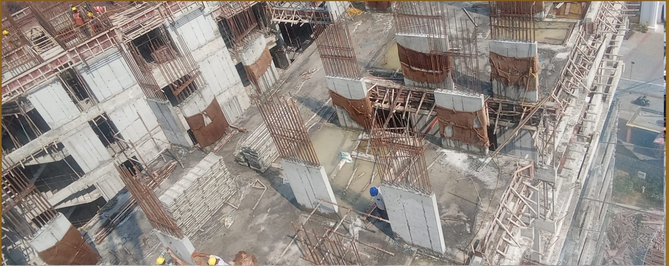
Block-b 10th floor column concrete work pour-2
