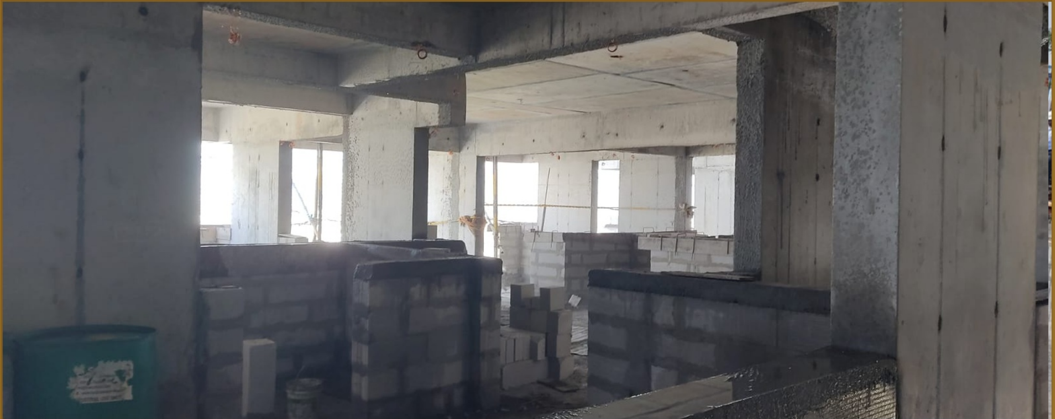
Block b -6th floor block work
