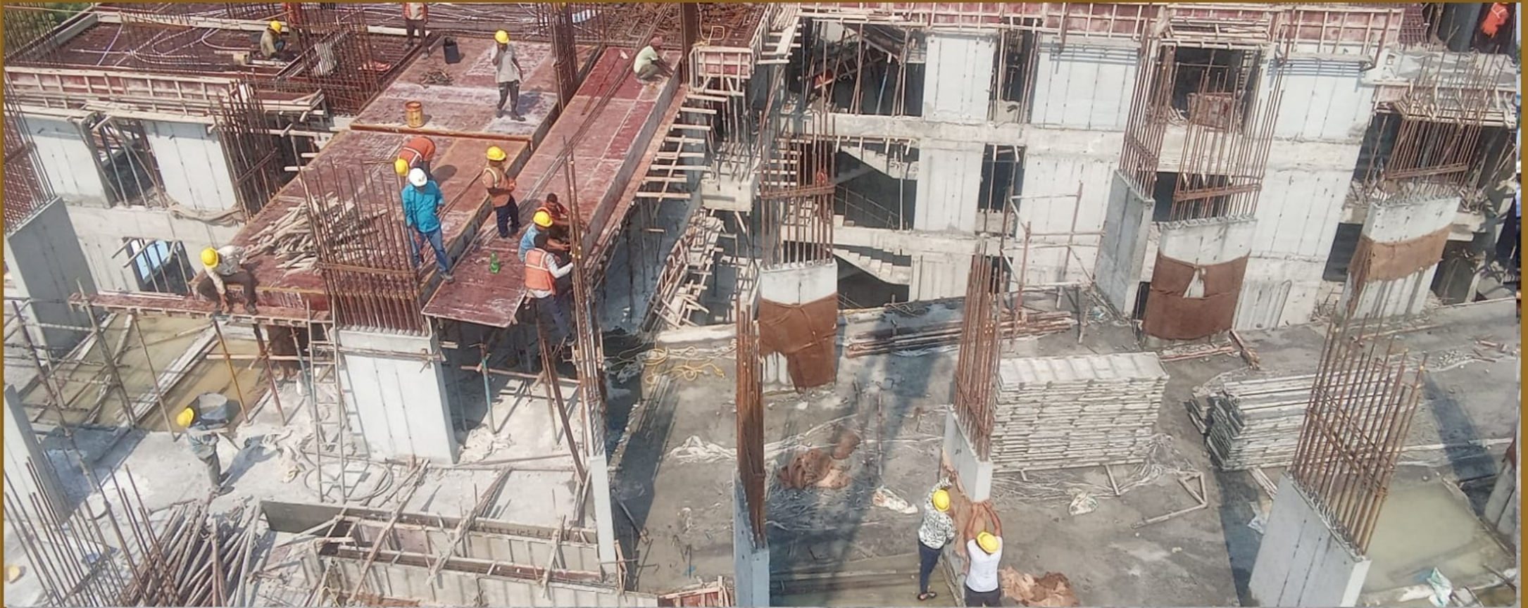
Block-b 10th floor roof slab shuttering work pour-1
