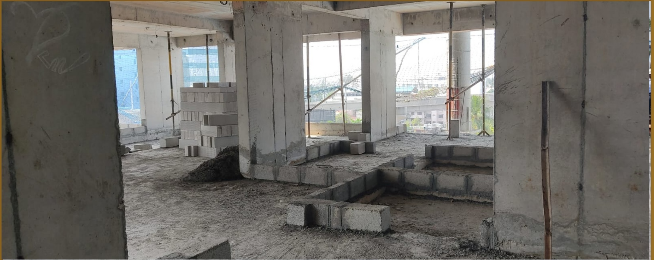
Block b -6th floor block work
