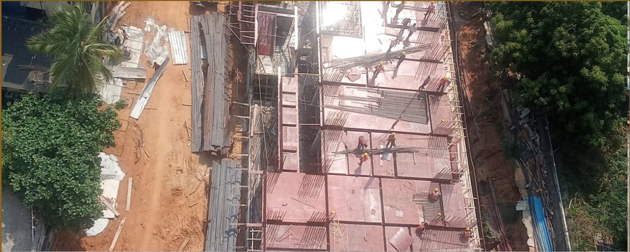
Block a - stilt roof slab shuttering work pour-1
