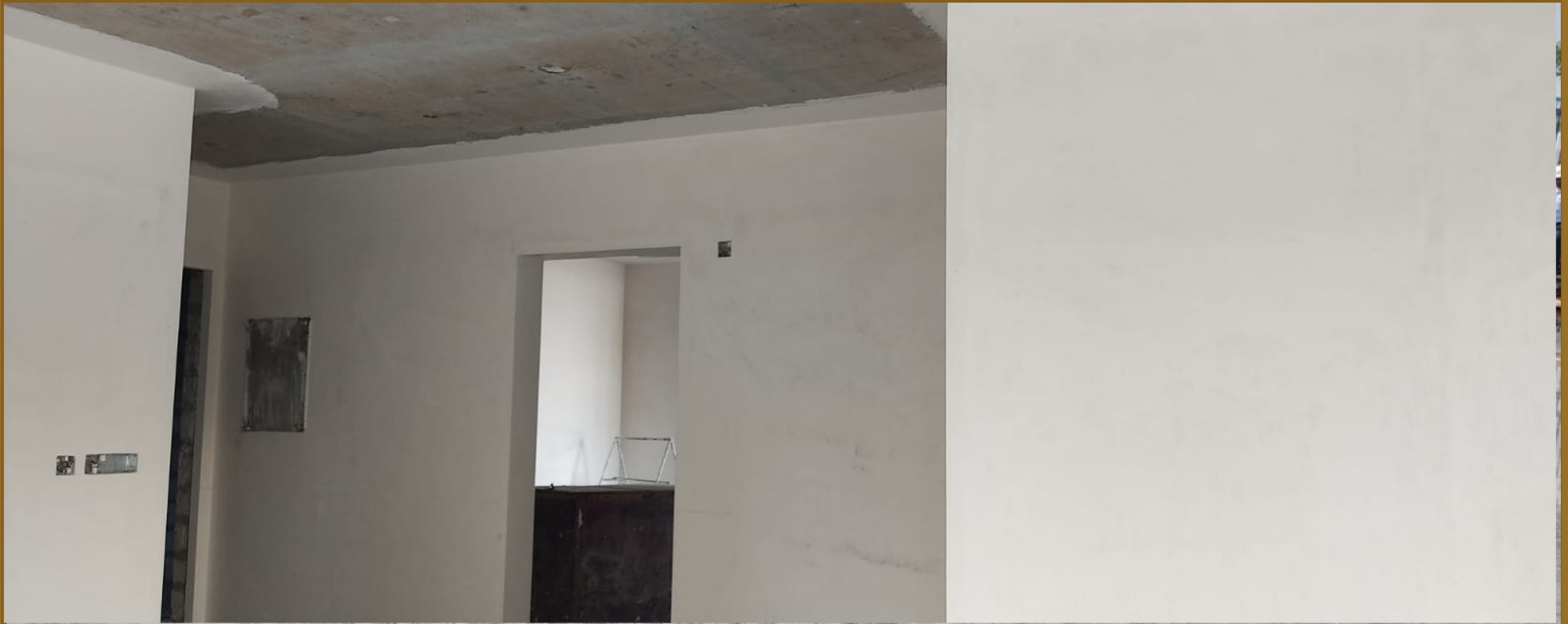
Block b -1st floor -flat No 8 Gypsum plaster work
