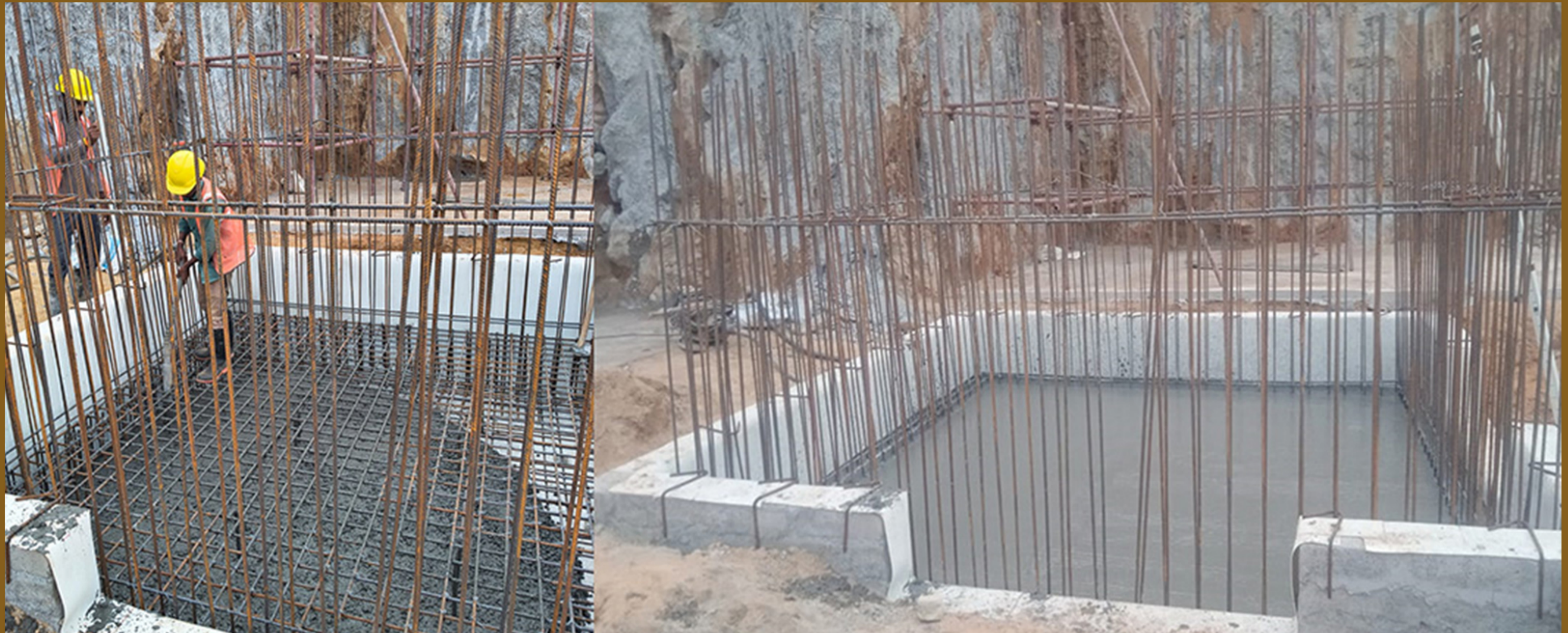
Block B collection pit raft concrete work
