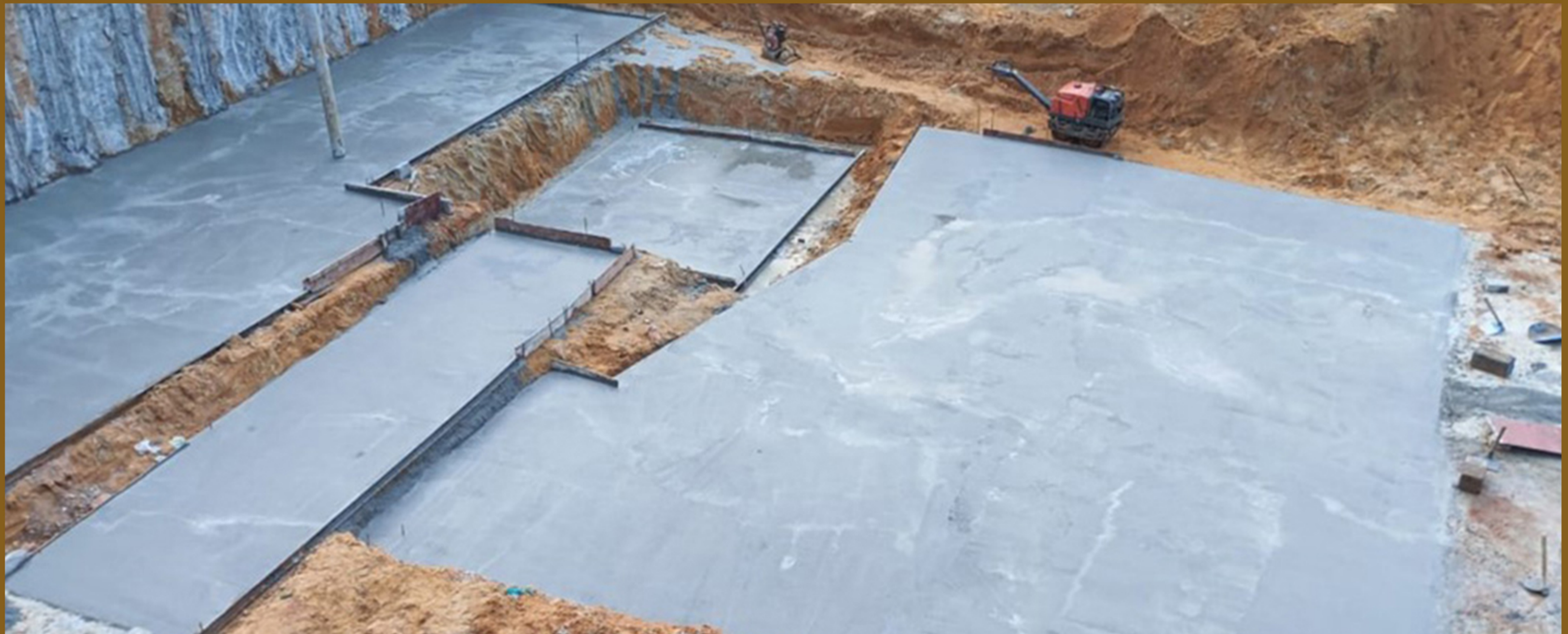
Block B Raft PCC laying
