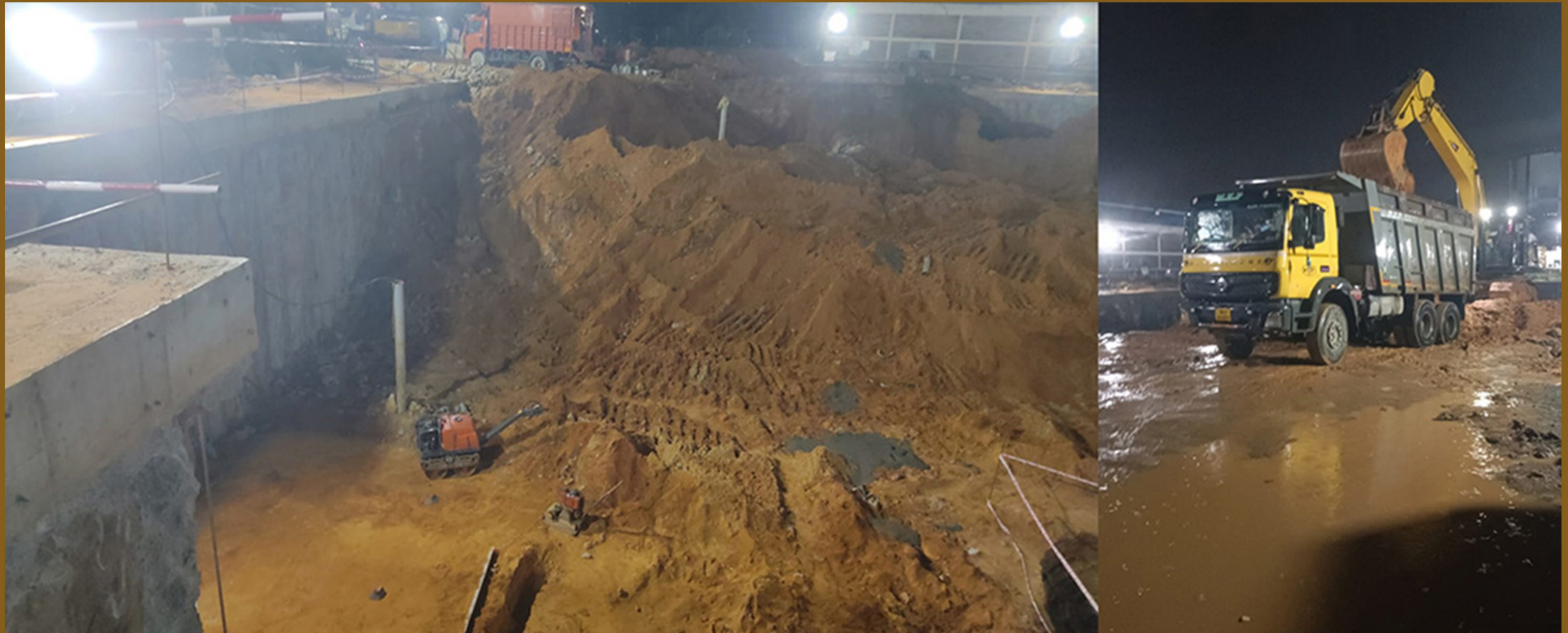
Block B earth excavation works
