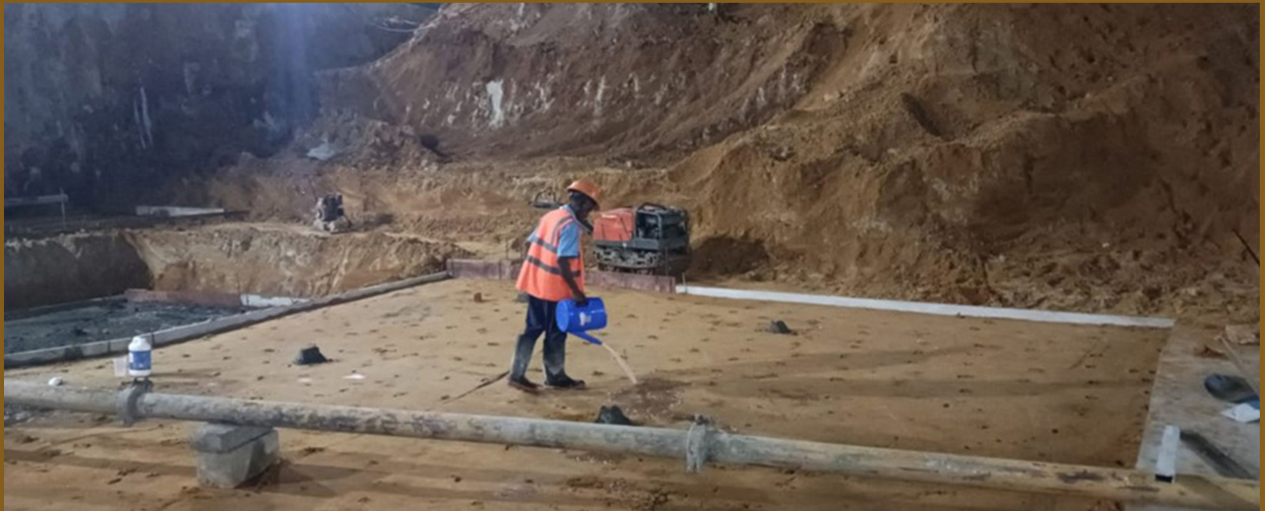
Block B Raft anti-termite work
