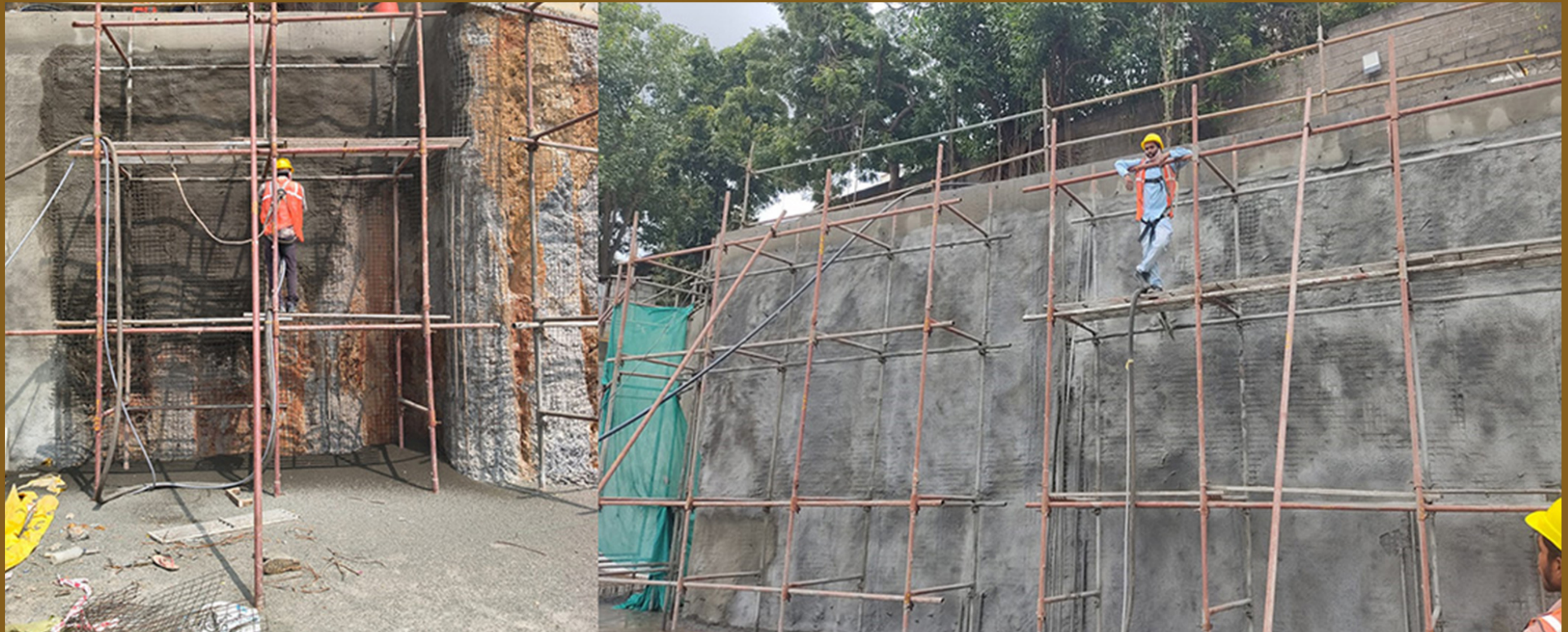
Block B shotcreting work
