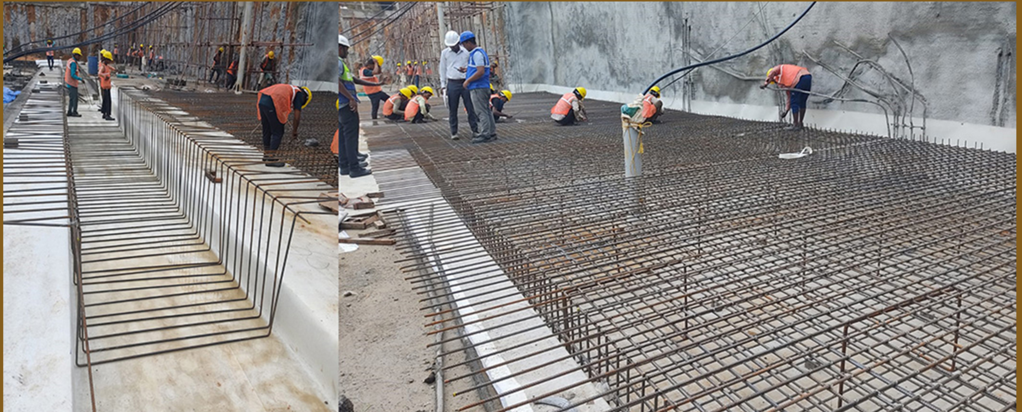
Block B raft reinforcement work
