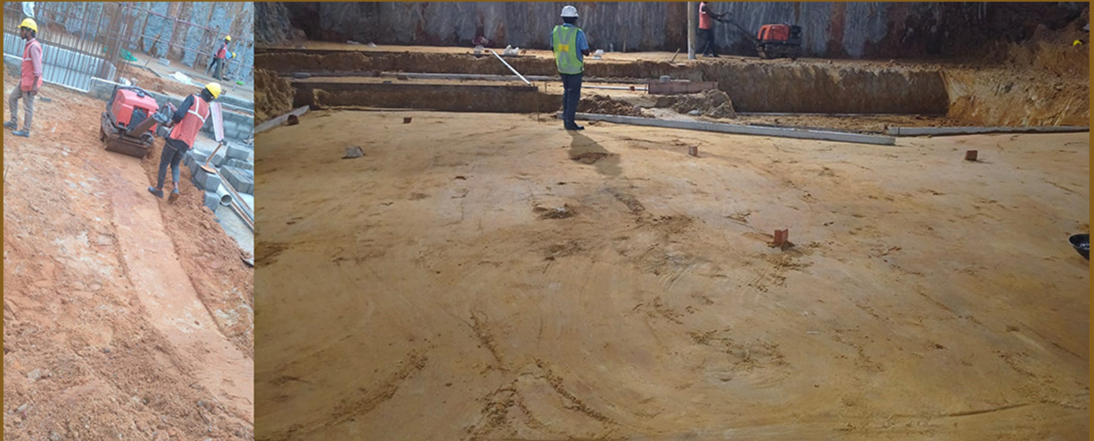
Block B earth excavation and dressing works
