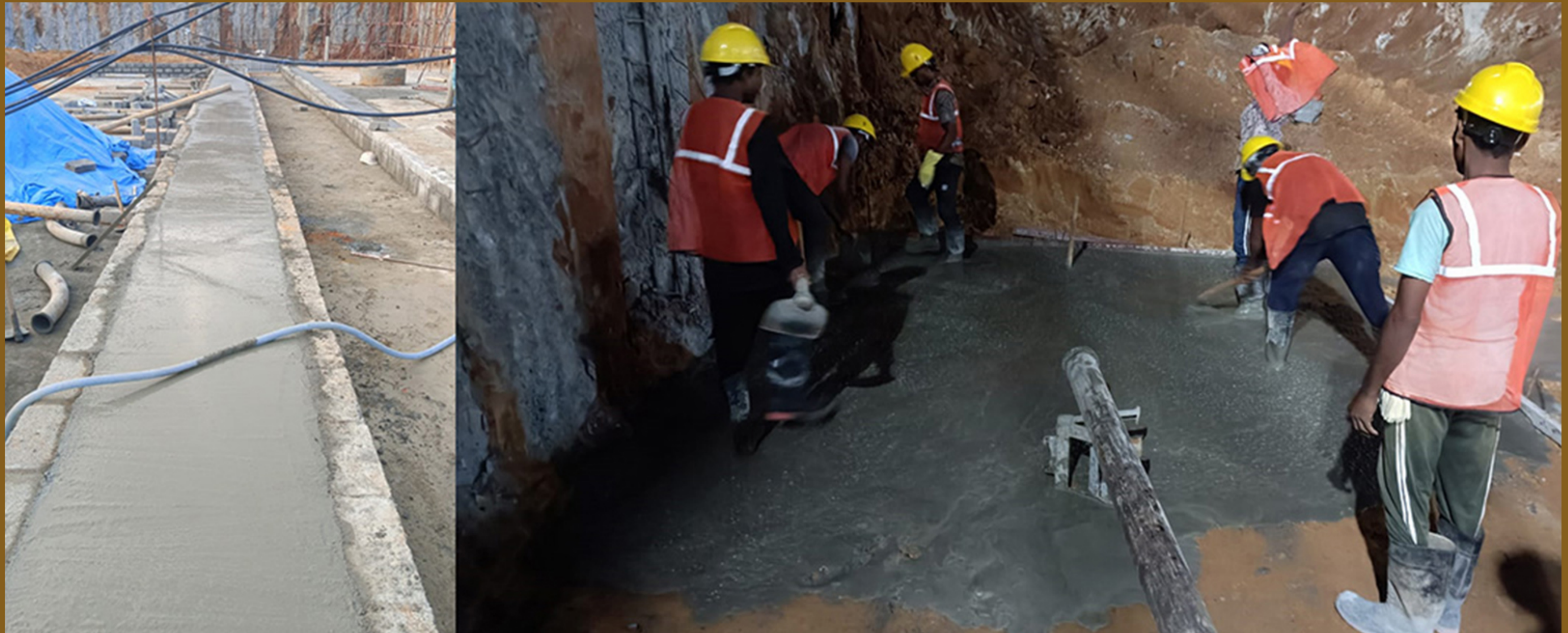
Block B Raft PCC laying
