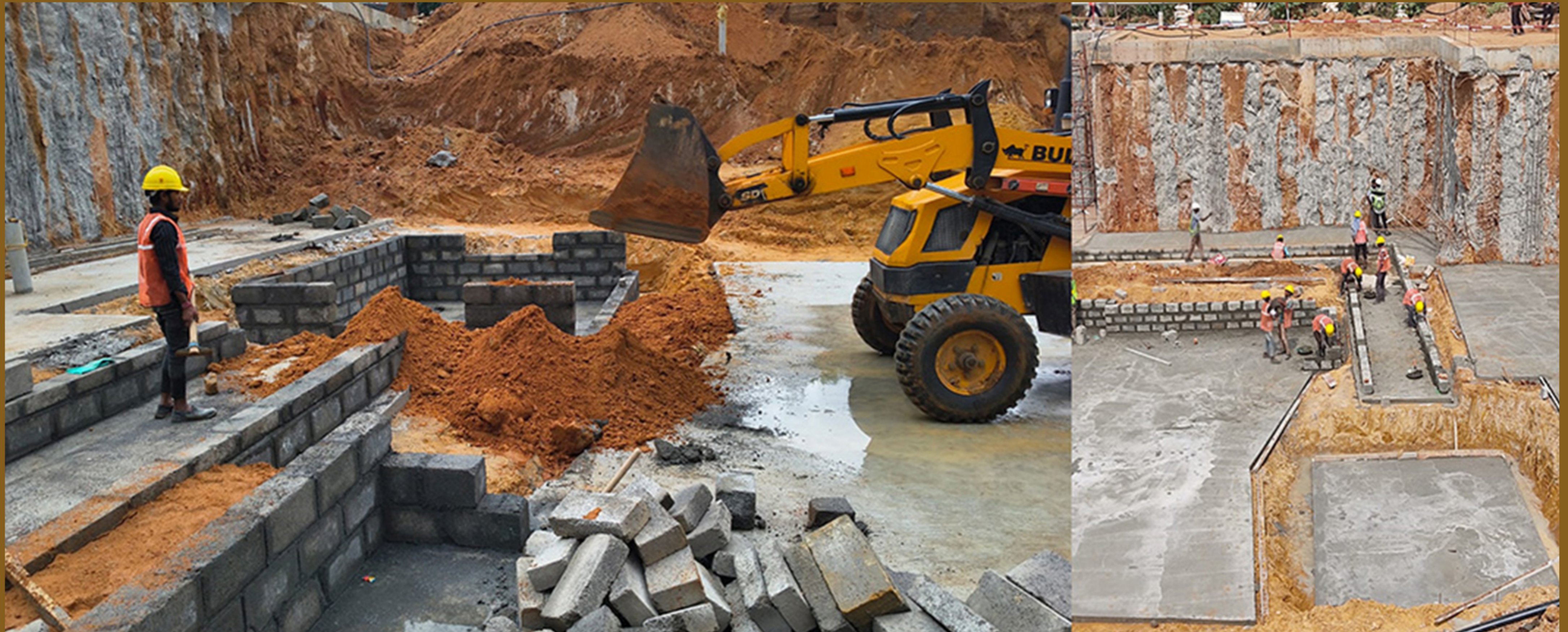
Block B trench block work
