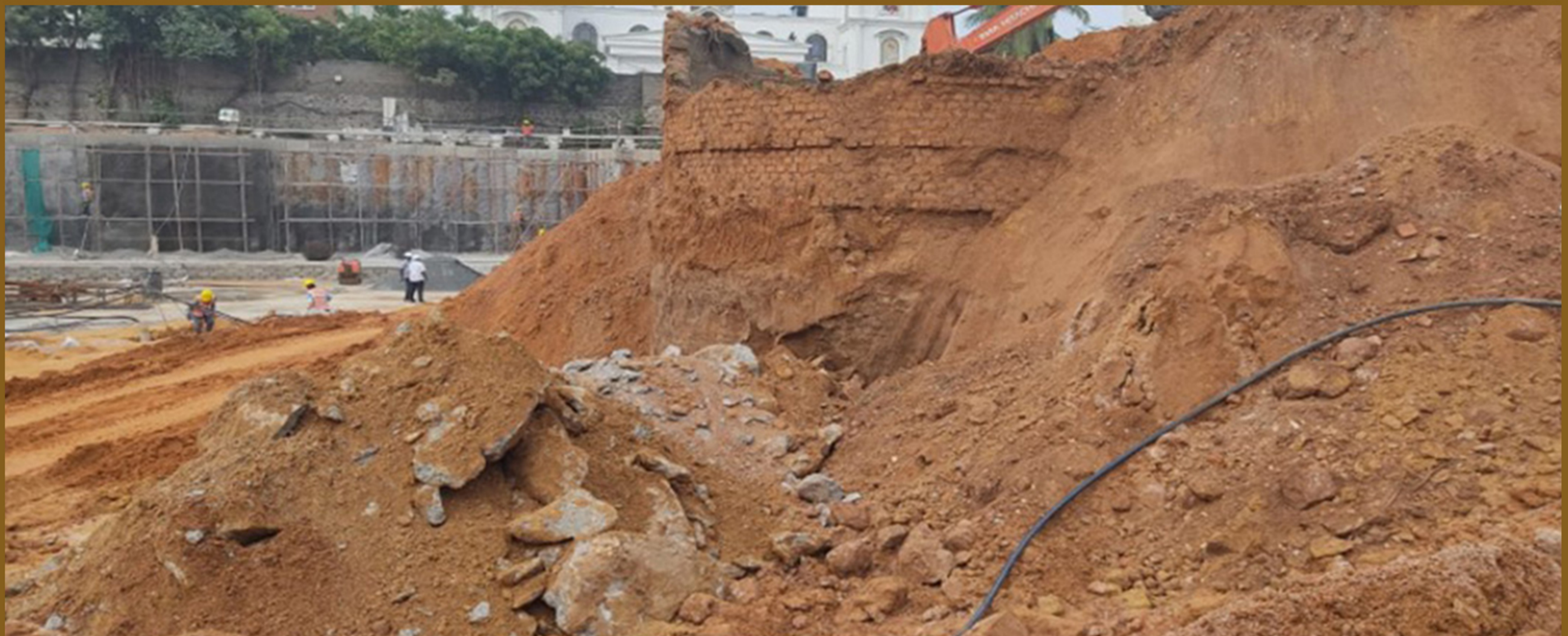
Block B earth excavation works
