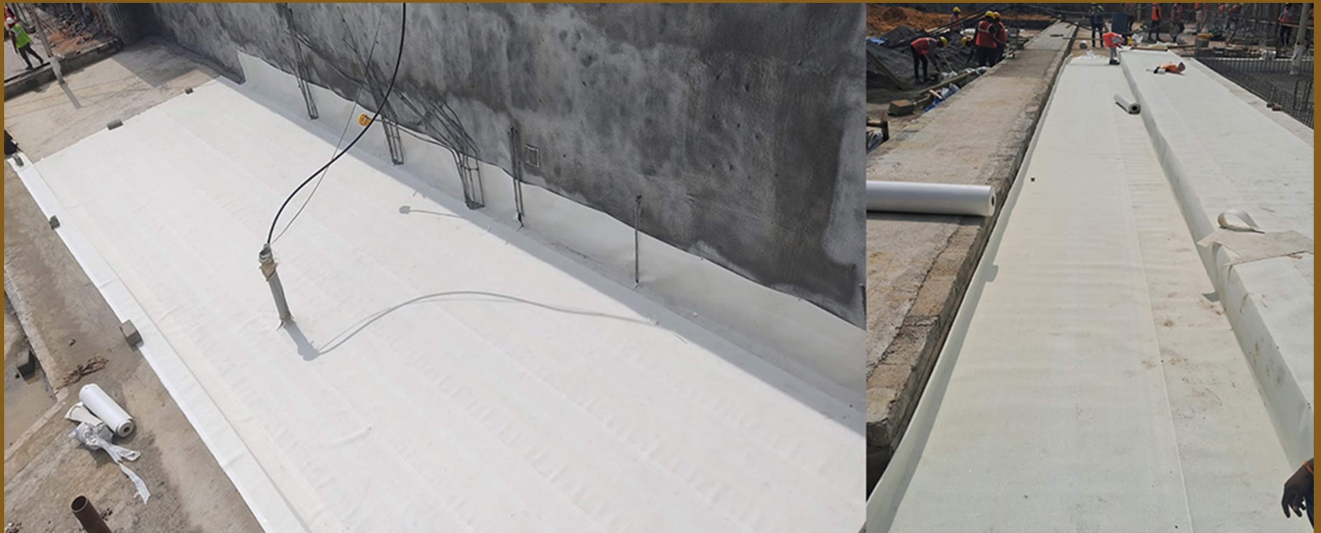
Block B raft water proofing work
