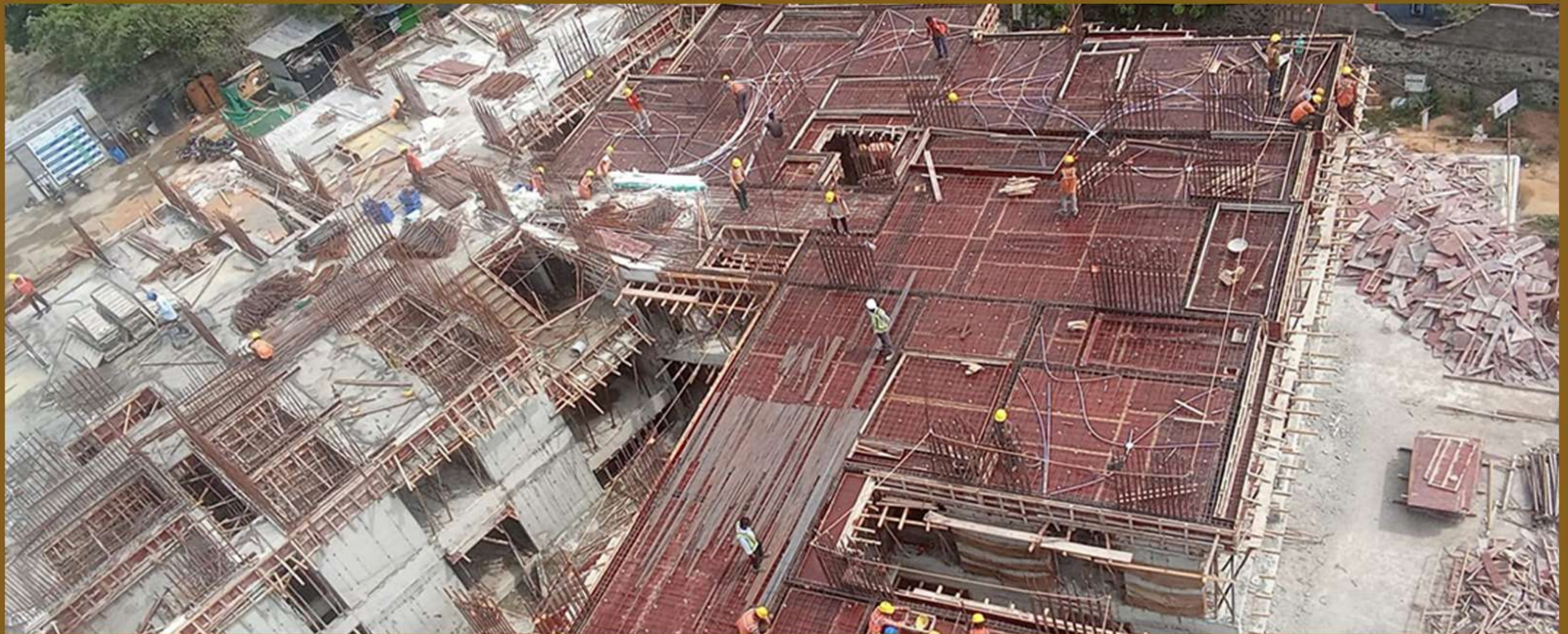
Block B – 2nd Floor Roof Shuttering Work
