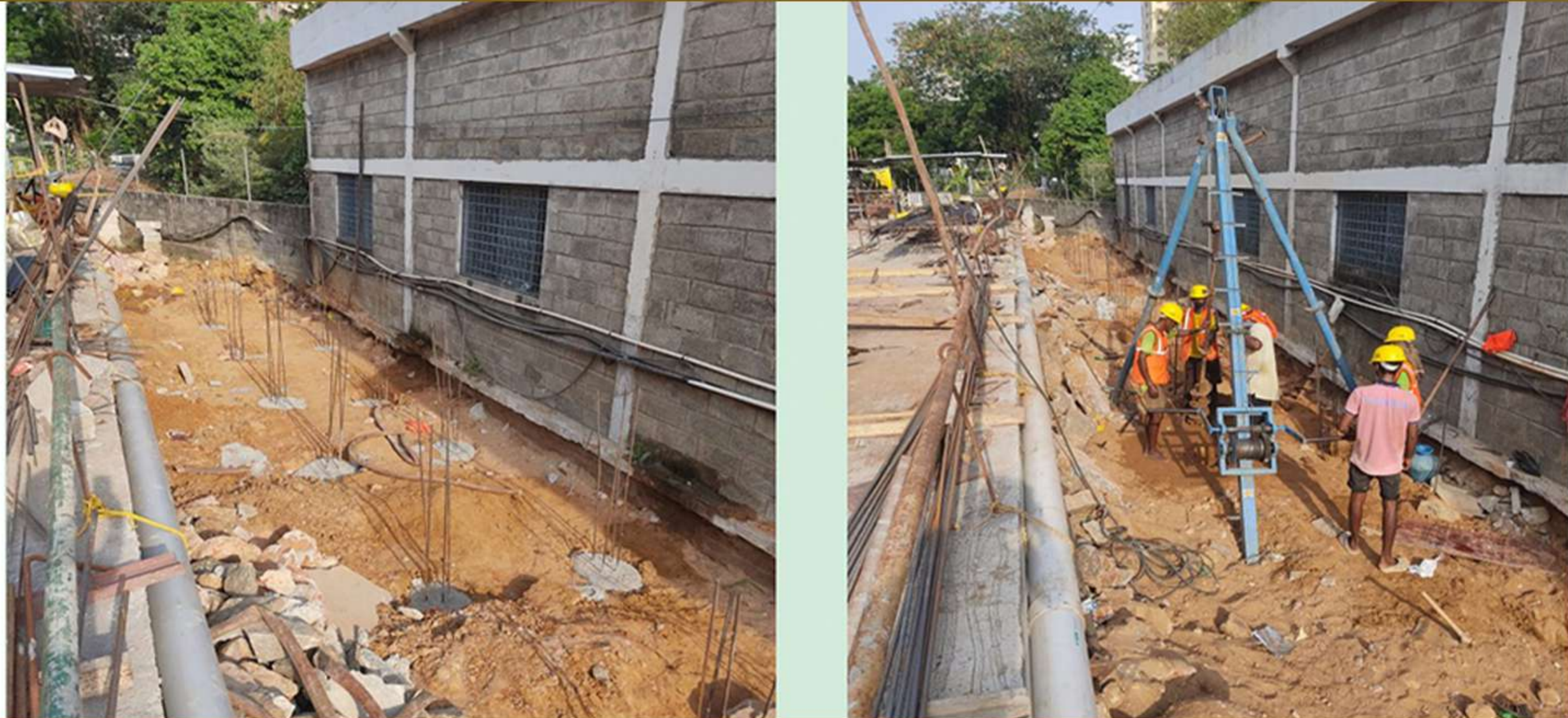
Block A – South Side Compound Wall Pile Work
