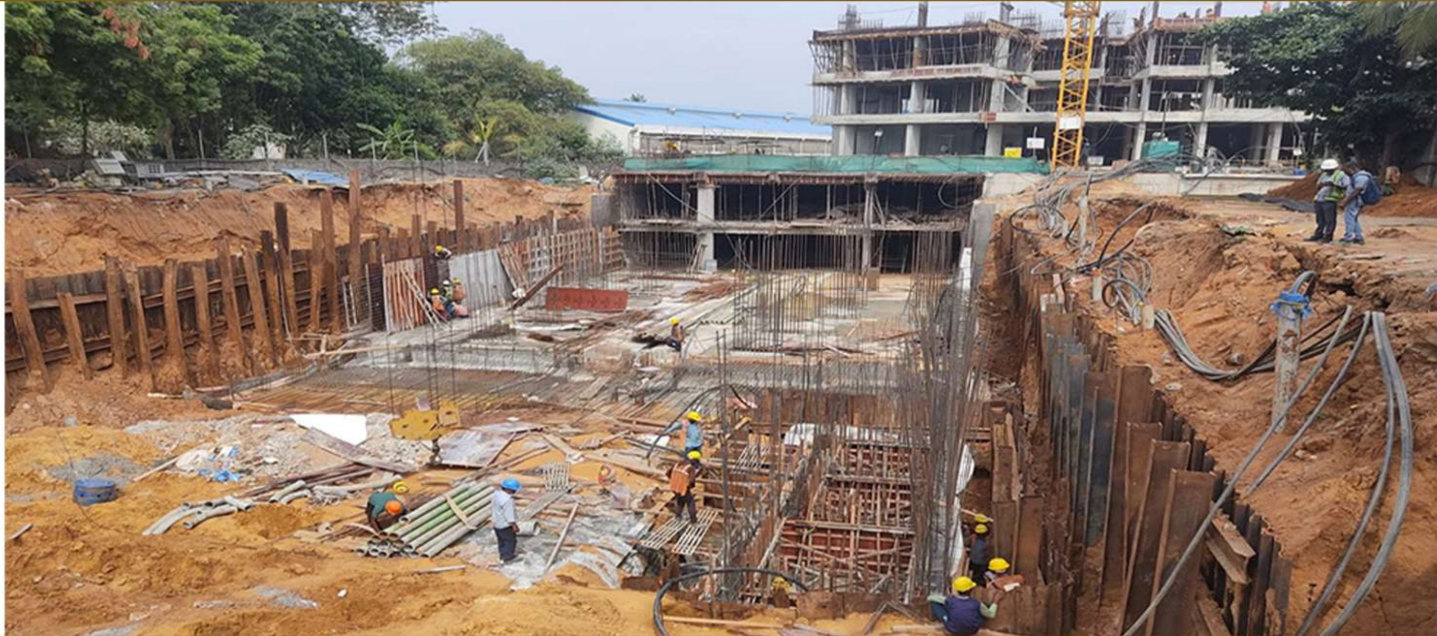
Block A – Lift Raft Rcc Laying
