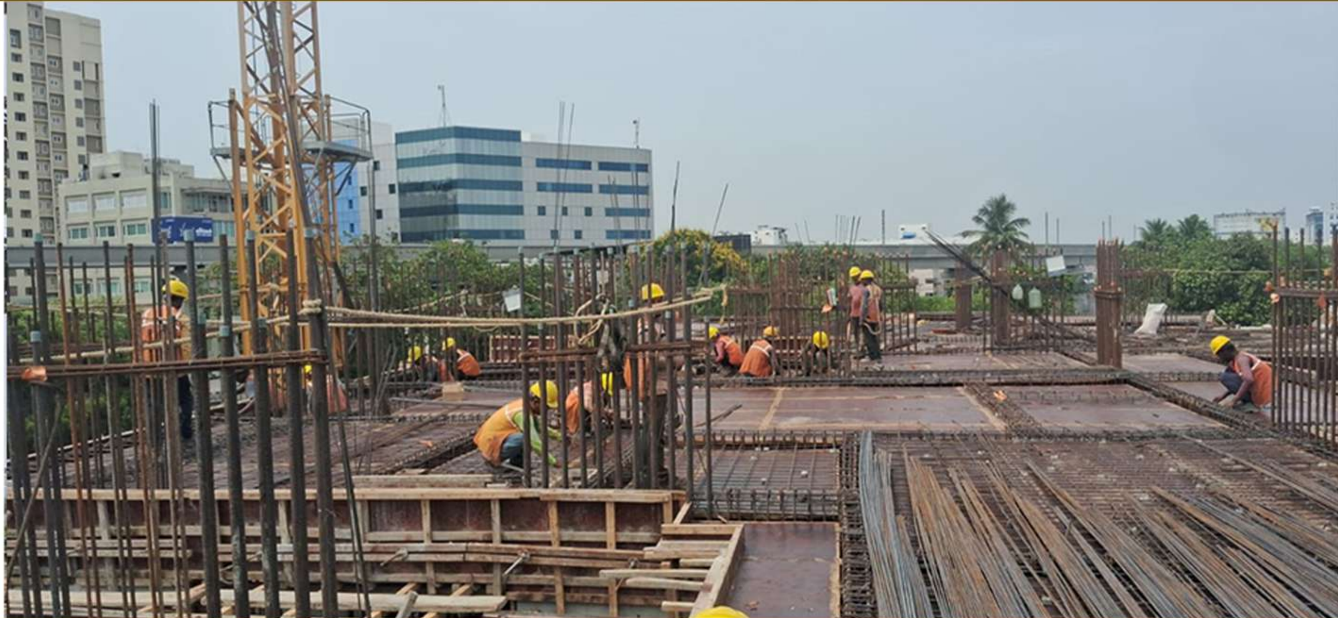
Block B – 2nd Floor Roof Reinforcement Work
