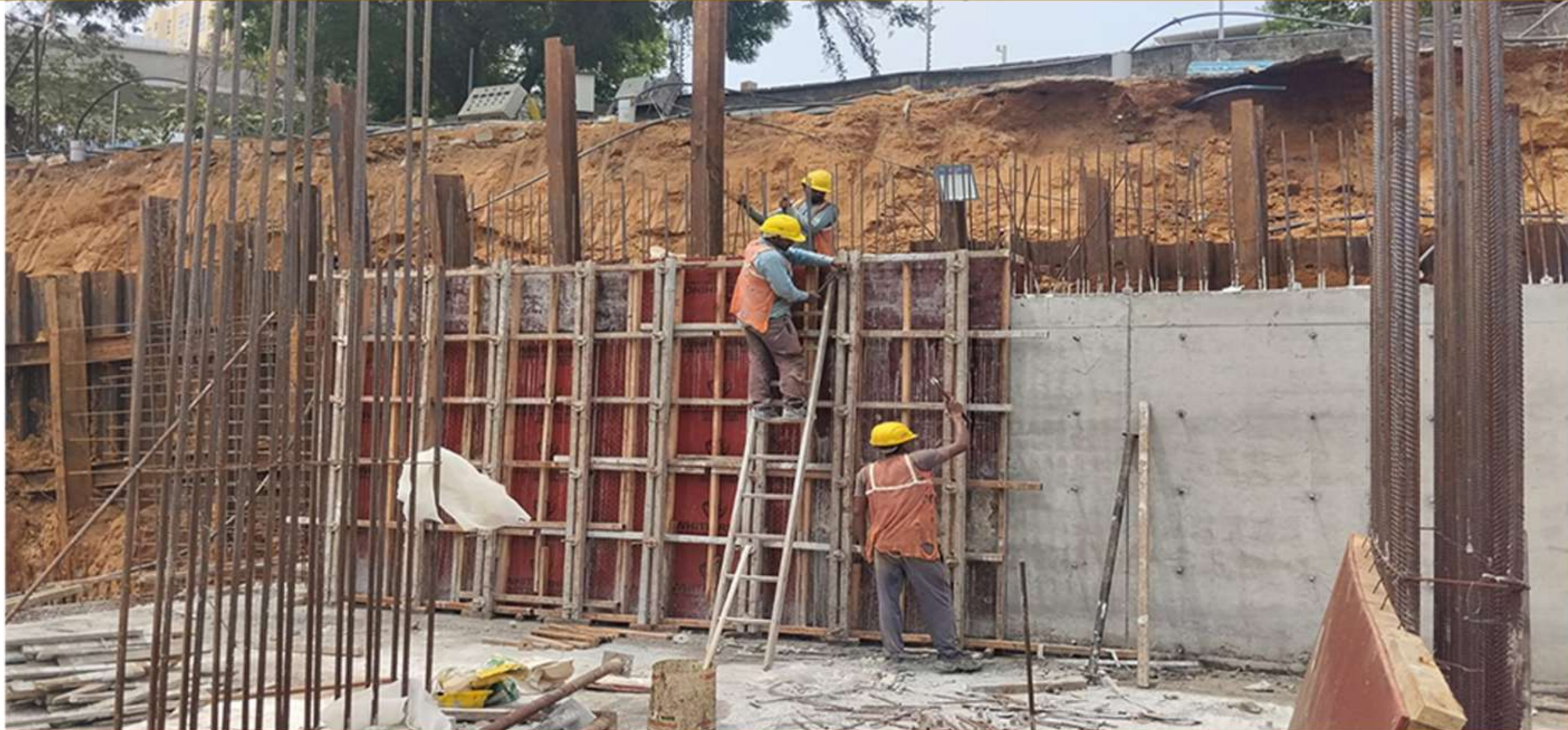
Block A – Retaining Wall Shuttering Work
