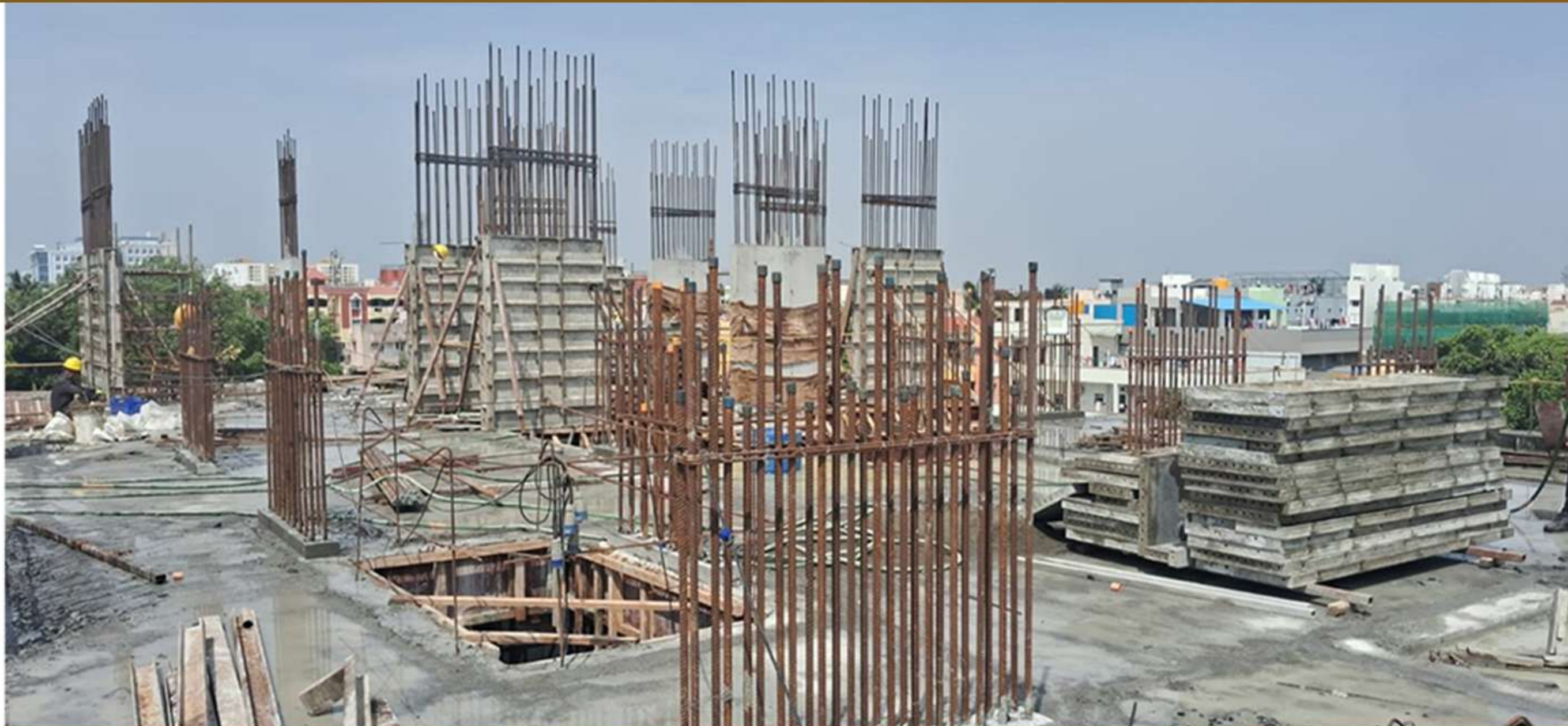
Block b – 3rd Floor Column Concrete Work
