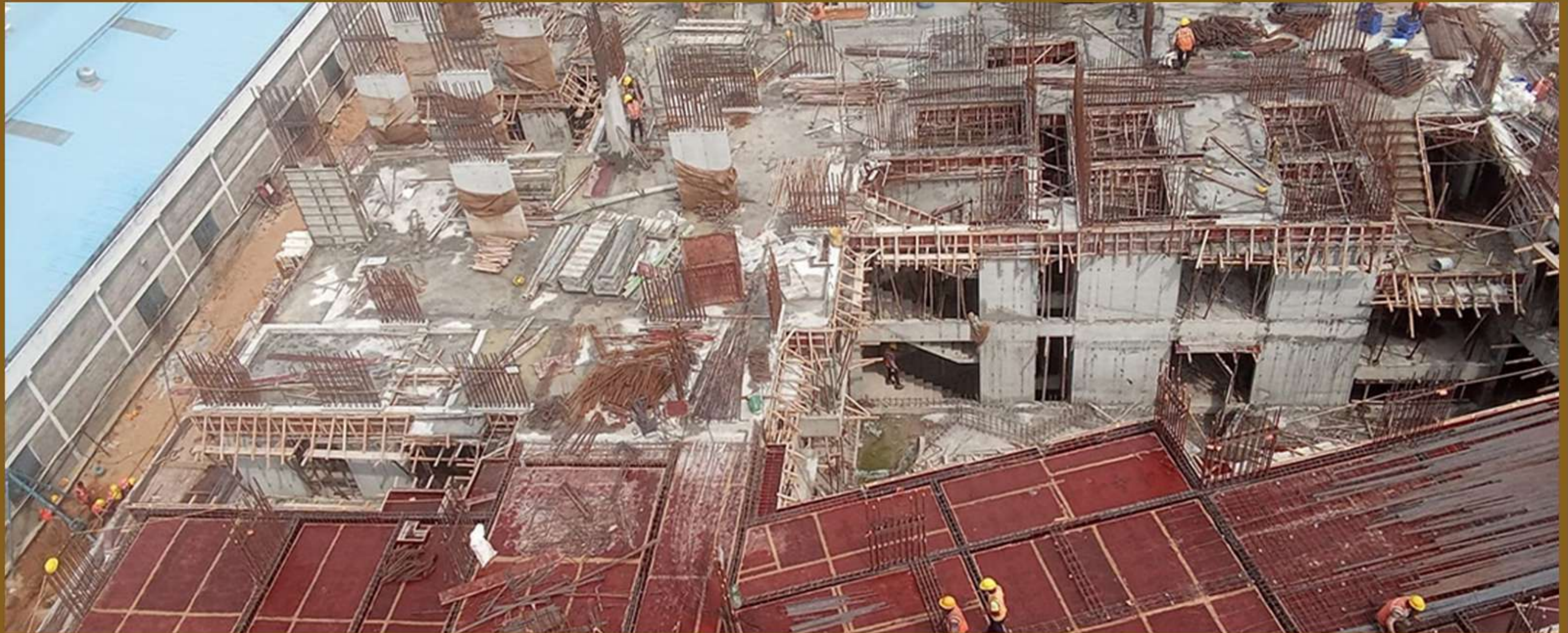
Block B – 2nd Floor Roof Reinforcement Work
