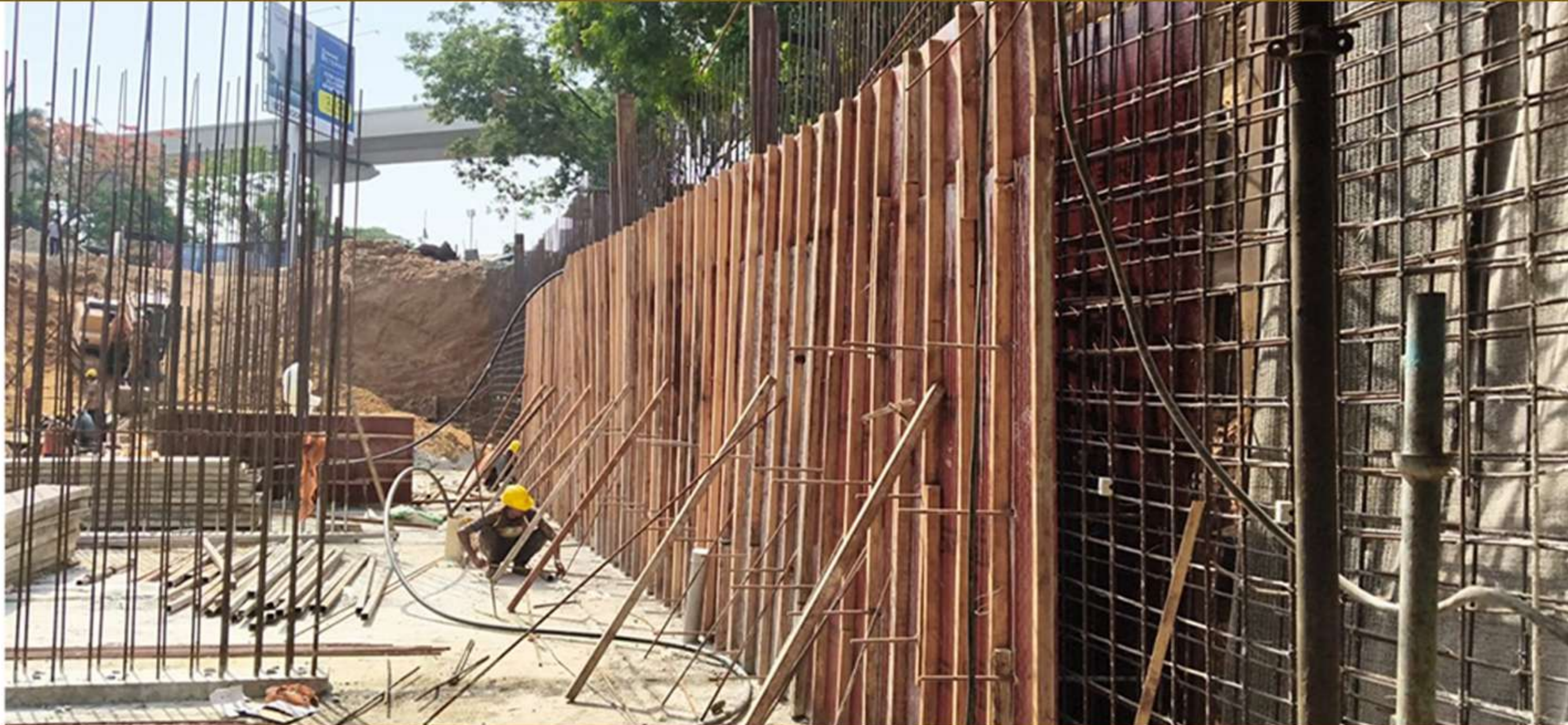
Block A – Retaining Wall Shuttering Work
