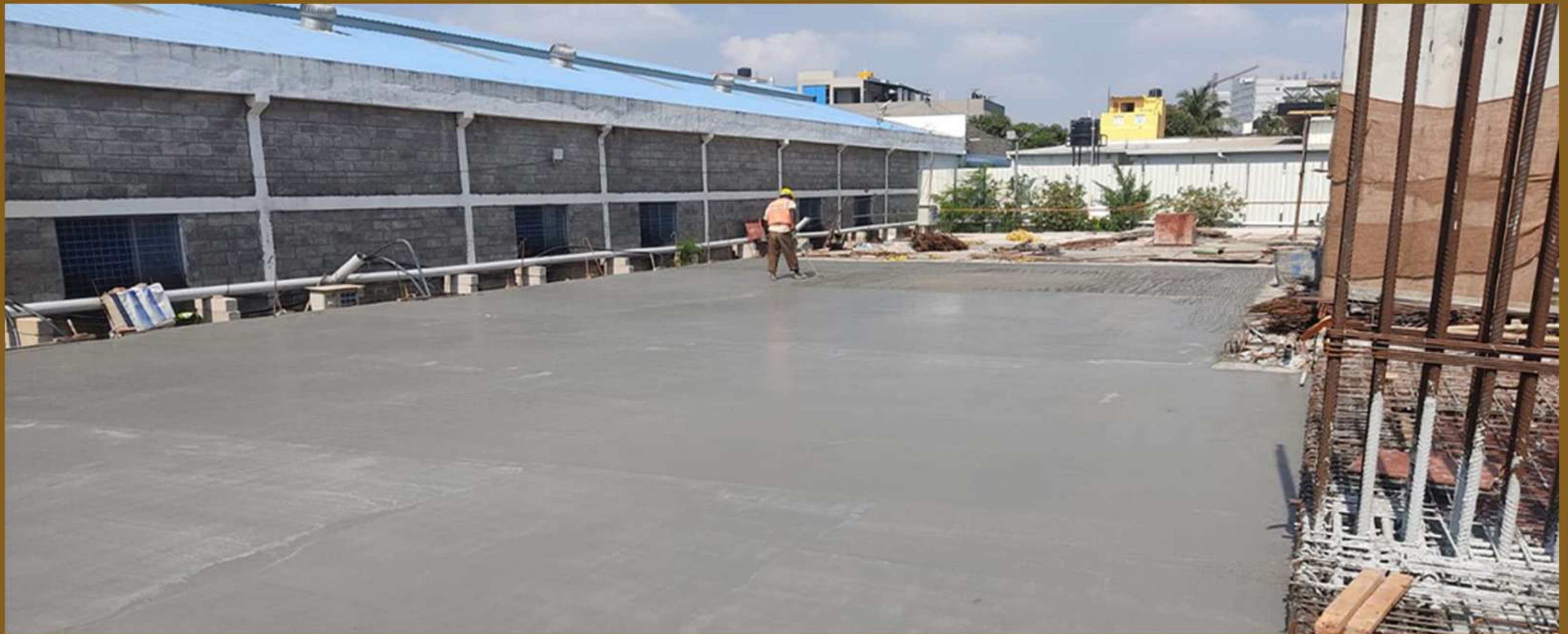
Block B Basement-1 Roof Concrete Work
