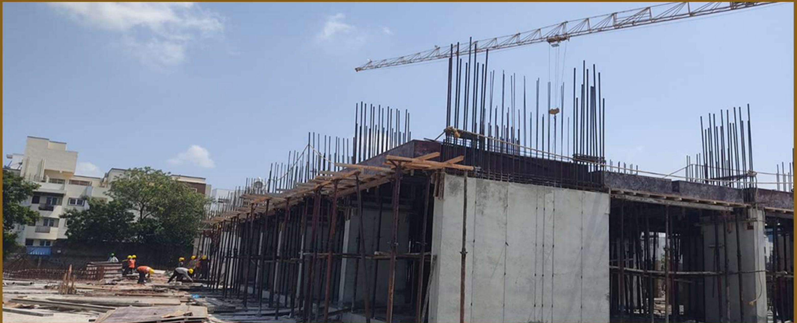
Block-B Stilt Roof Slab Shuttering Work
