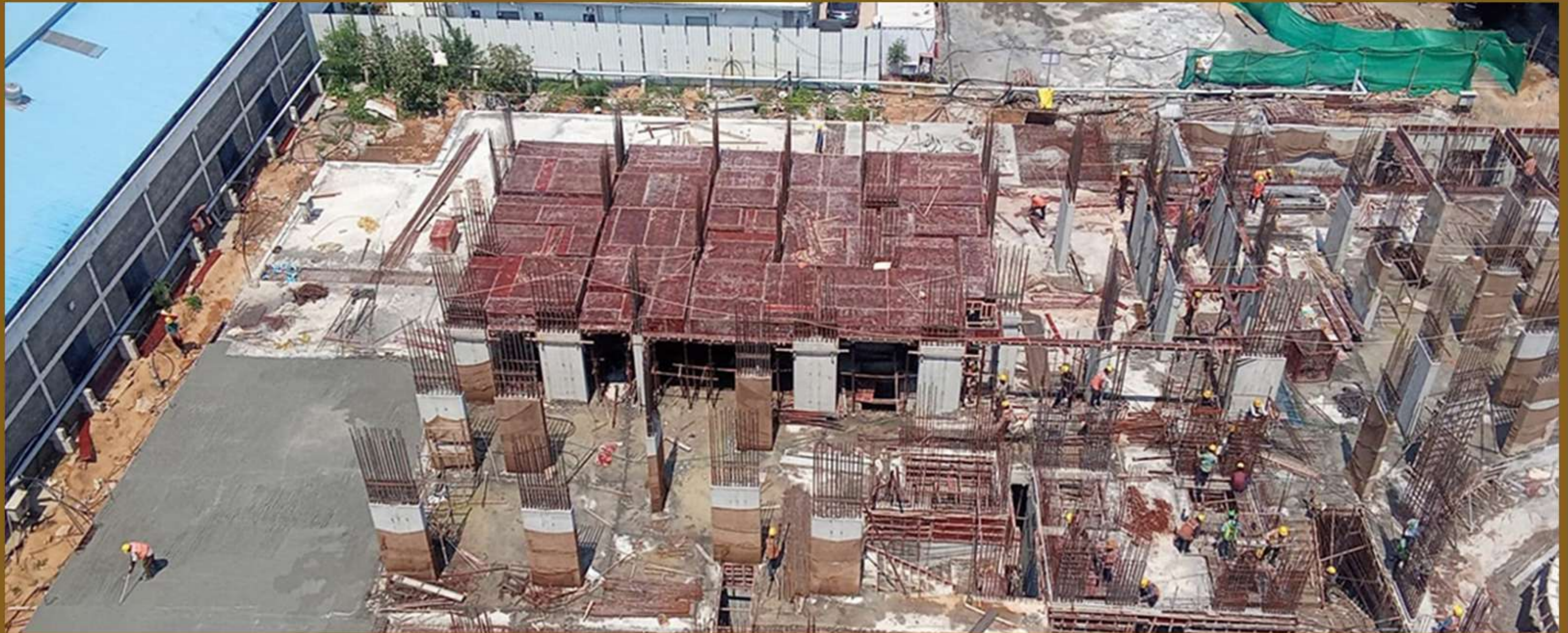
Block-B Stilt Roof Slab Shuttering Work
