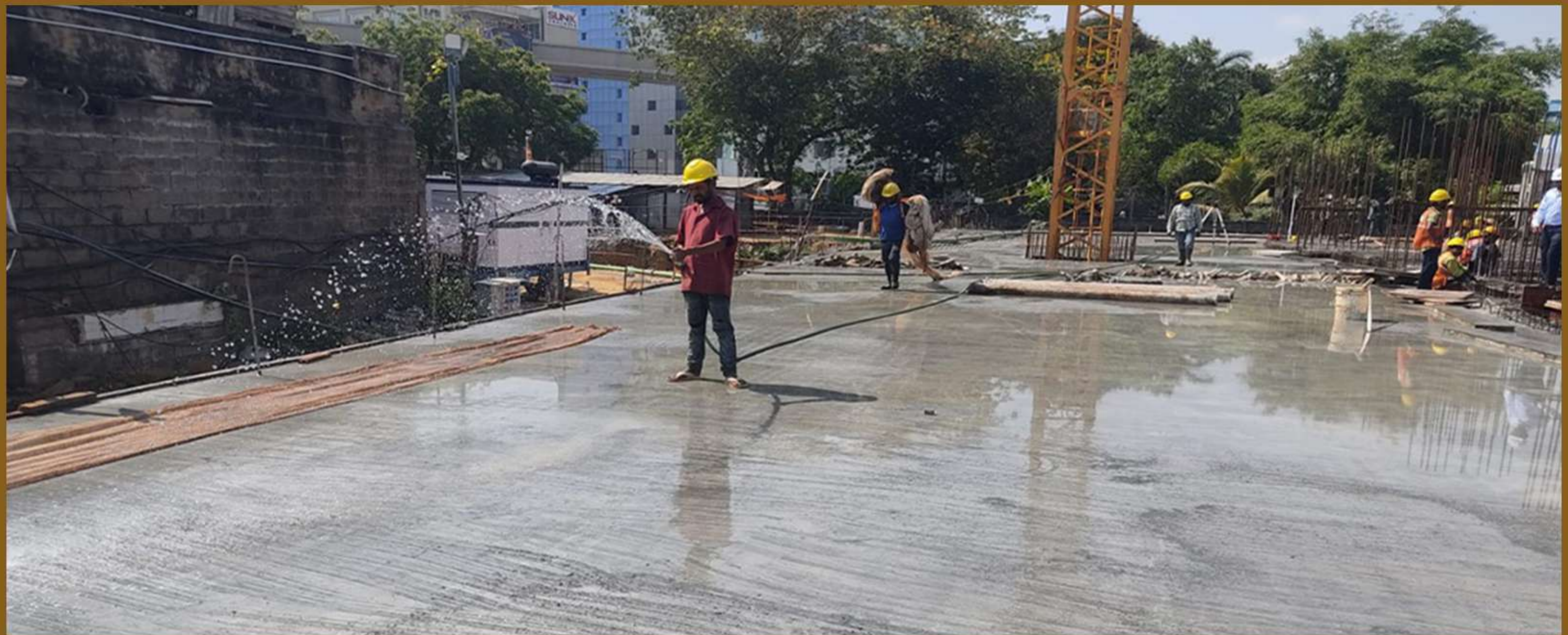
Block B - Curing Works
