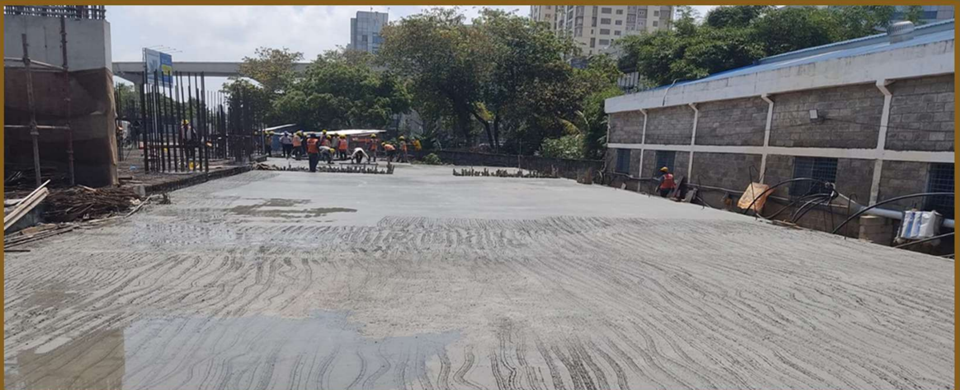
Block B Basement-1 Roof Concrete Work
