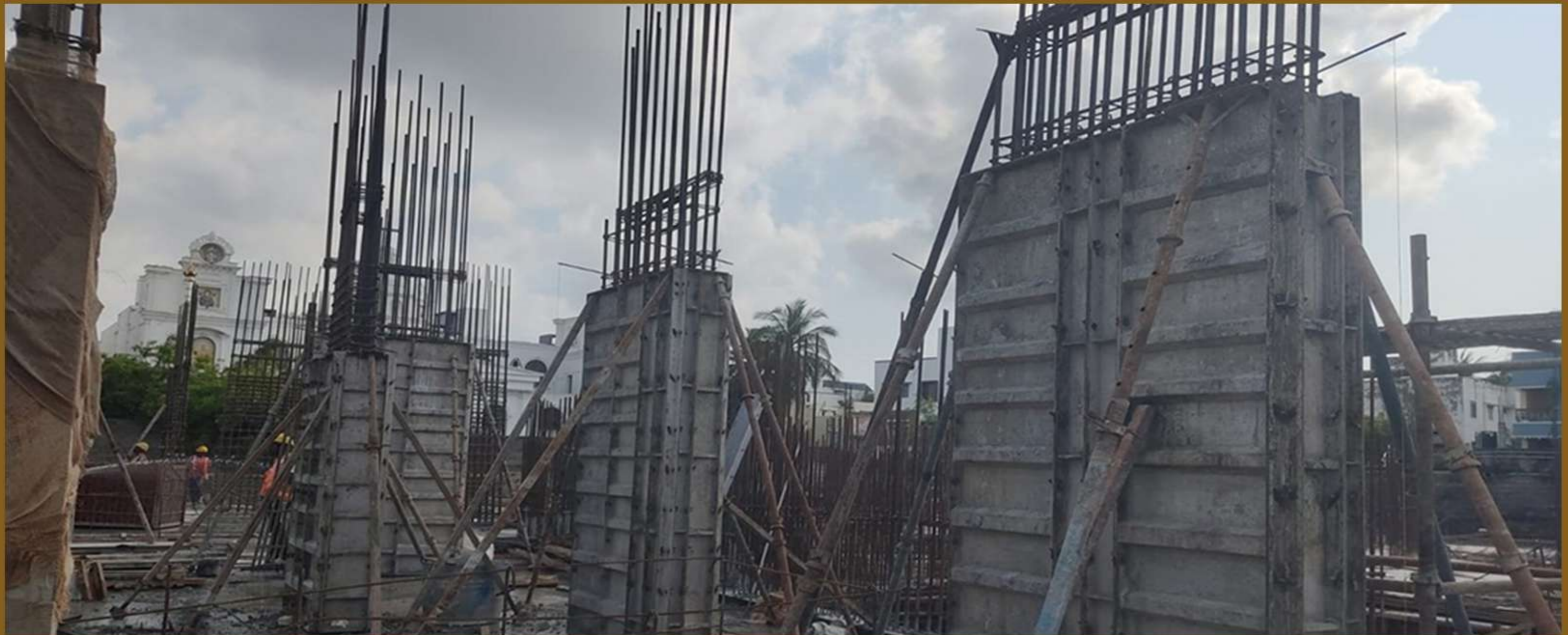
Block B Column Shuttering Work In Stilt Floor
