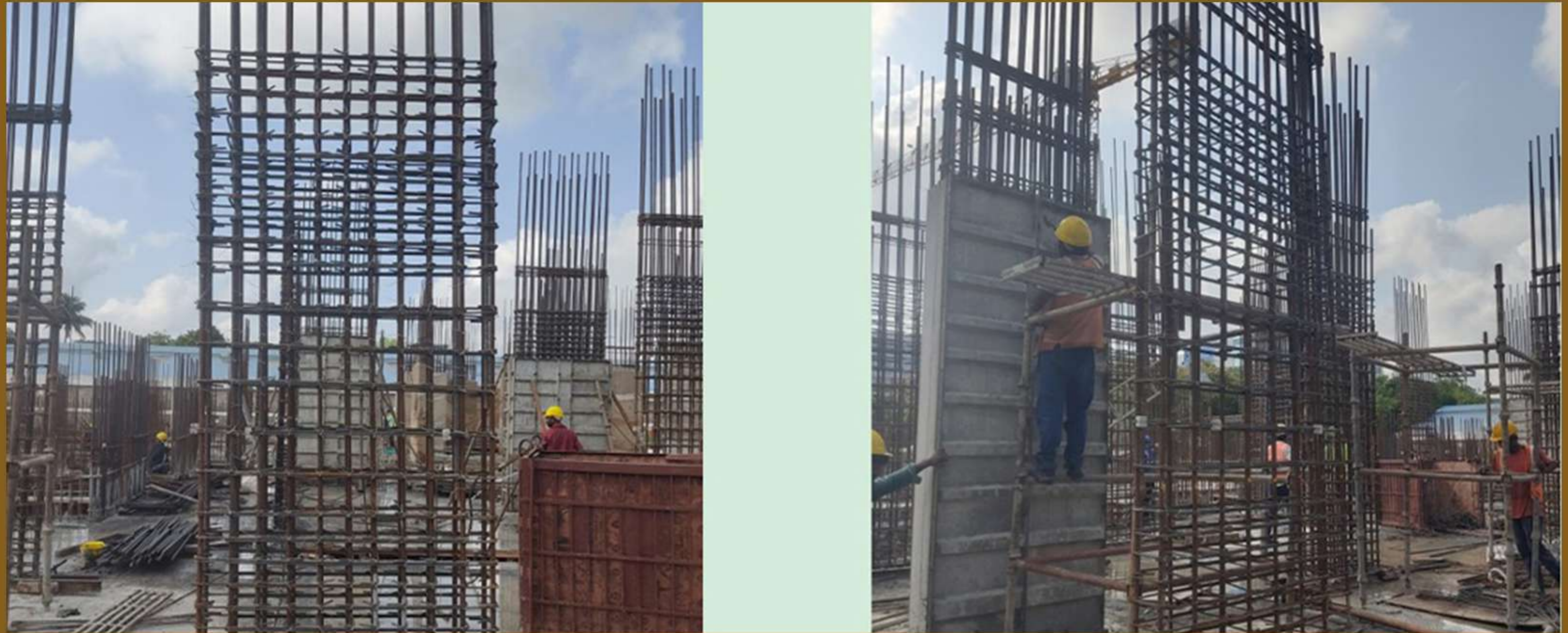
Block B Column Reinforcement Work In Stilt Floor
