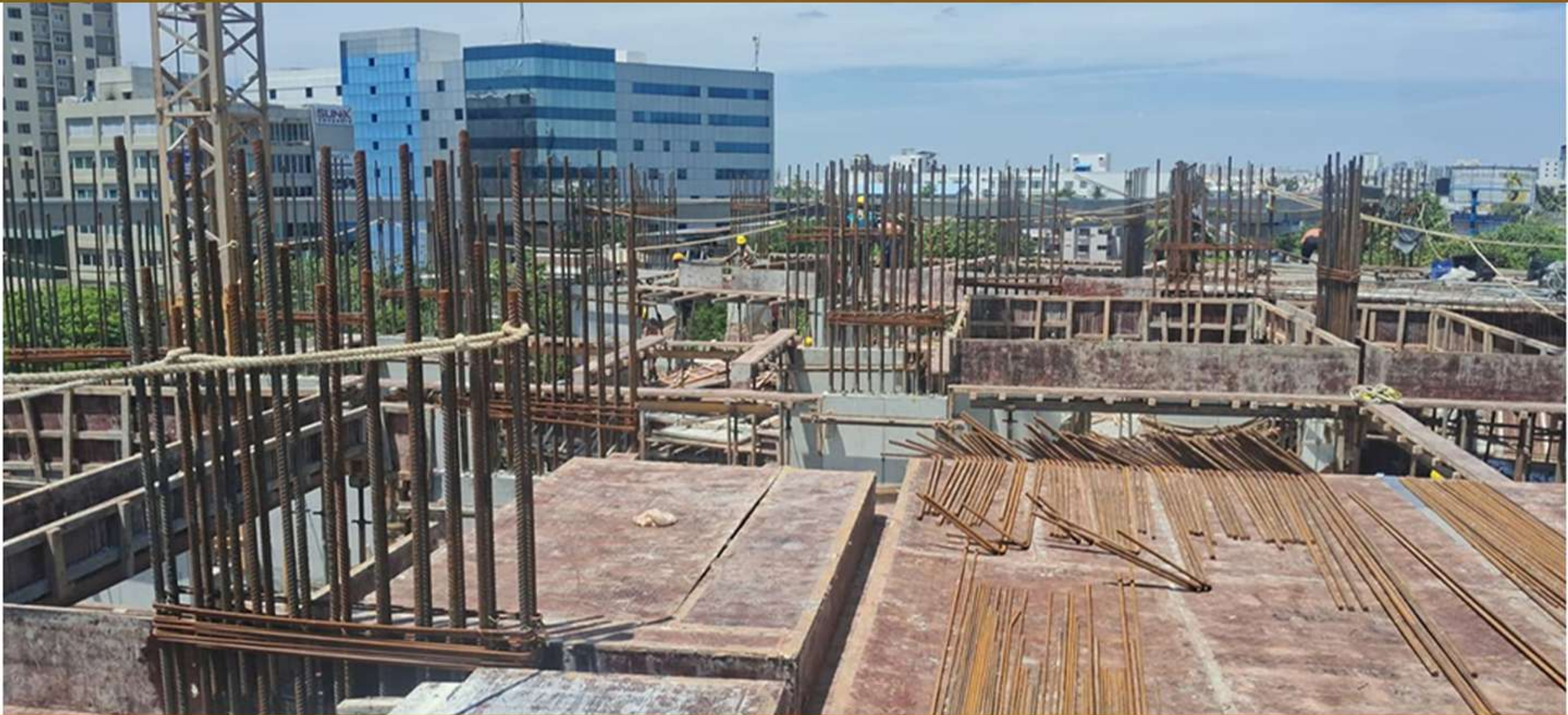
Block B – 4th Floor Roof Shuttering Work
