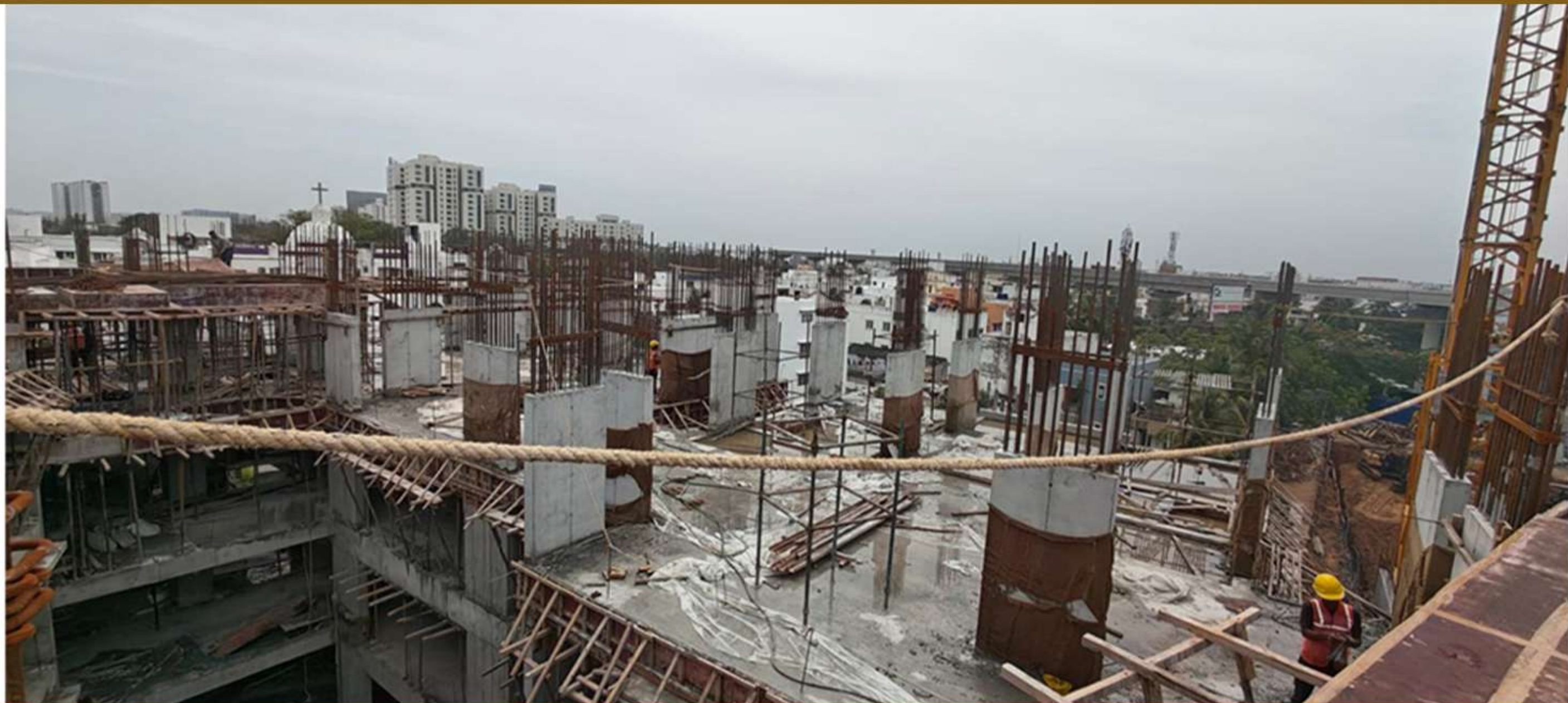
Block B – 4th Floor column concrete work
