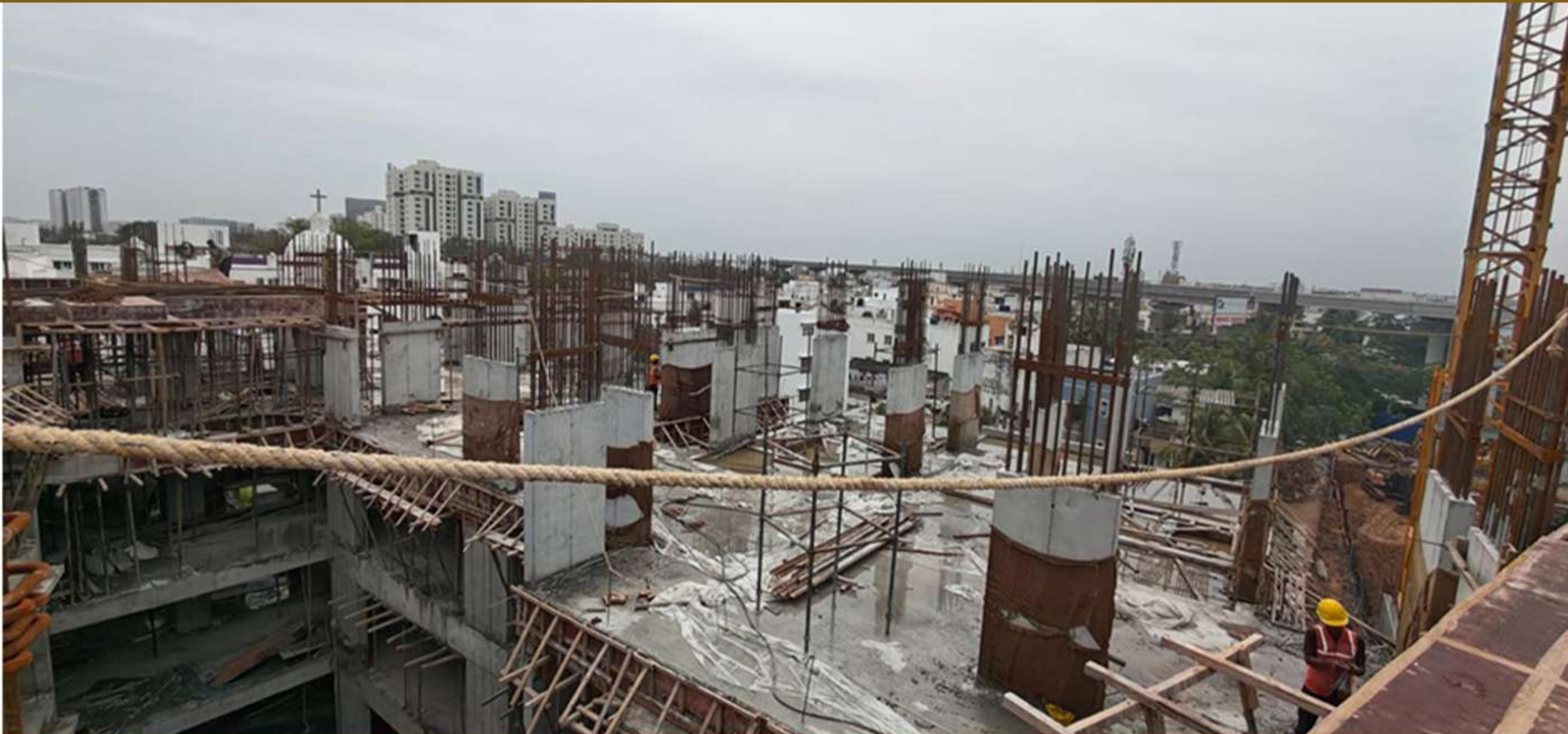
Block B – 4th Floor Column Shuttering Work
