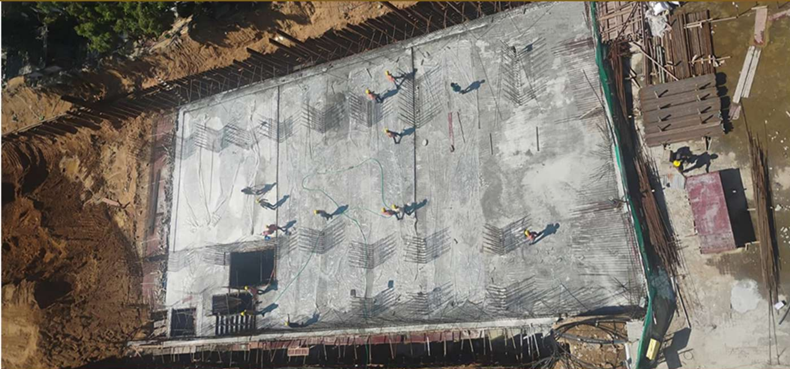
Block A – Lower basement roof slab concrete (pour-1)
