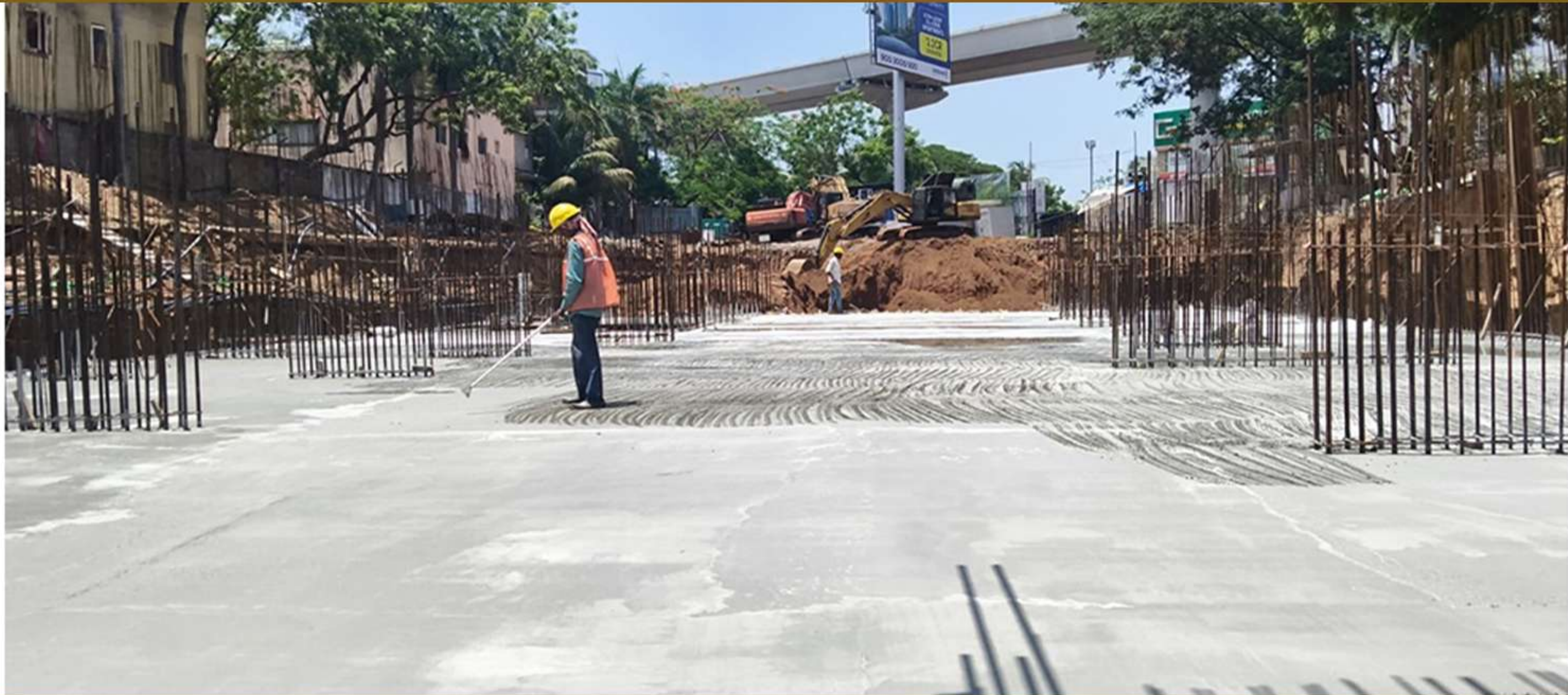
Block A – Lower basement roof concrete (pour-1)
