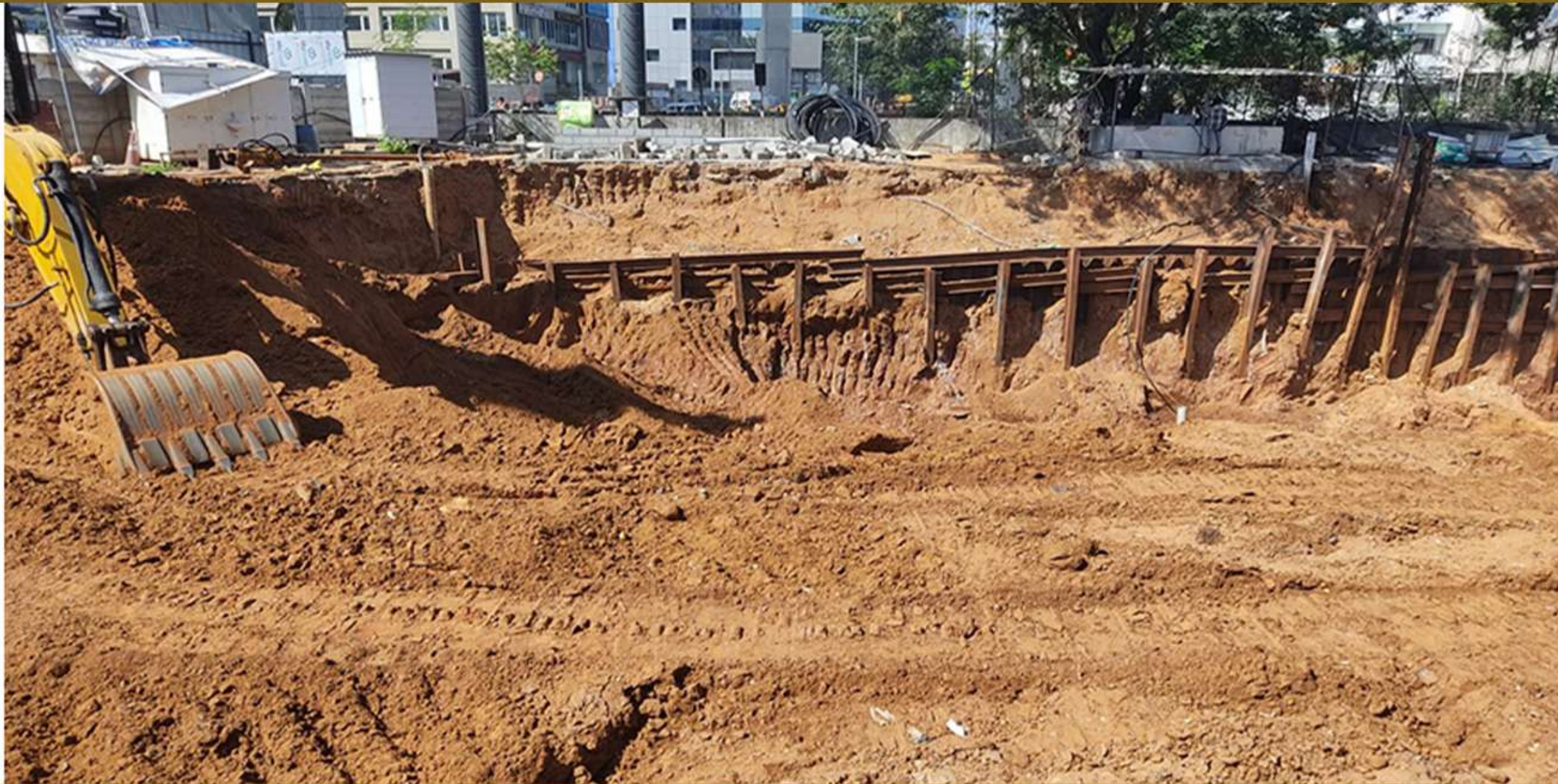
Block A – Earth work excavation (pour-2)
