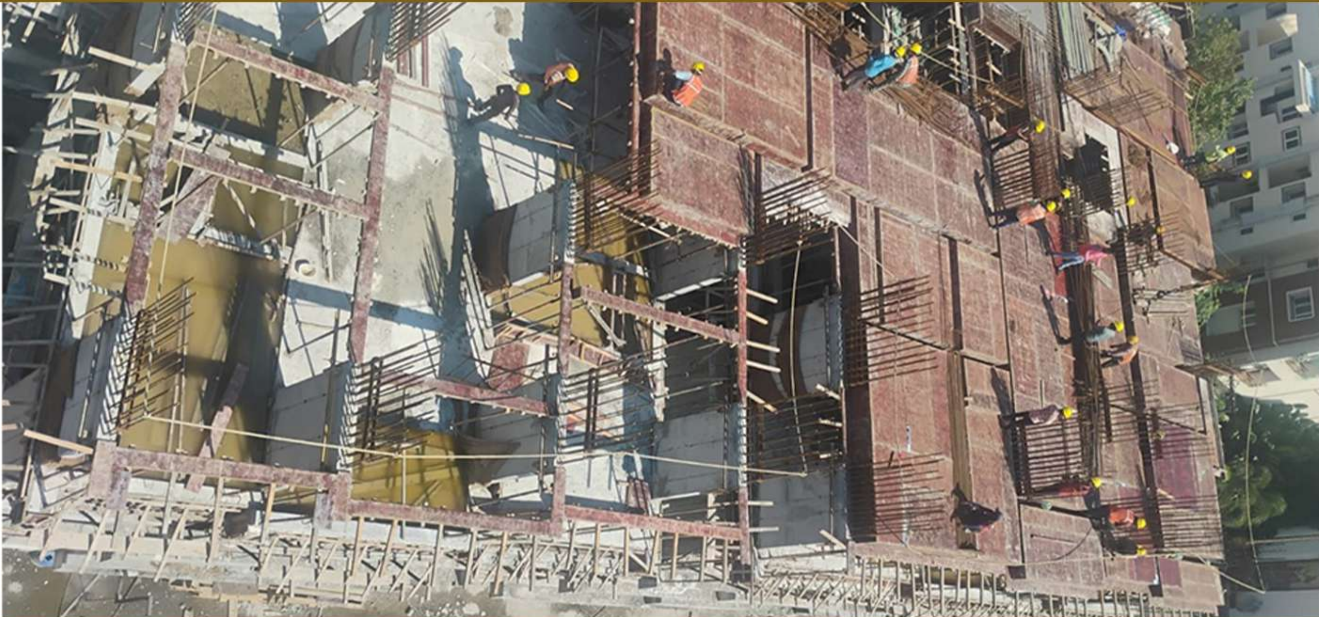
Block B – 4th Floor Roof Shuttering Work
