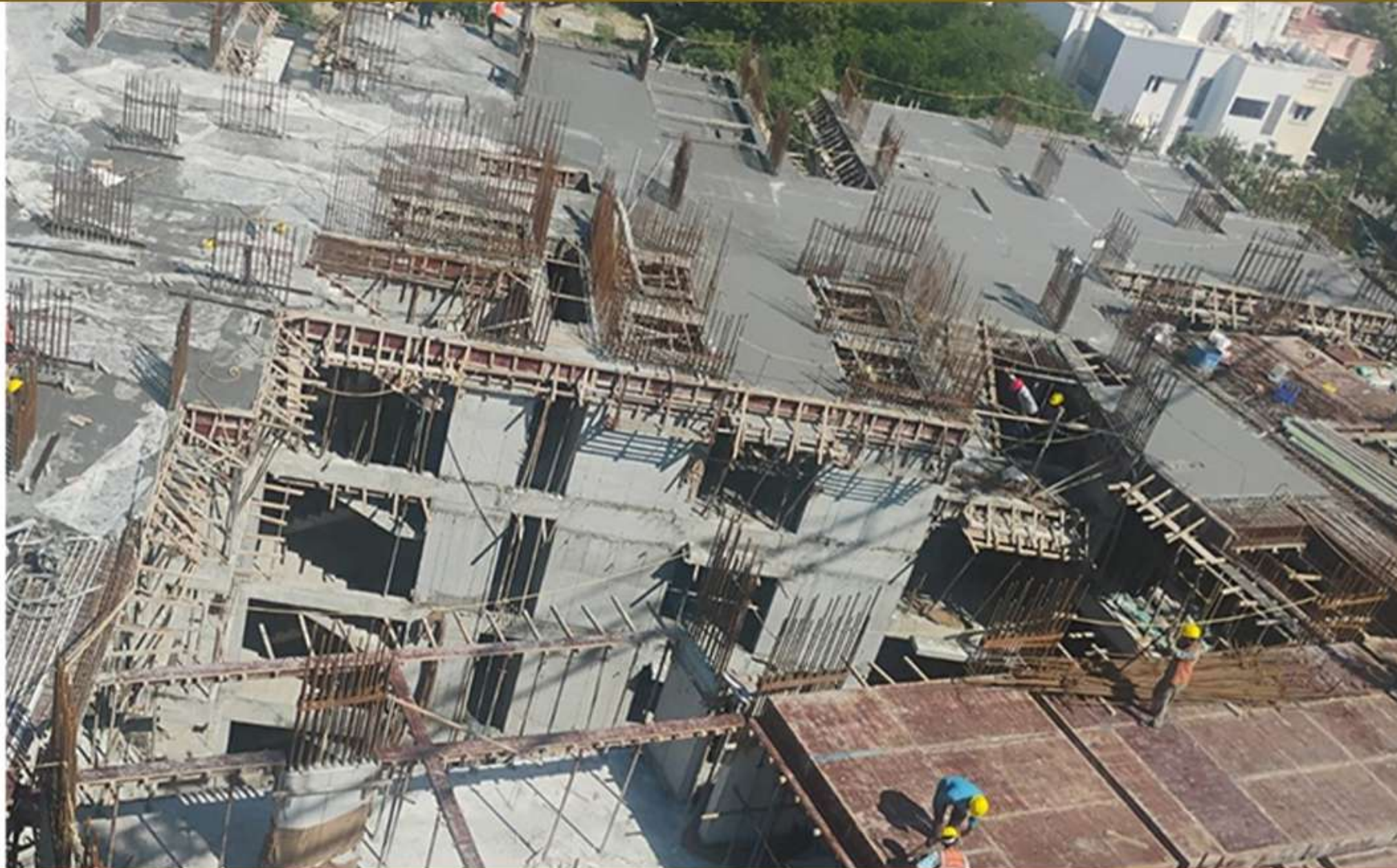
Block B – 4th Floor roof slab concrete work (pour-1)
