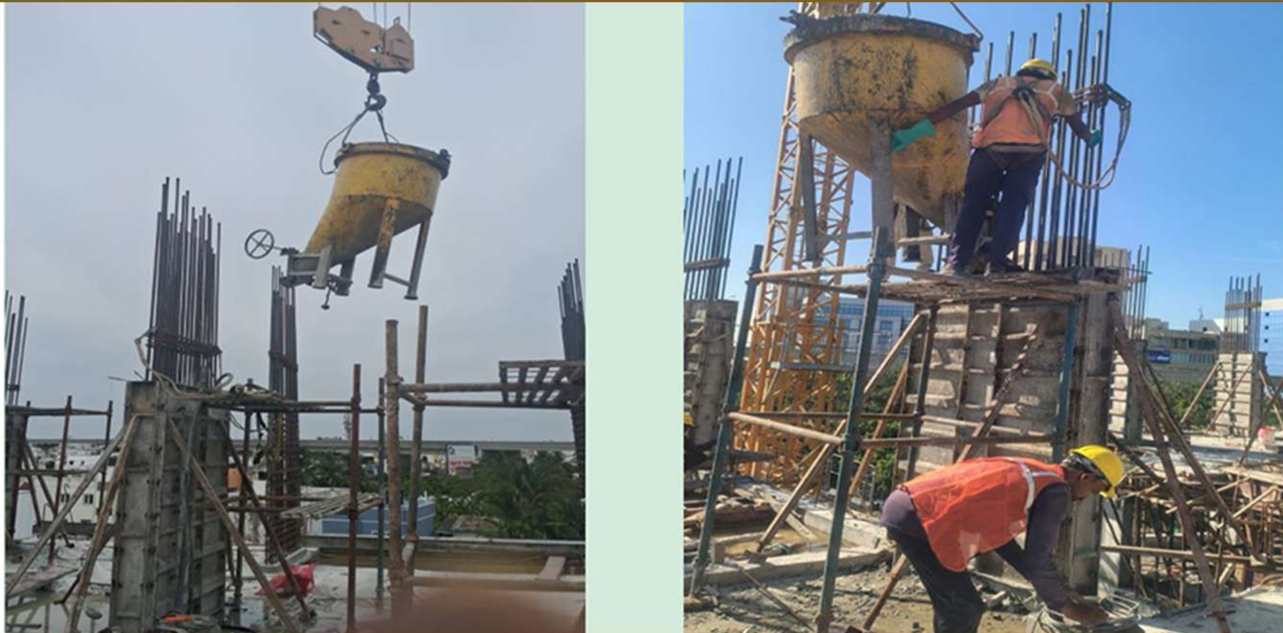
Block B – 4th Floor column concrete work
