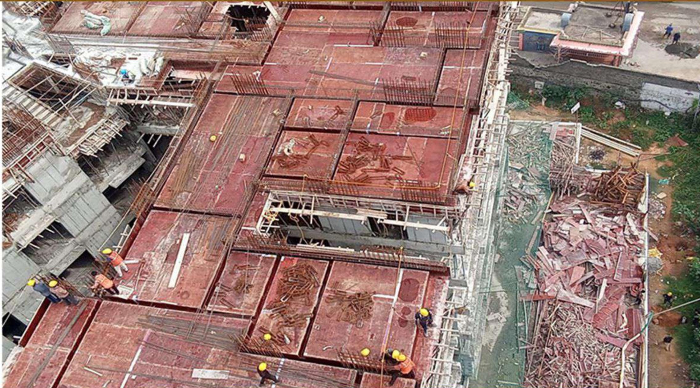
Block b – 6th floor roof slab Shuttering (Pour-2)
