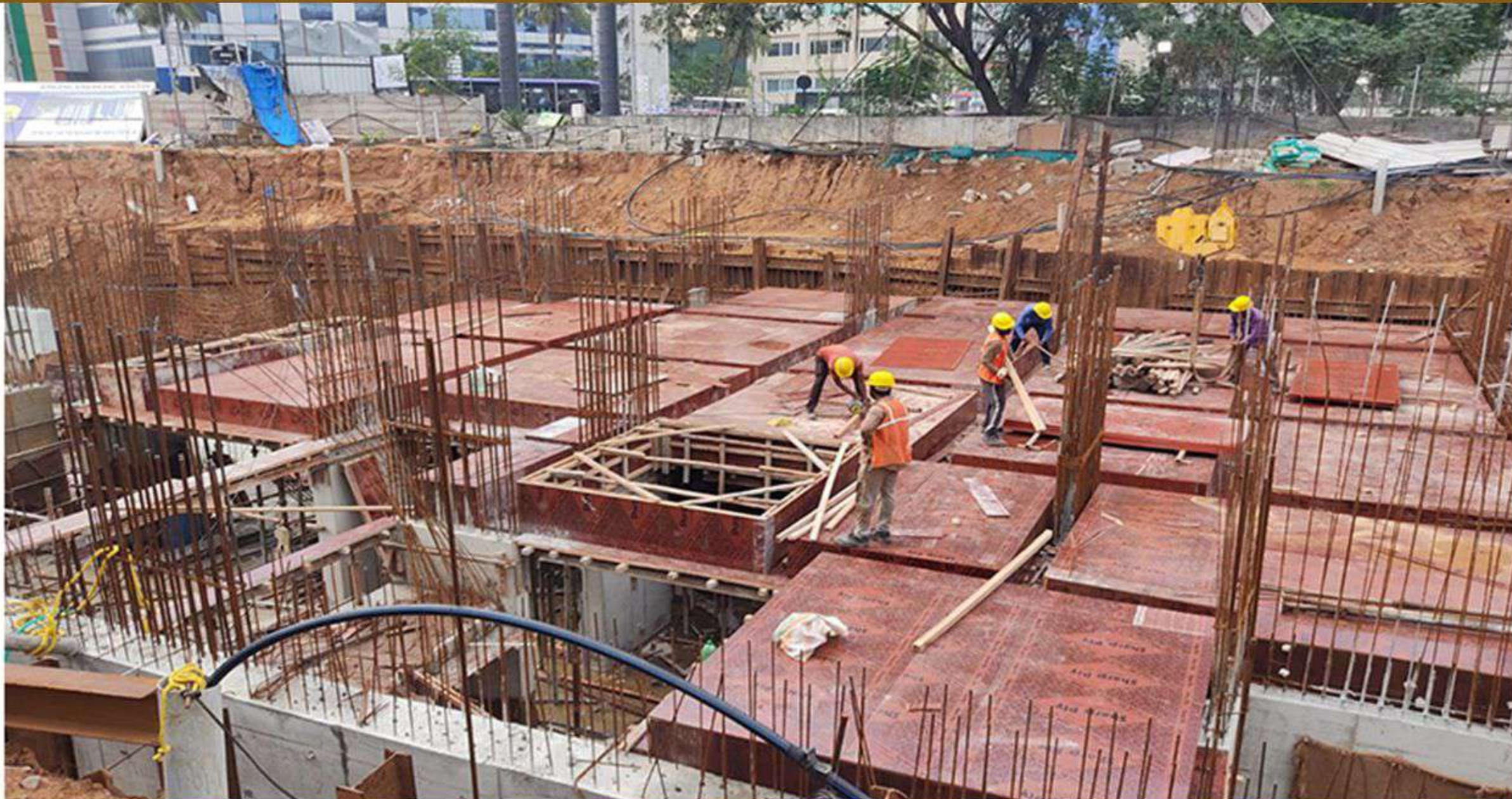
Block a – lower basement roof slab shuttering (pour-2)
