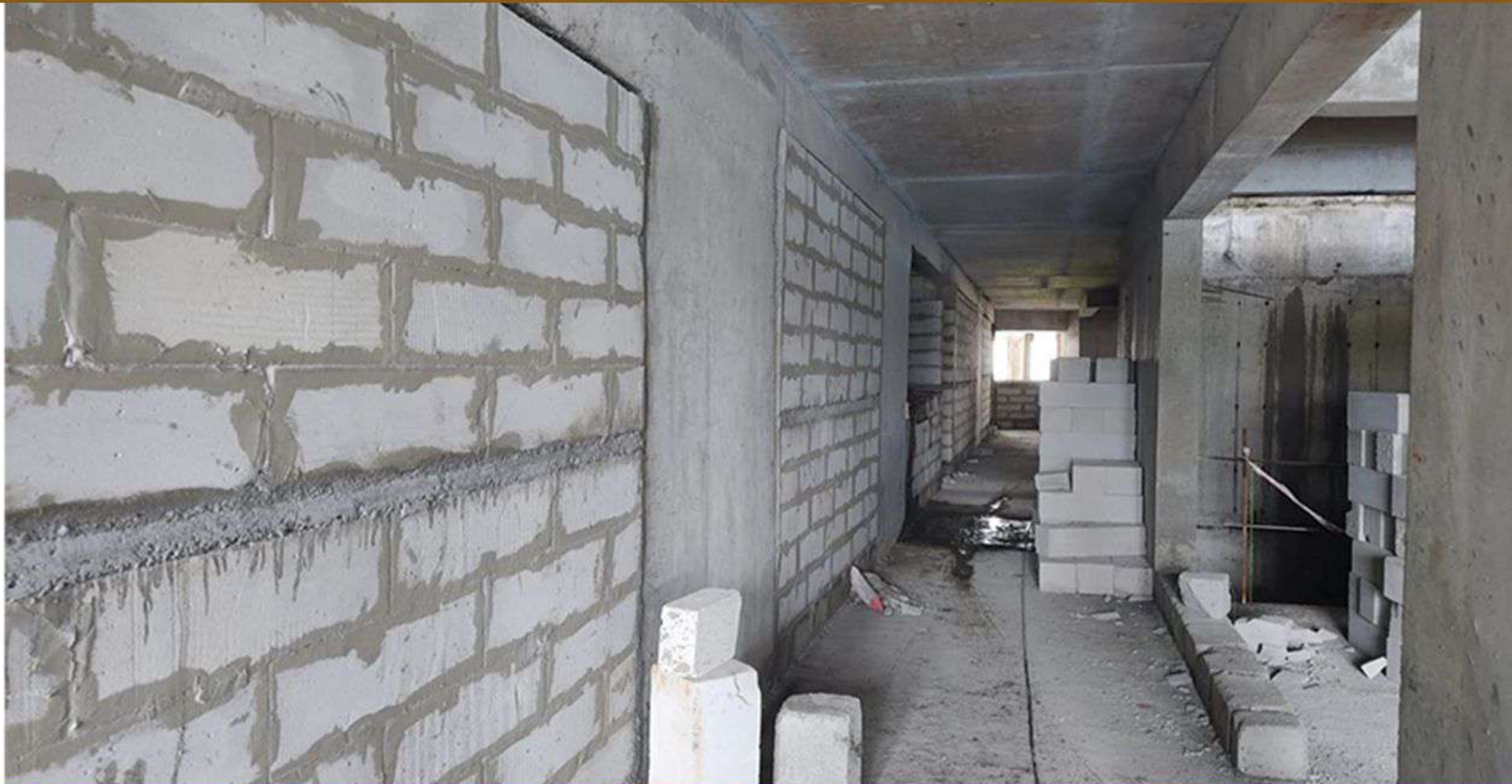
Block b – 2nd floor block work
