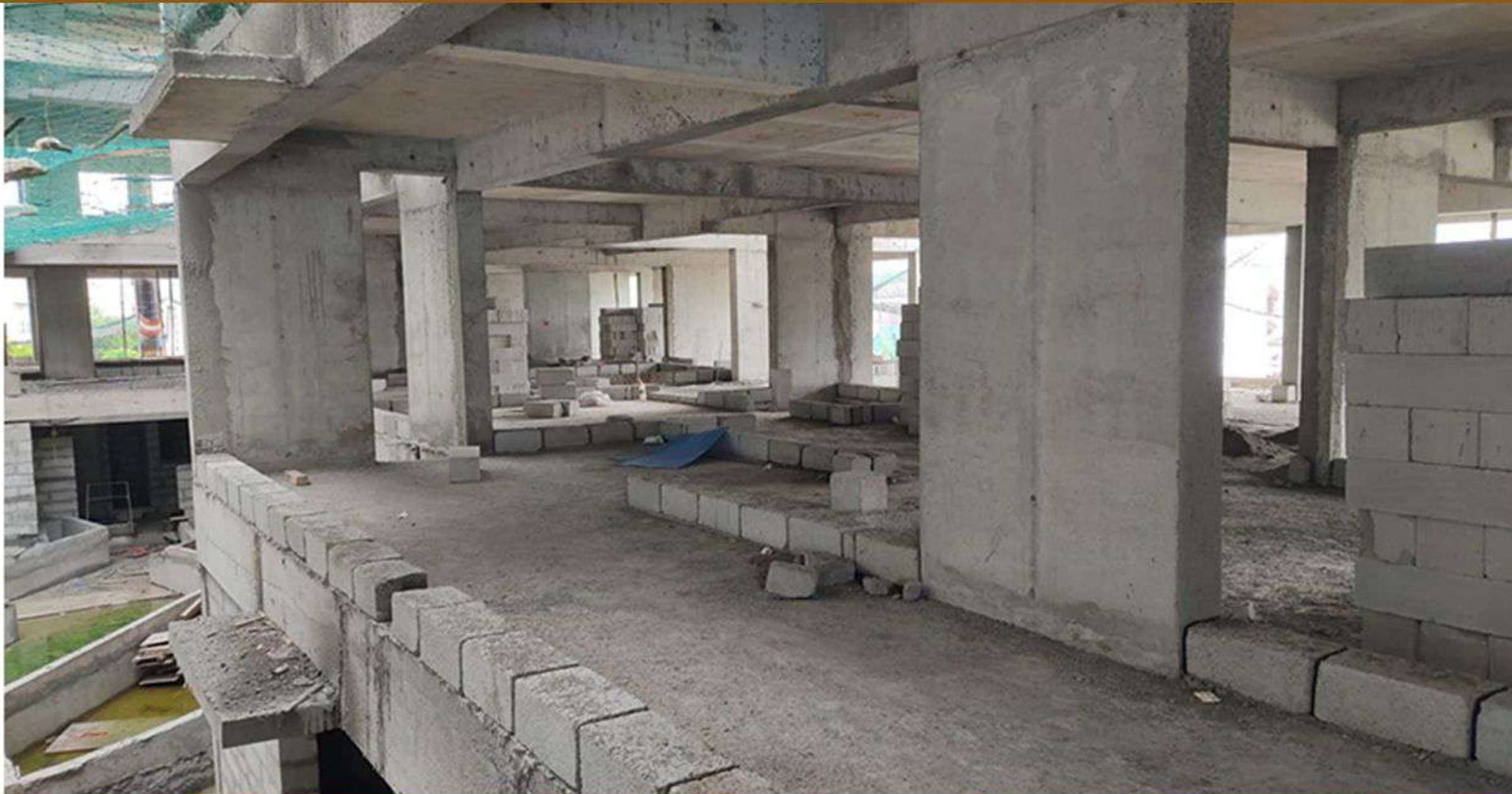
Block b – 2nd floor block work
