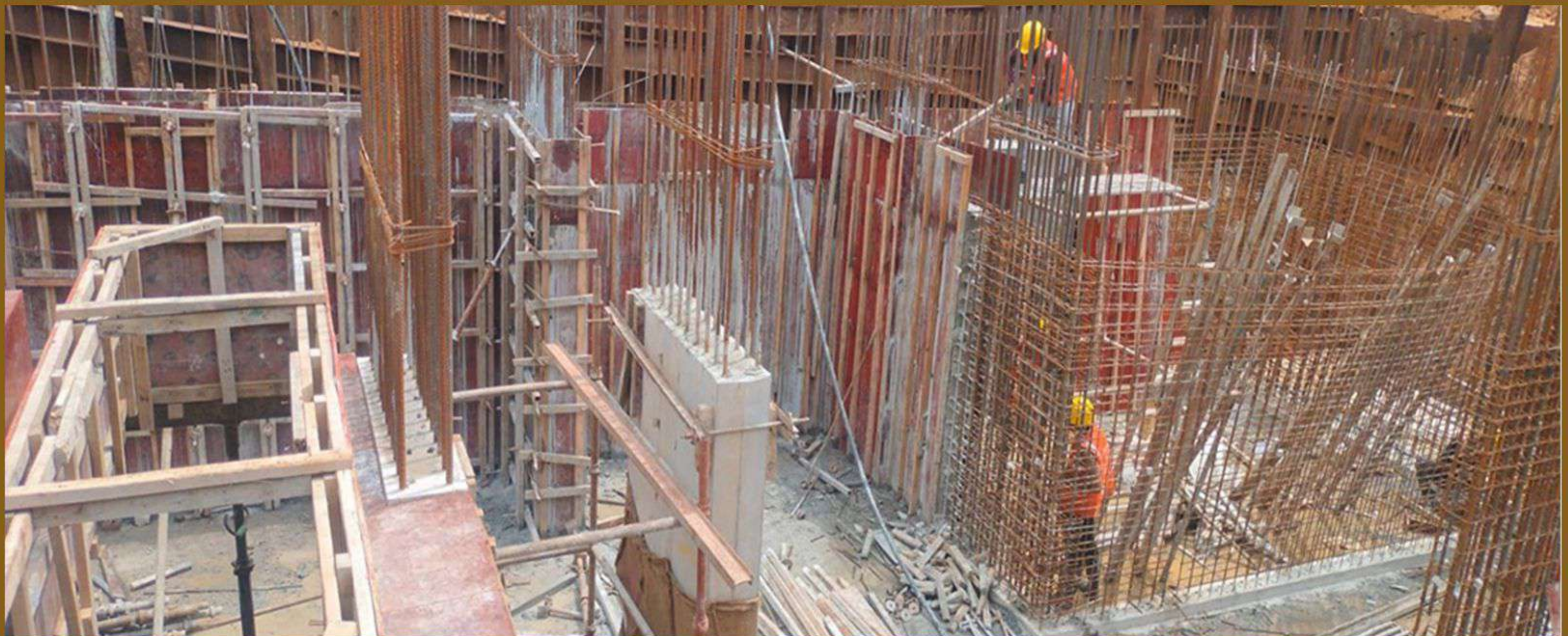
Block a – lower basement RC wall shuttering
