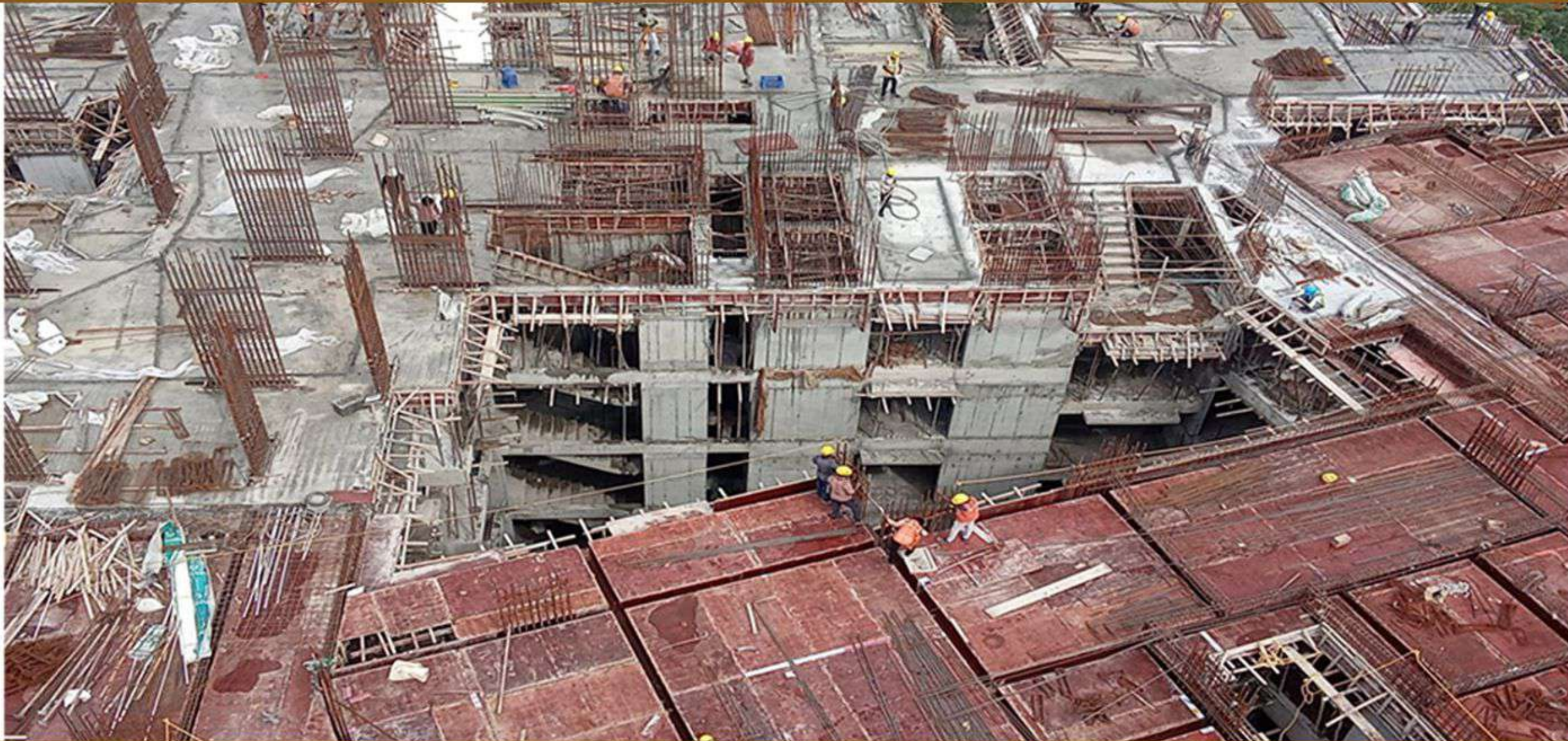
Block b – 6th floor roof slab concrete (Pour-1)
