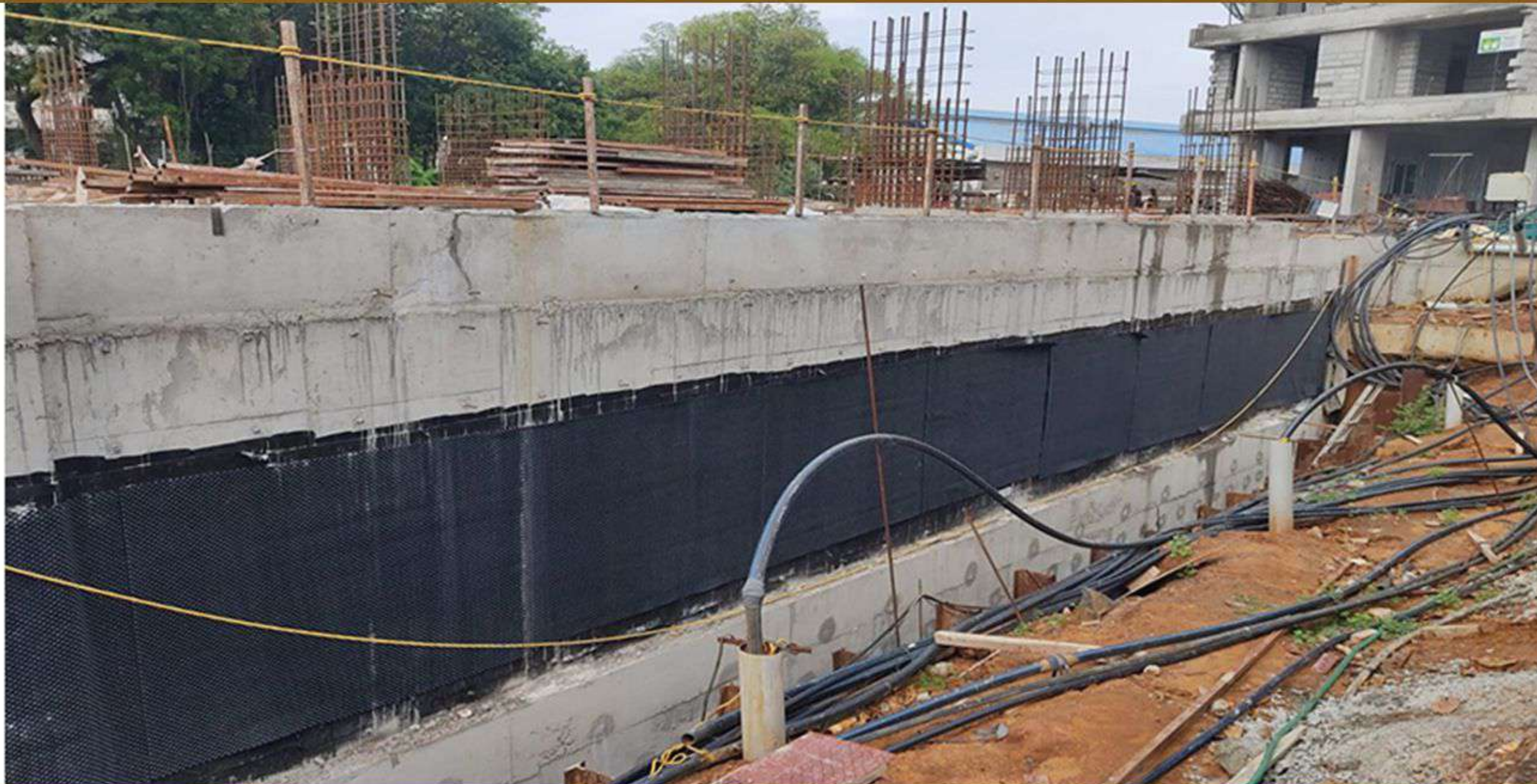
Block a – retaining wall waterproofing work
