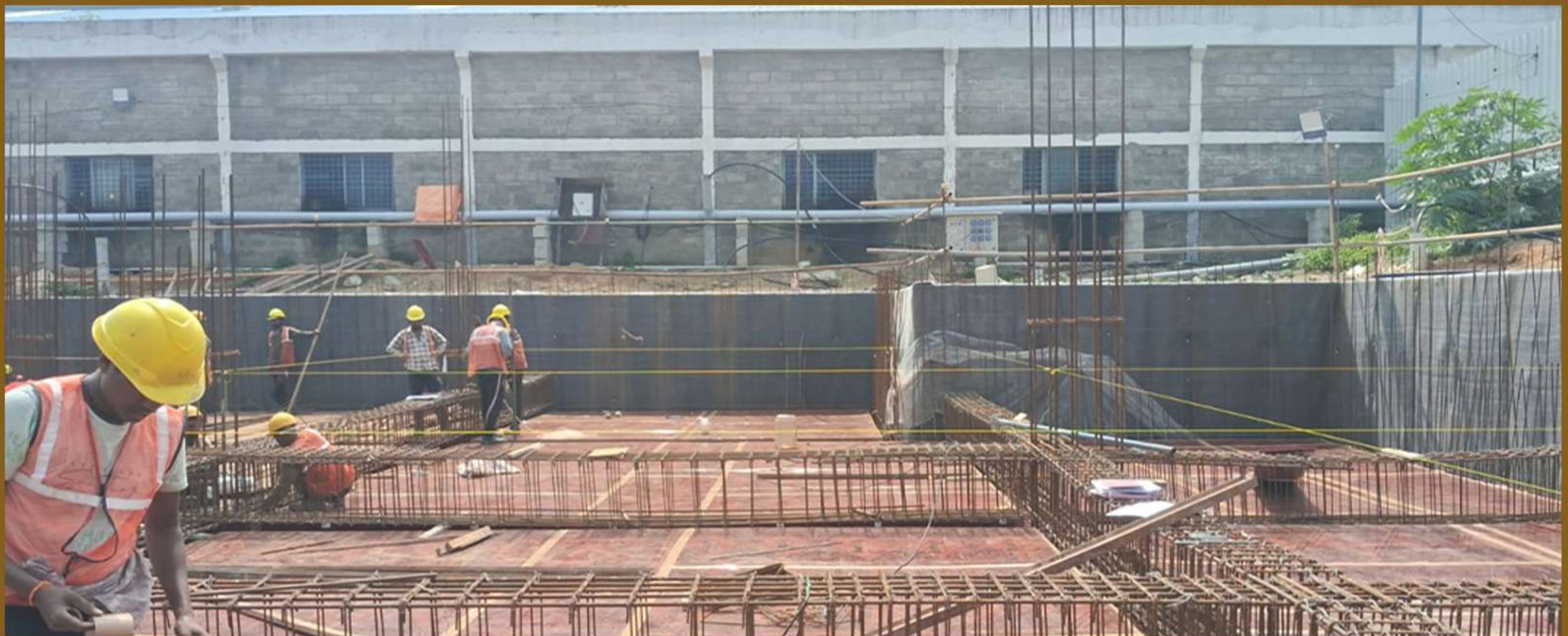
Block B slab reinforcement works
