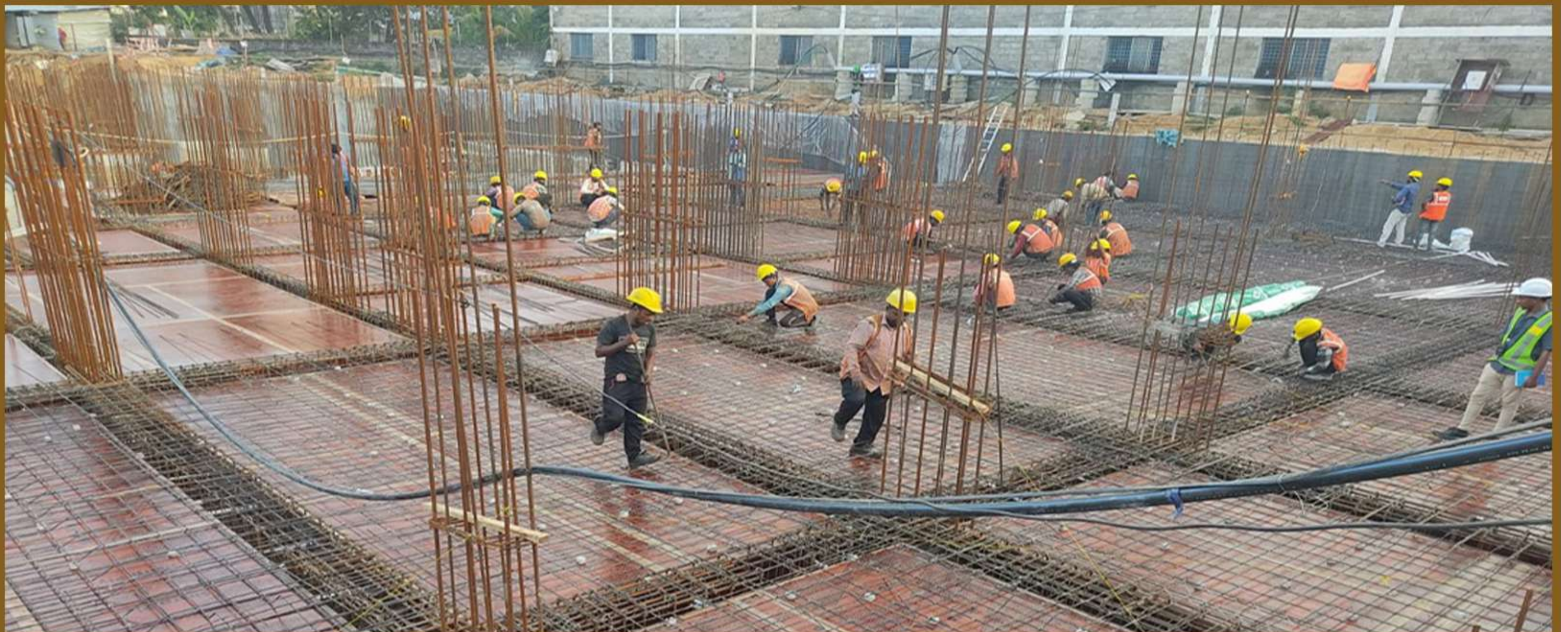
Block B slab reinforcement works
