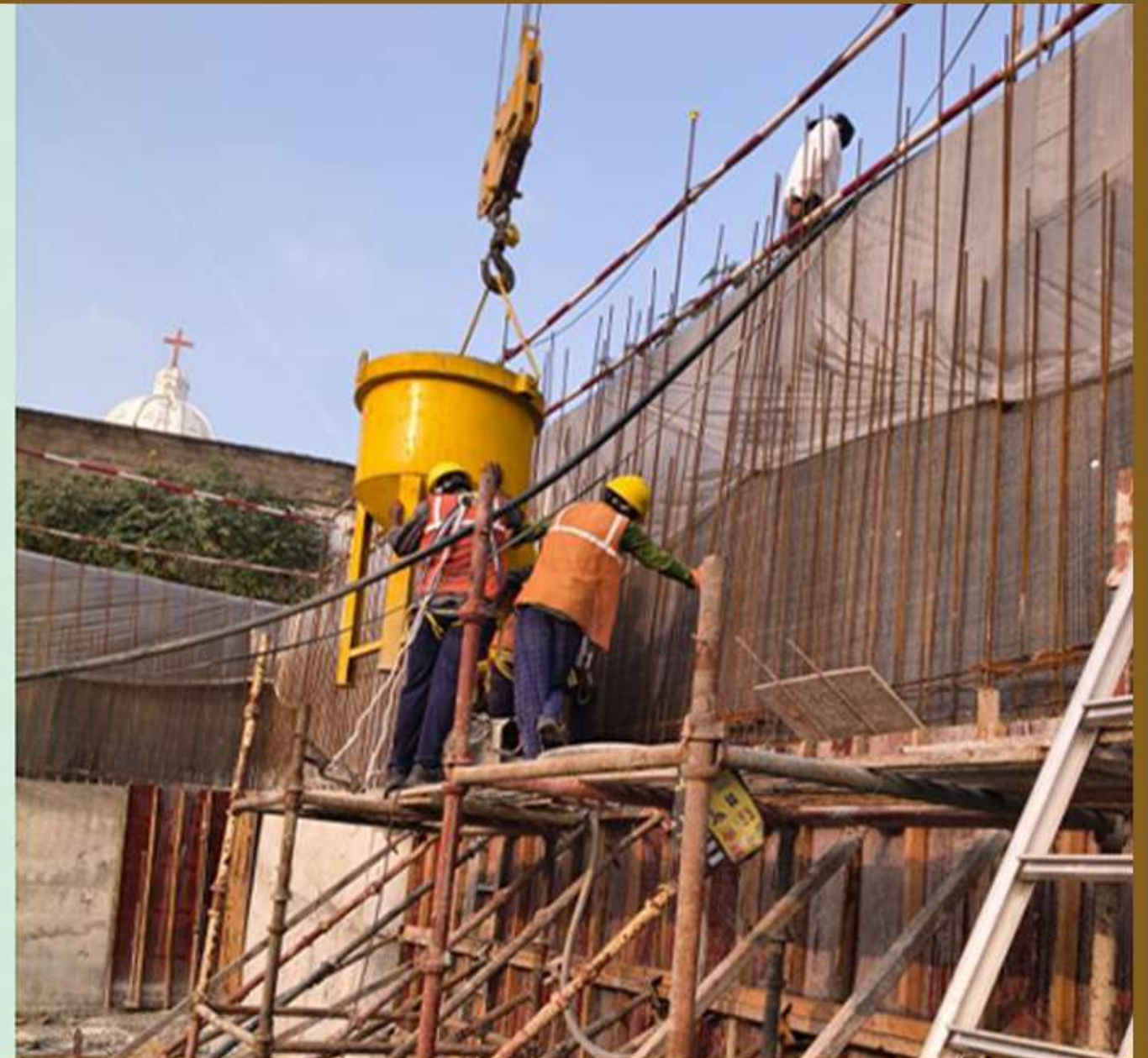
Block B RC-Wall concrete work in basement-2
