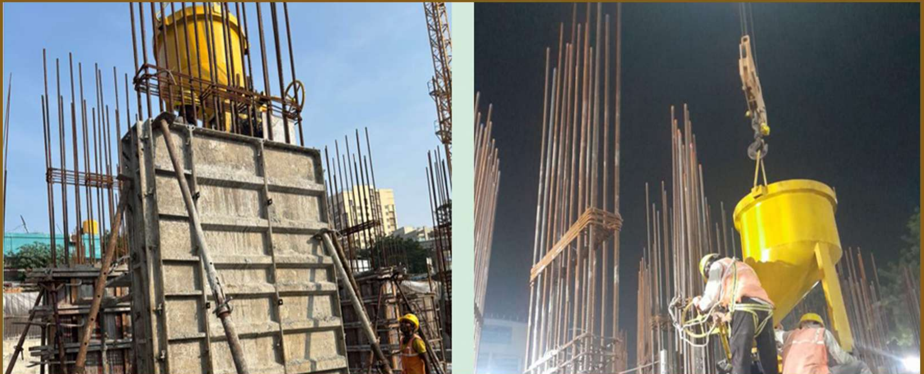
Block B column concrete work in basement-2
