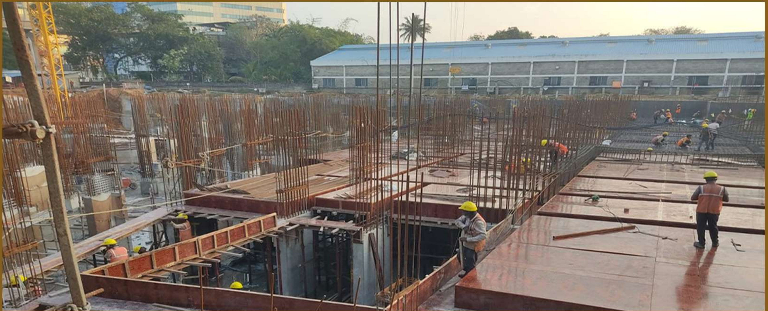
Block B roof slab shuttering work in basement-2
