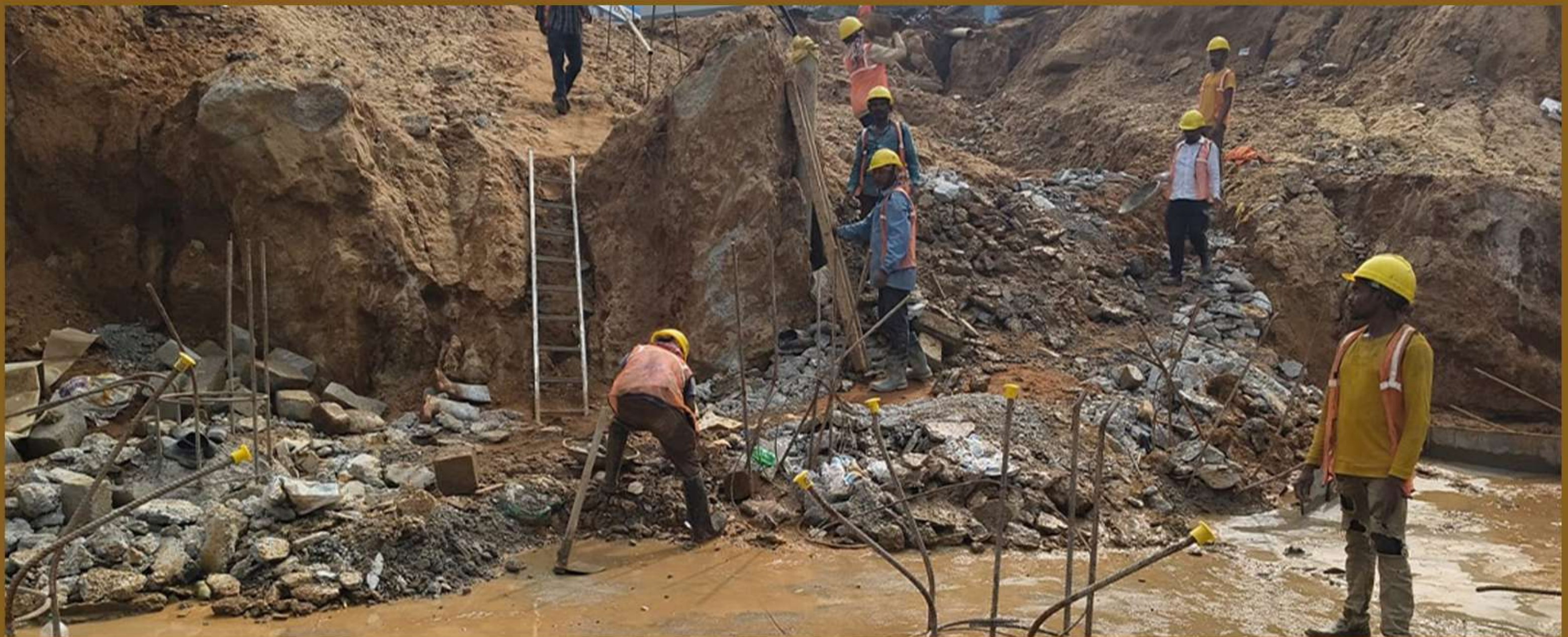
Block B slush removal works
