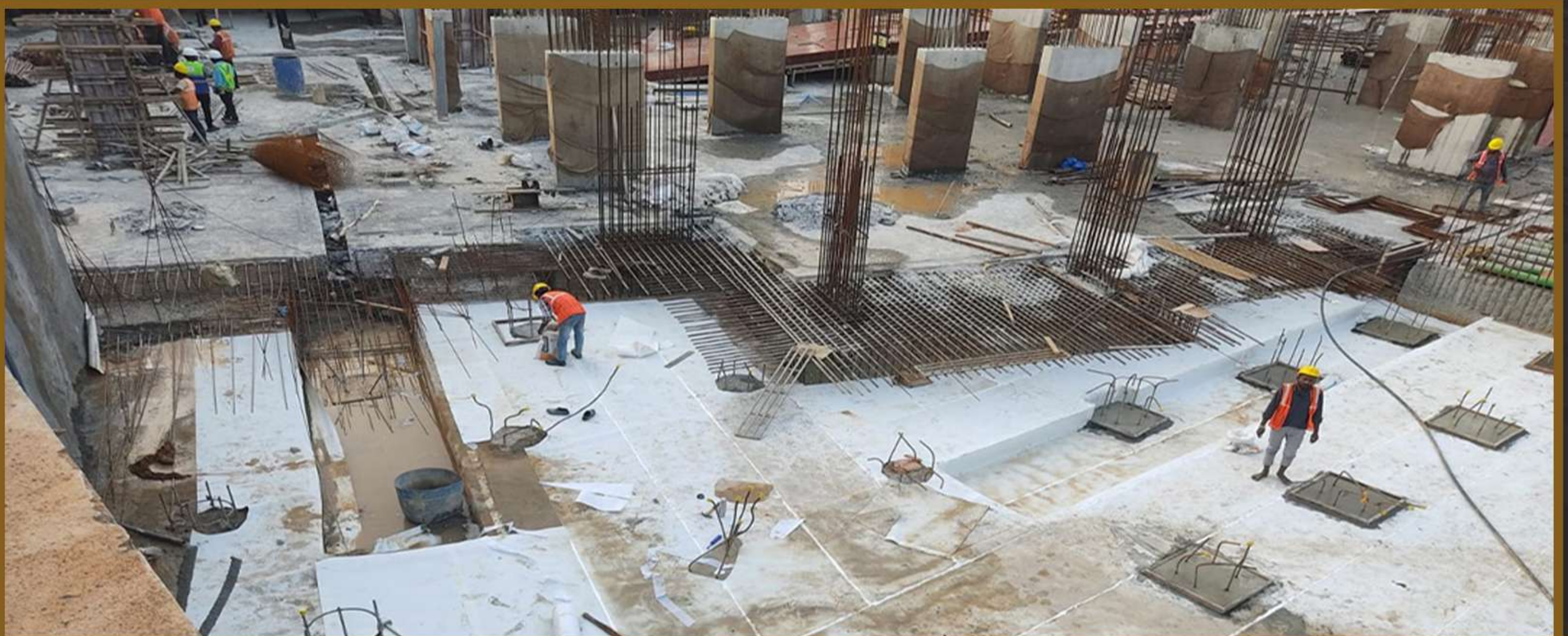
Block B raft water proofing work
