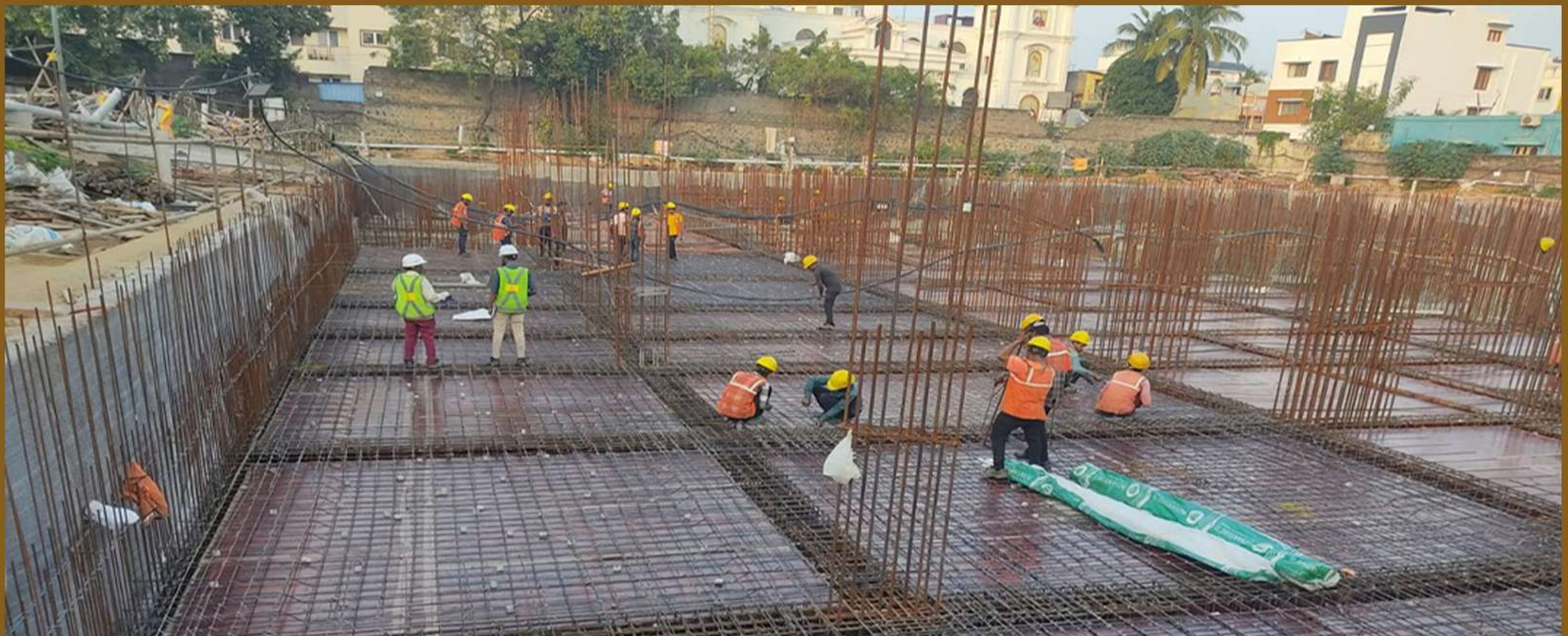
Block B slab reinforcement works
