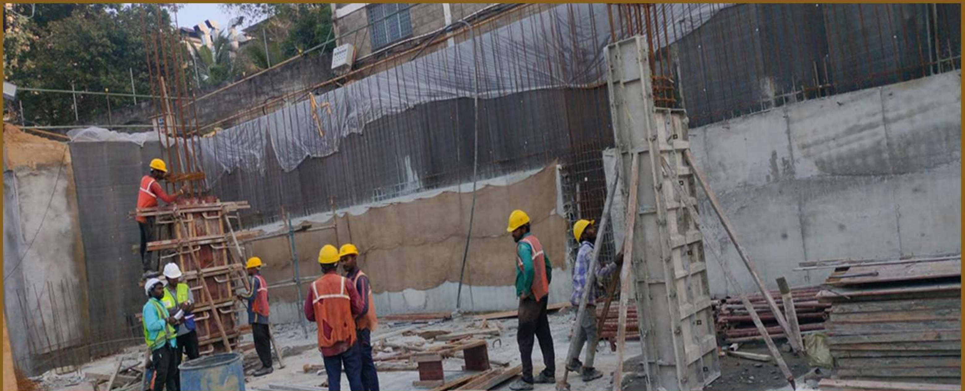
Block B column shuttering work in basement-2
