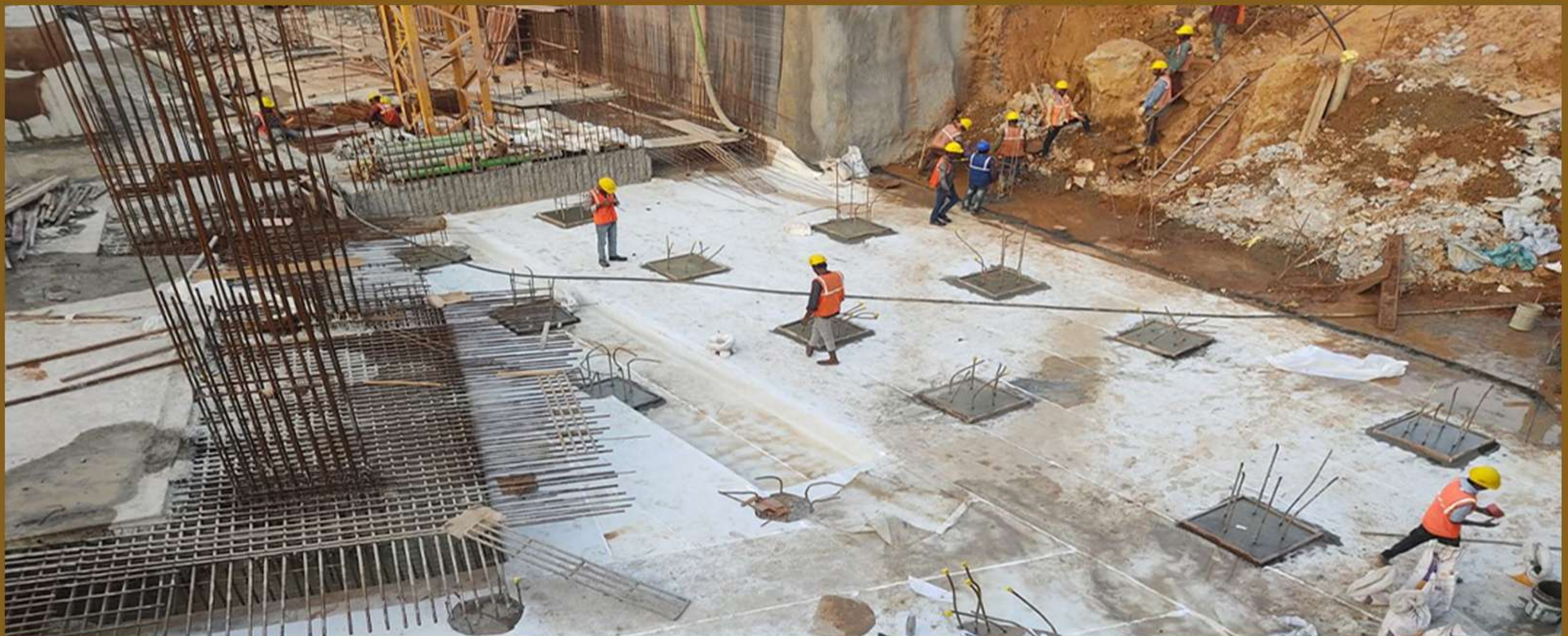
Block B raft water Proofing work
