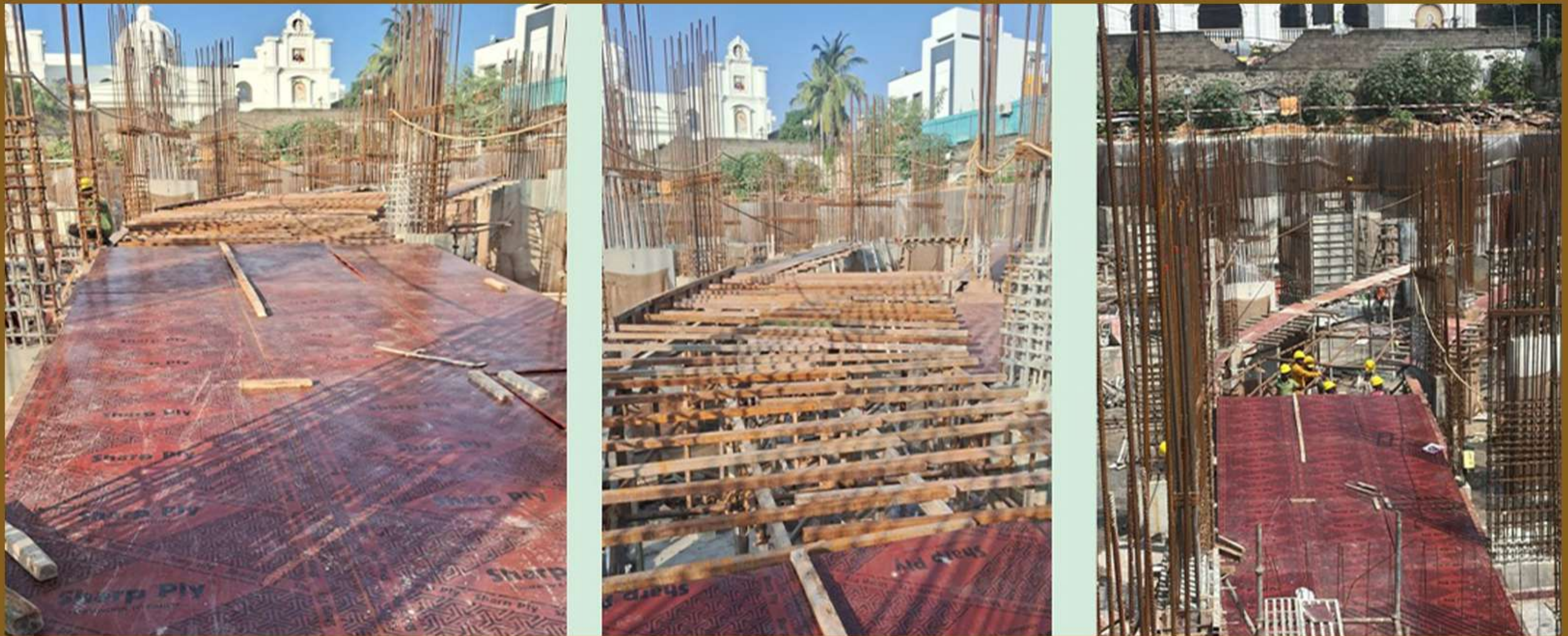
Block B ramp shuttering work in basement-2
