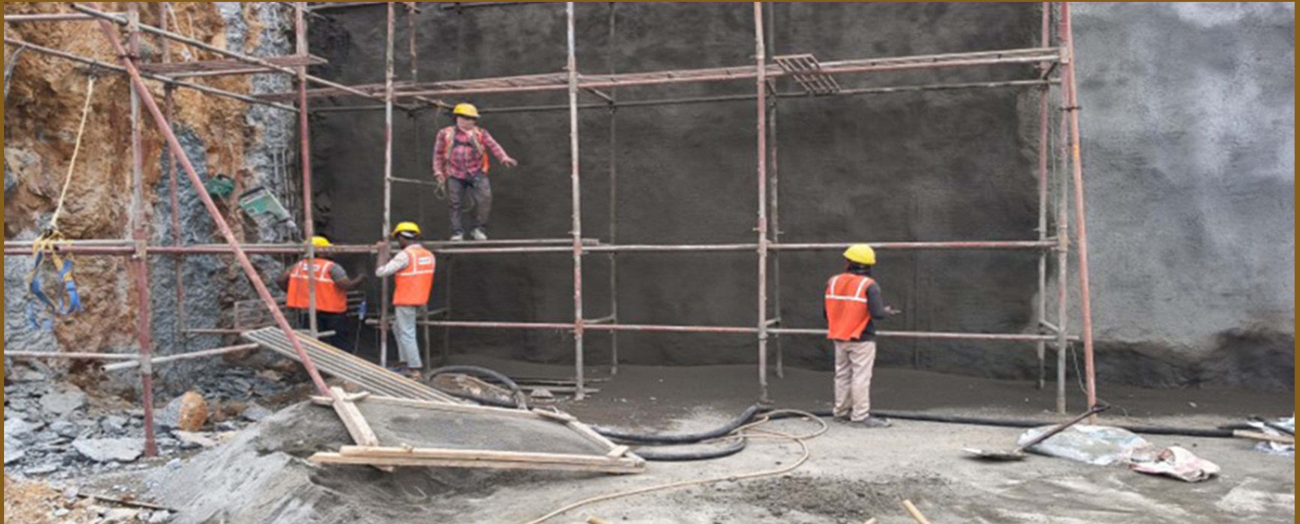
Block B short creating work
