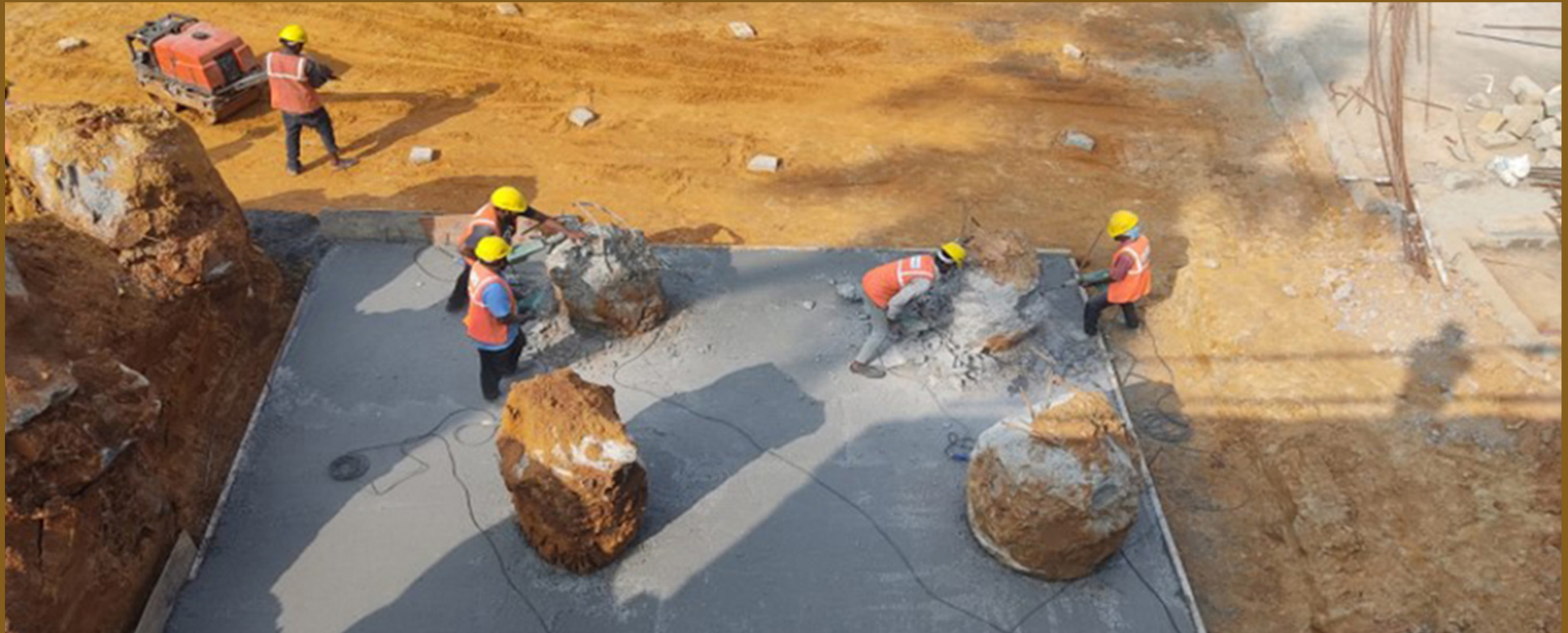
Block B tower crane Raft PCC laying
