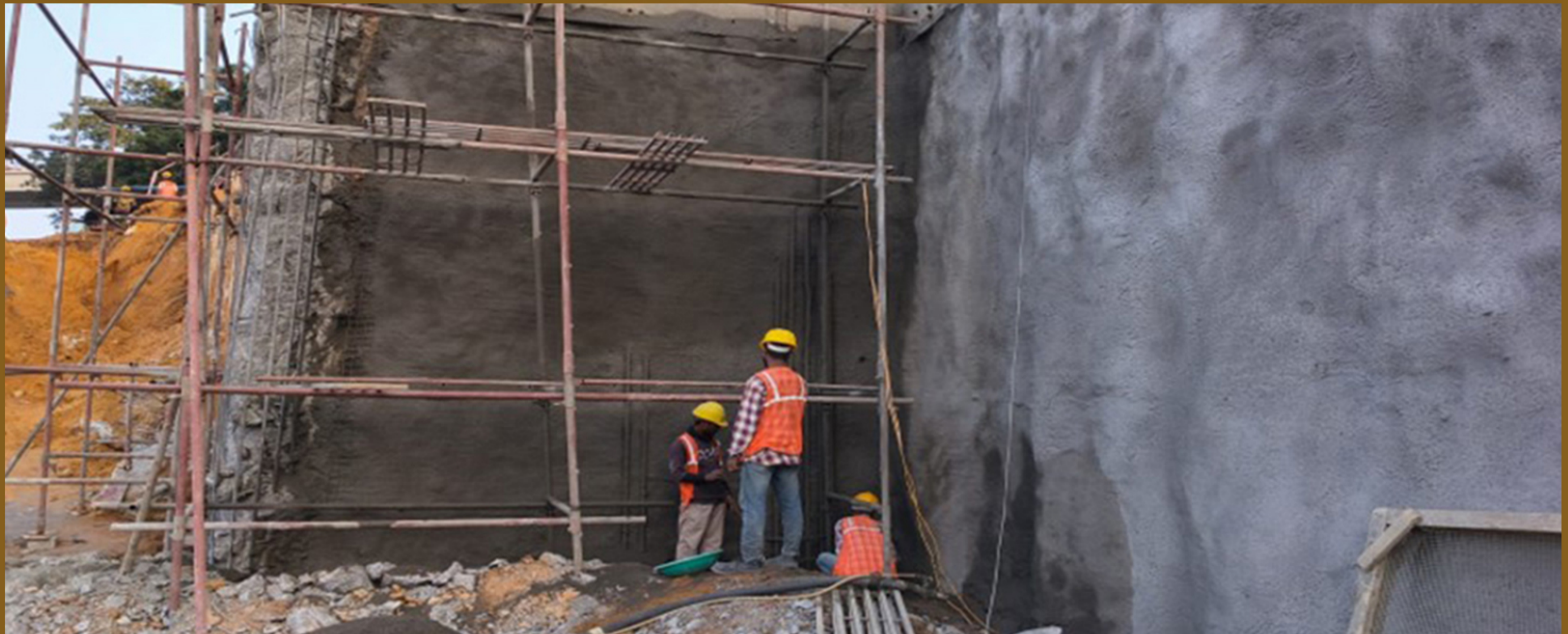
Block B short creating work
