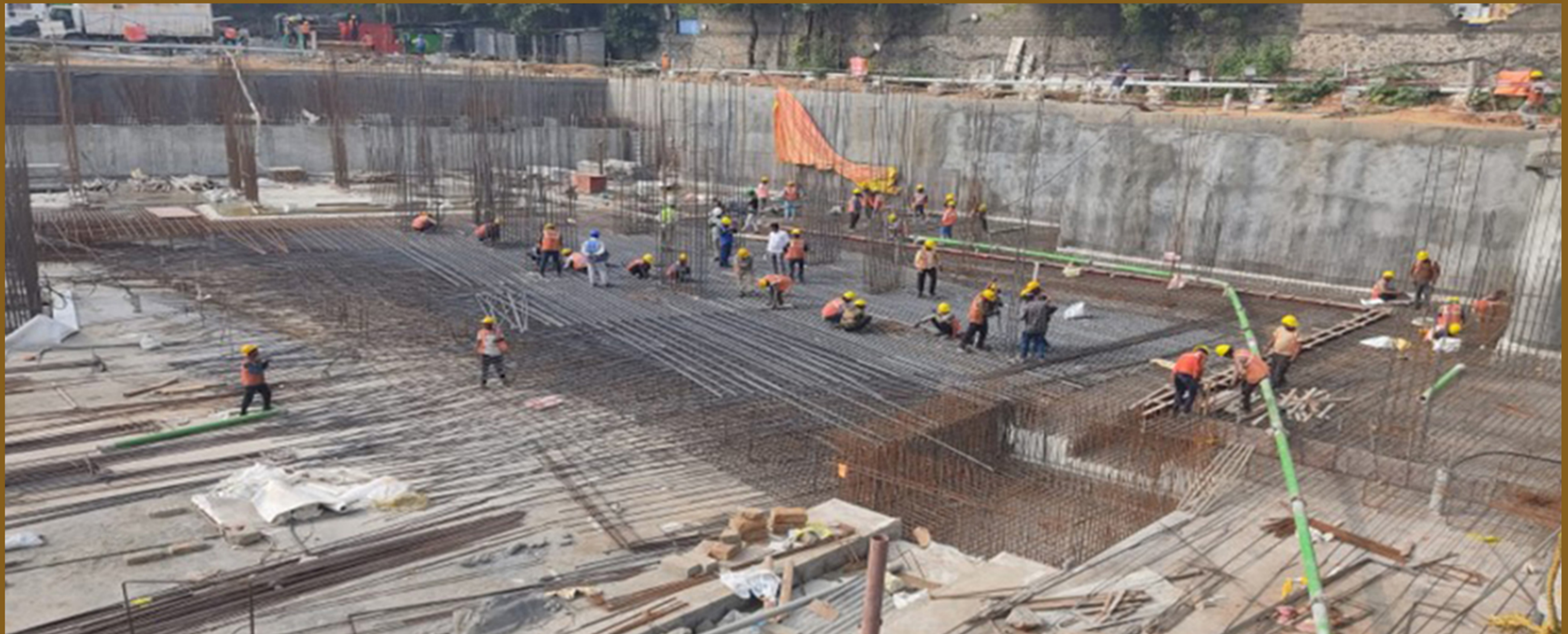
Block B raft reinforcement work
