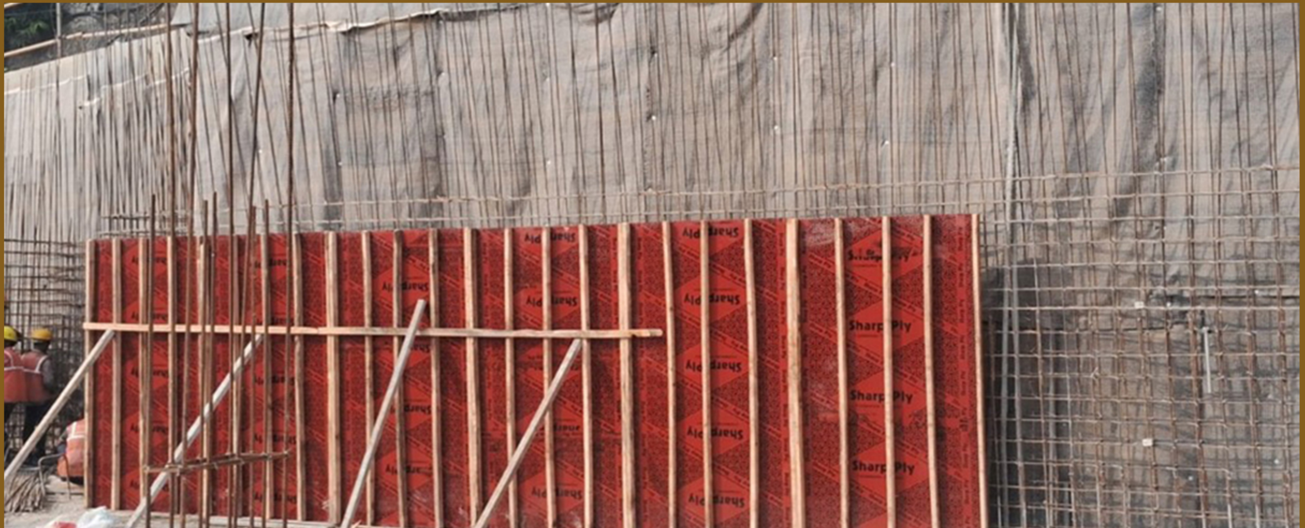
Block B Wall shuttering work
