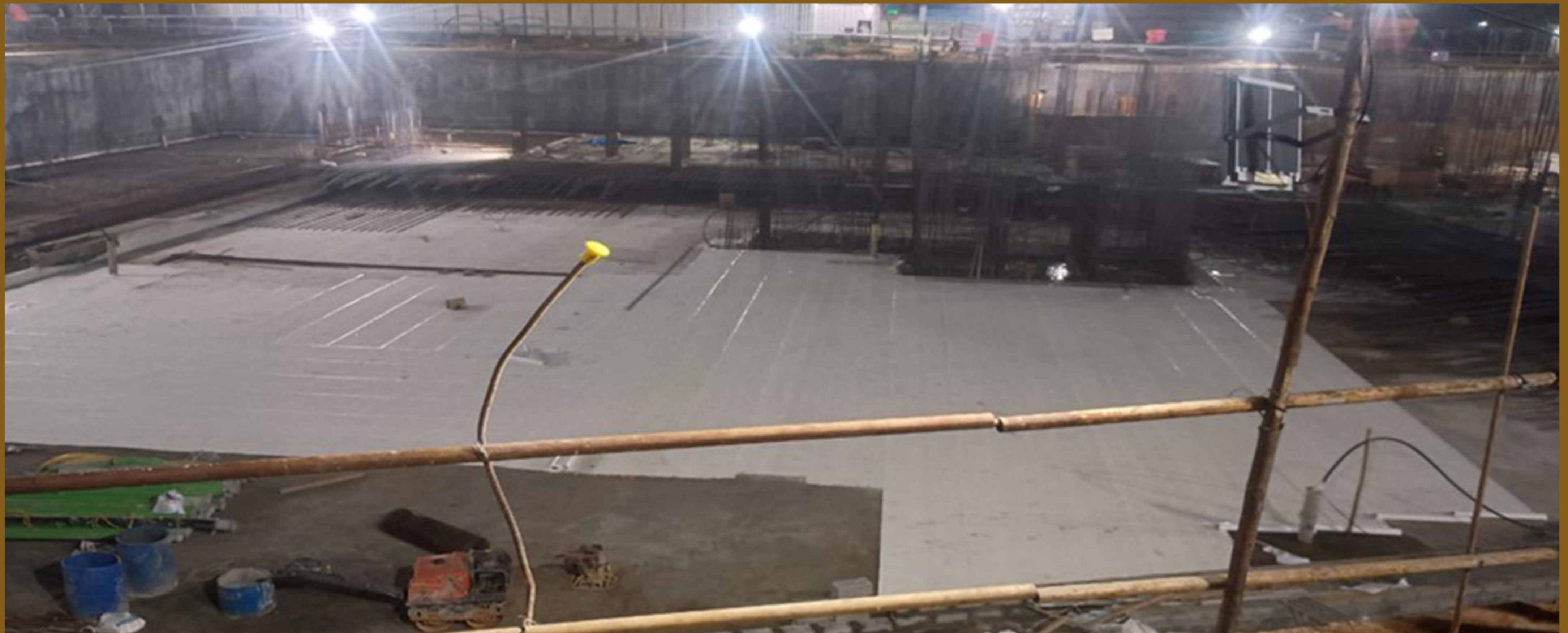
Block B raft water Proofing work
