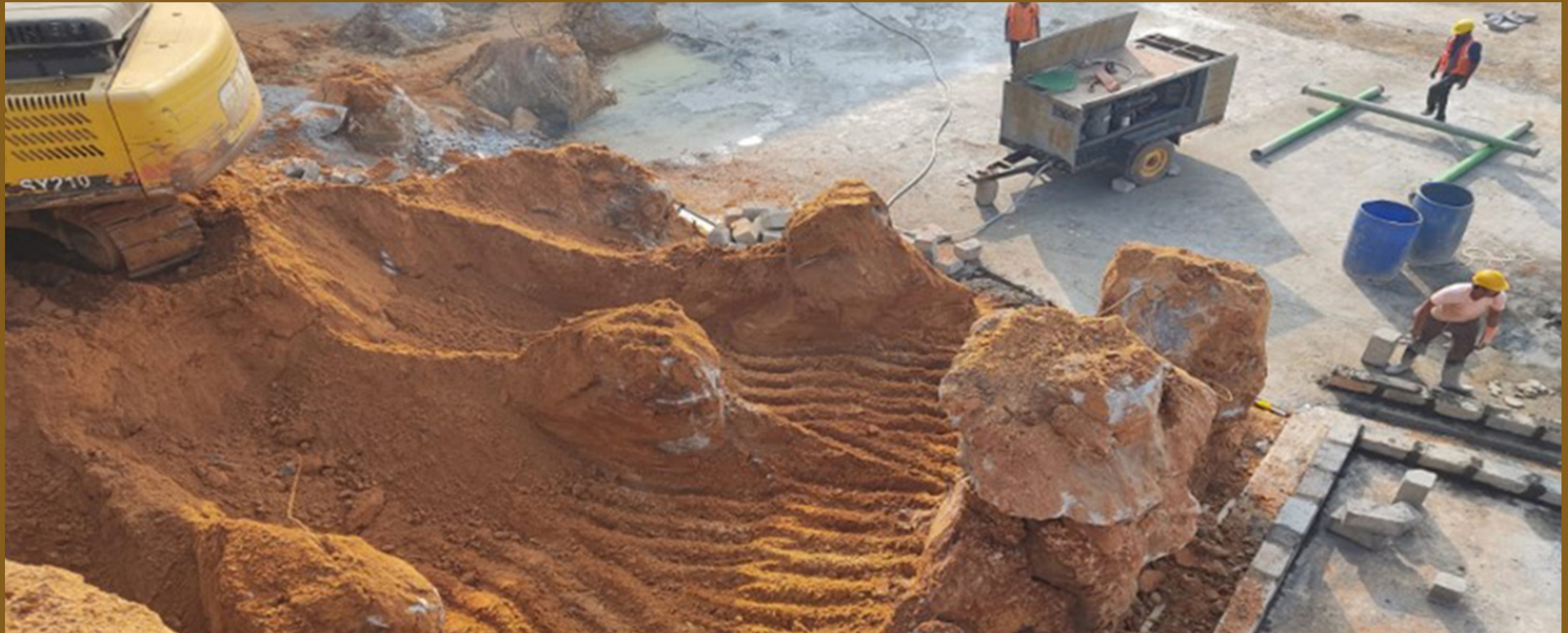
Block B stitch pipe area earth dressing works
