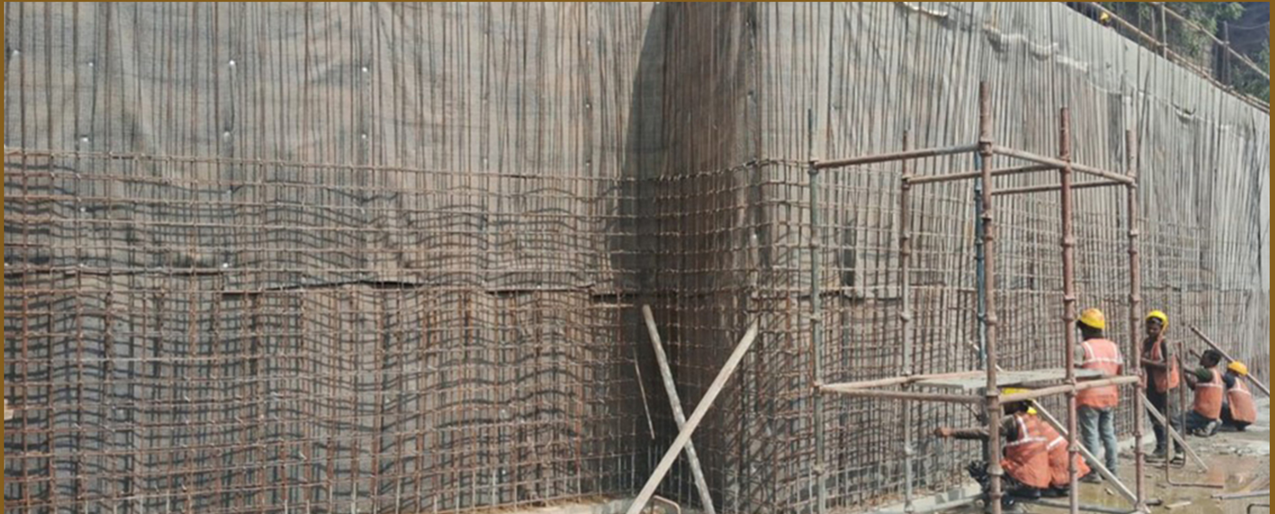
Block B Wall reinforcement work
