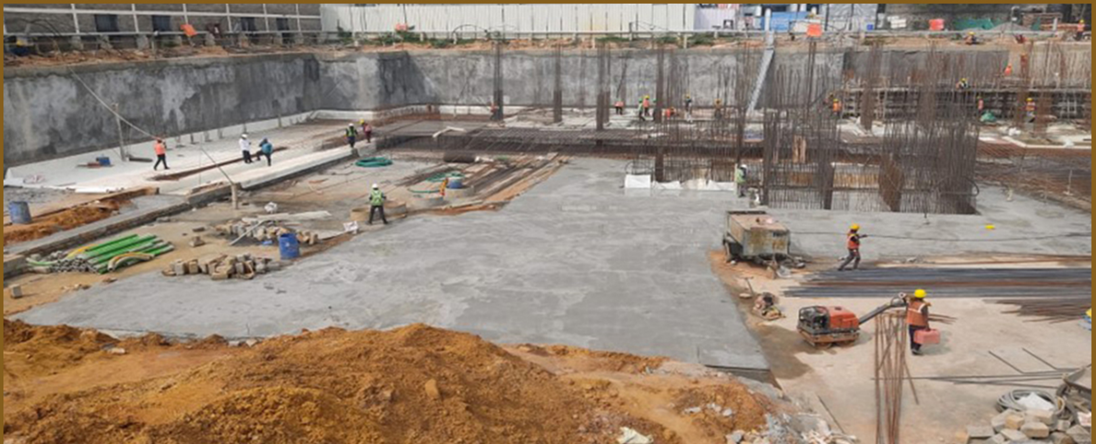
Block B Raft PCC laying
