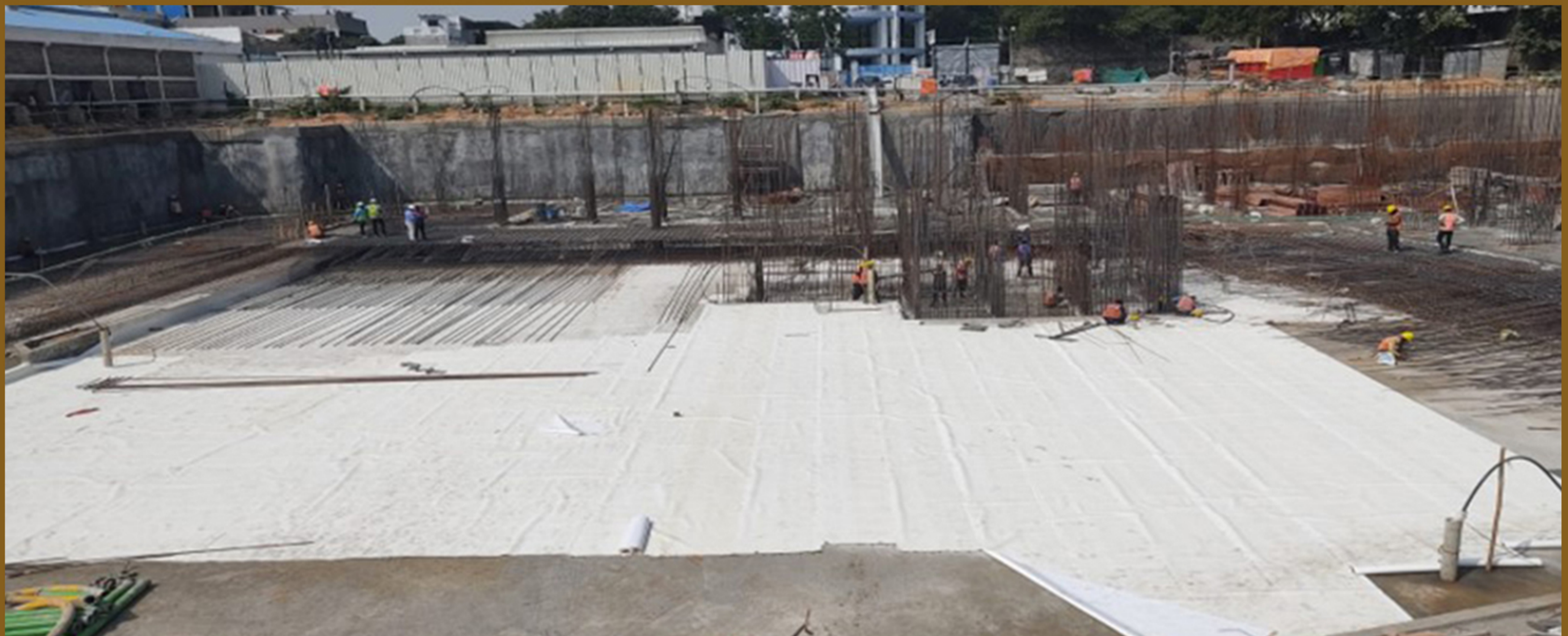
Block B raft reinforcement work
