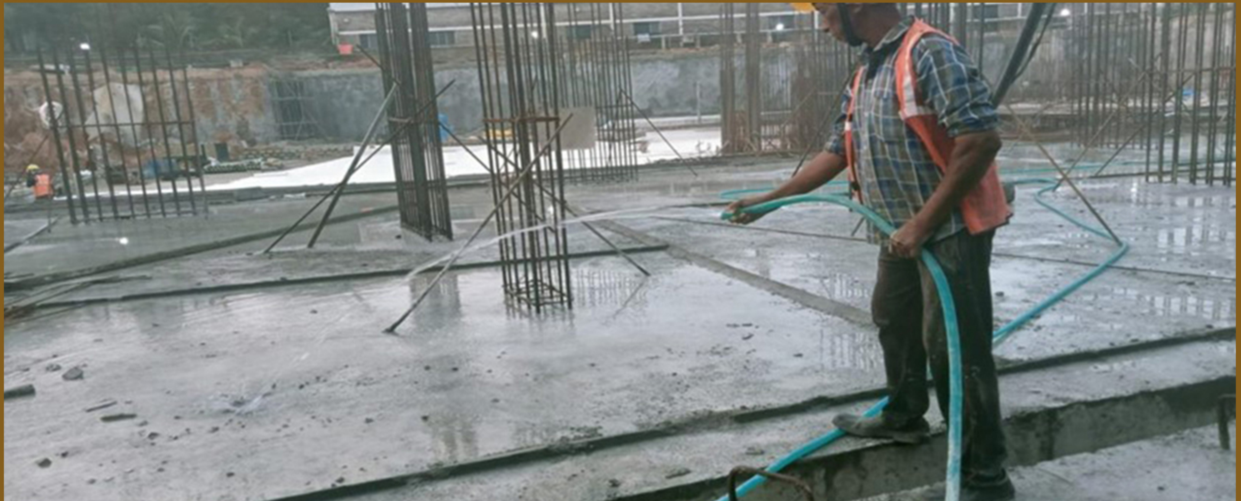
Block B Concrete curing work
