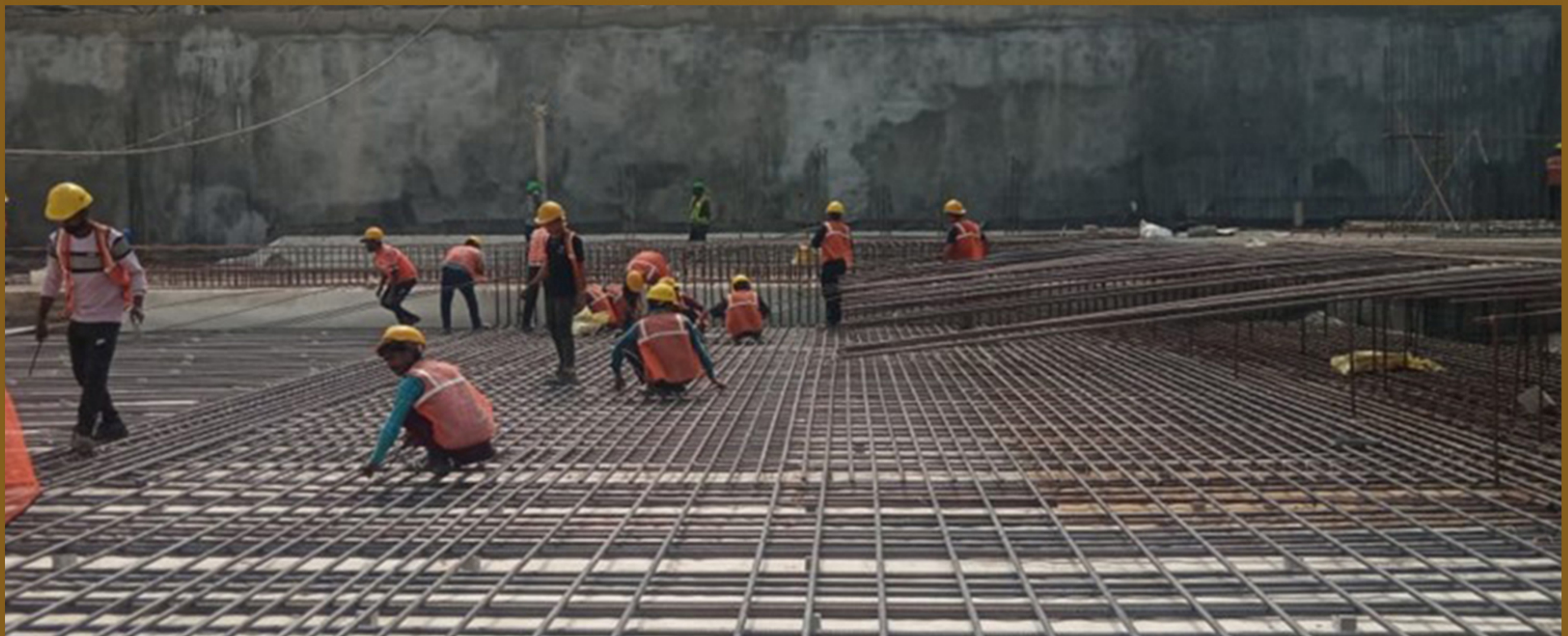
Block B raft reinforcement work
