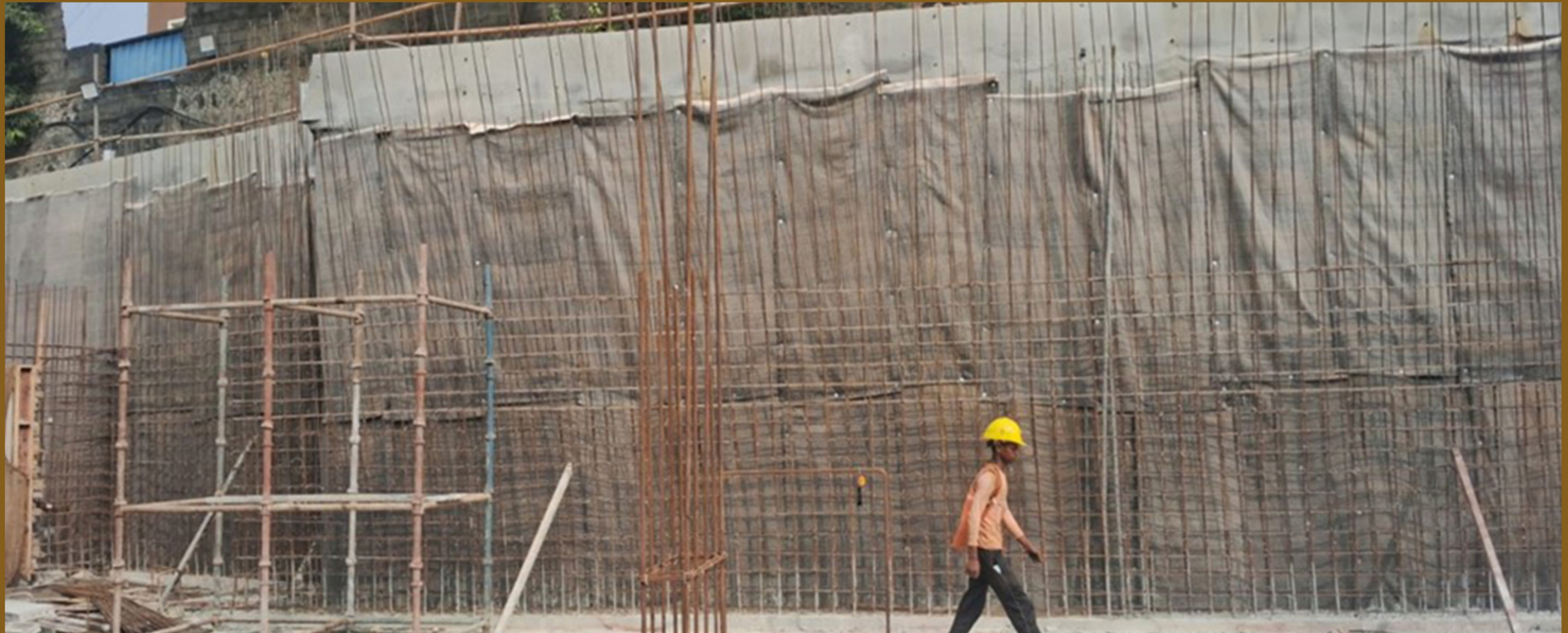
Block B Wall reinforcement work
