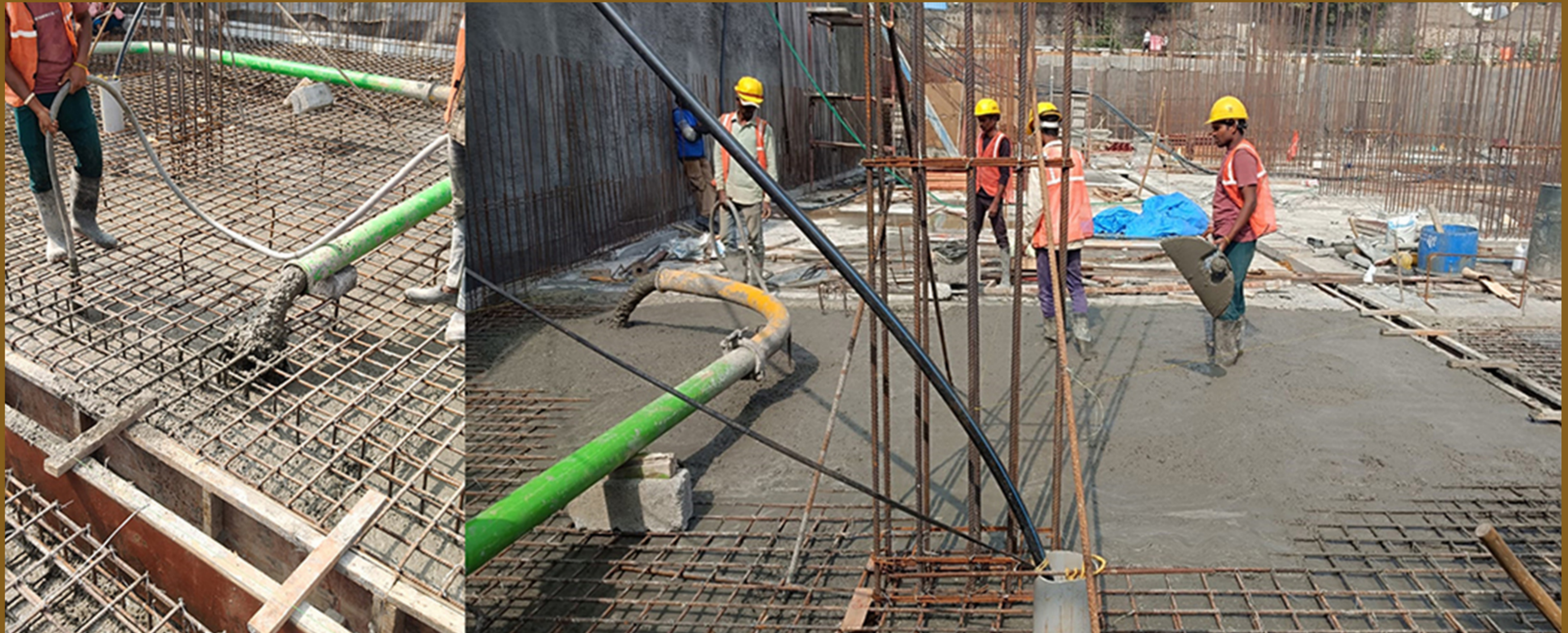
Block B raft concrete work
