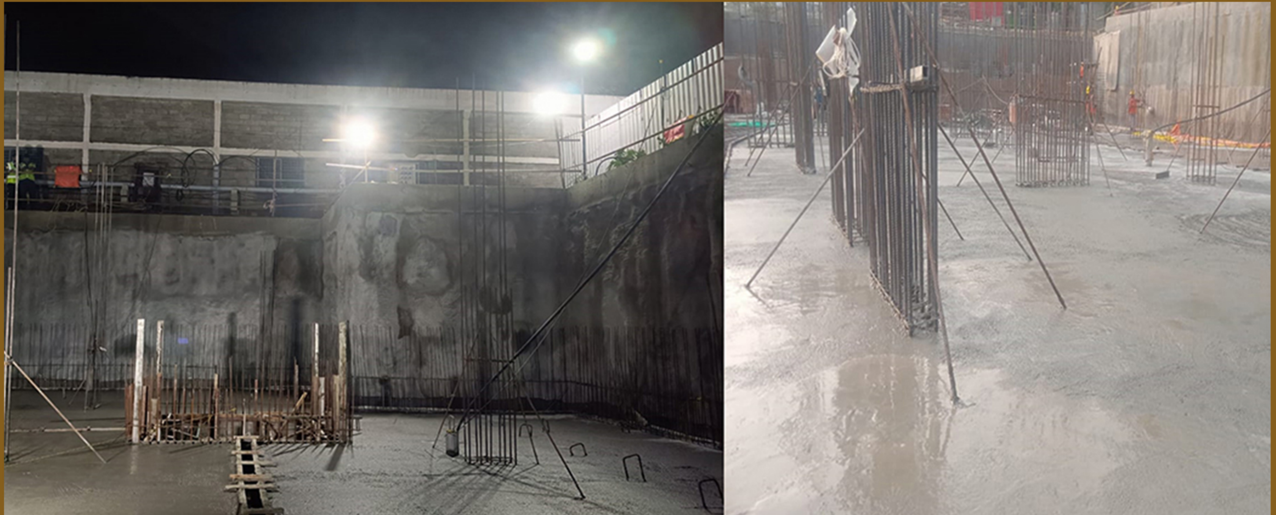
Block B raft reinforcement work
