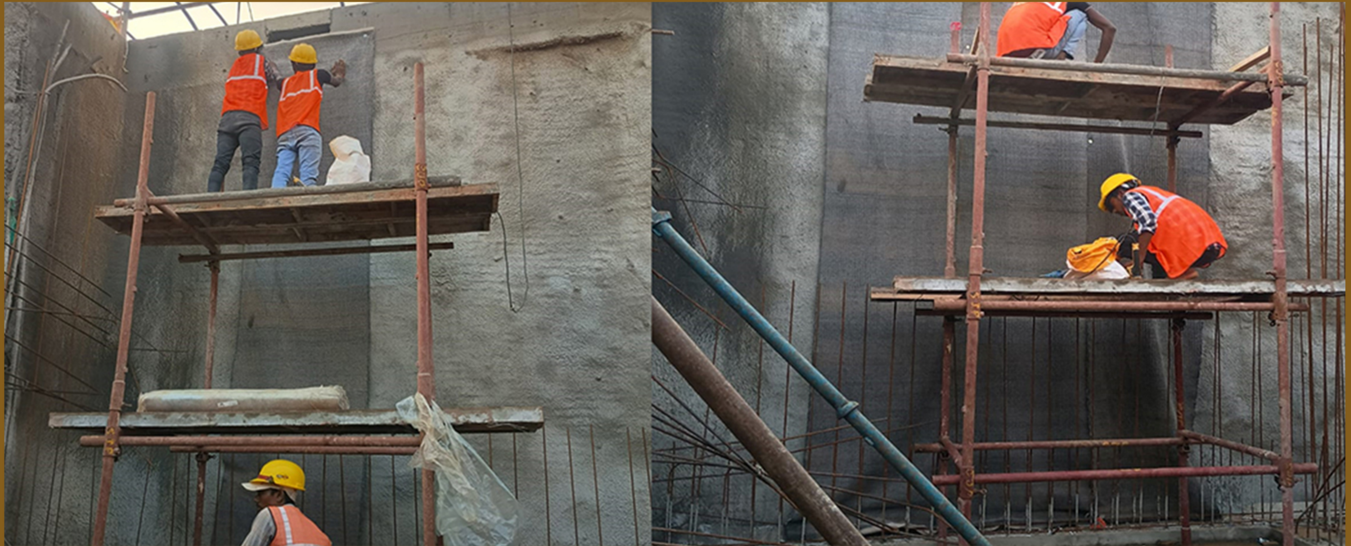
Block B RC-wall water Proofing work
