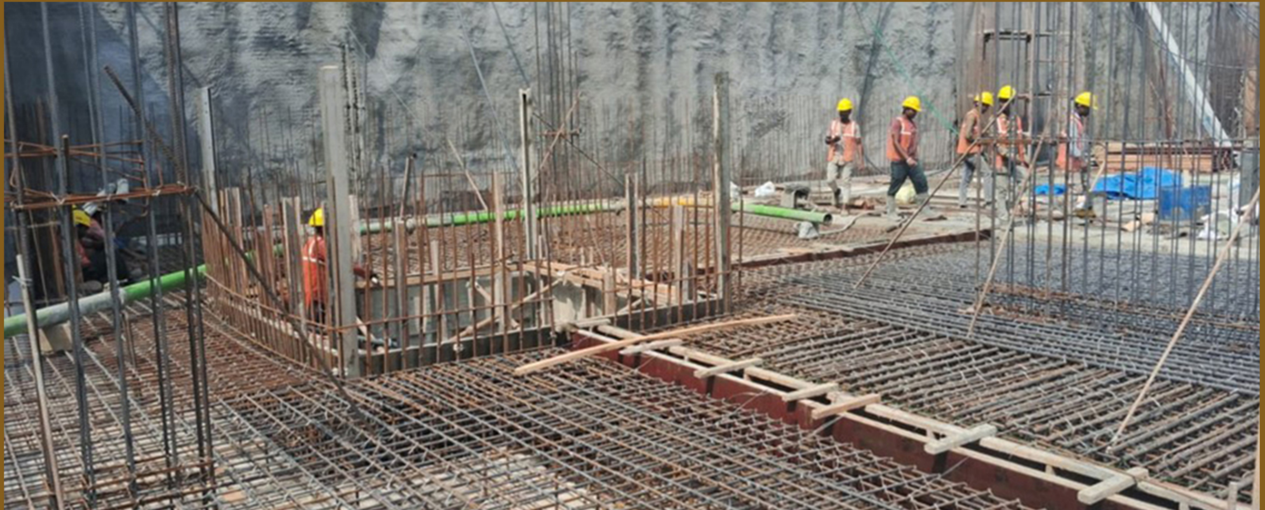
Block B raft reinforcement work
