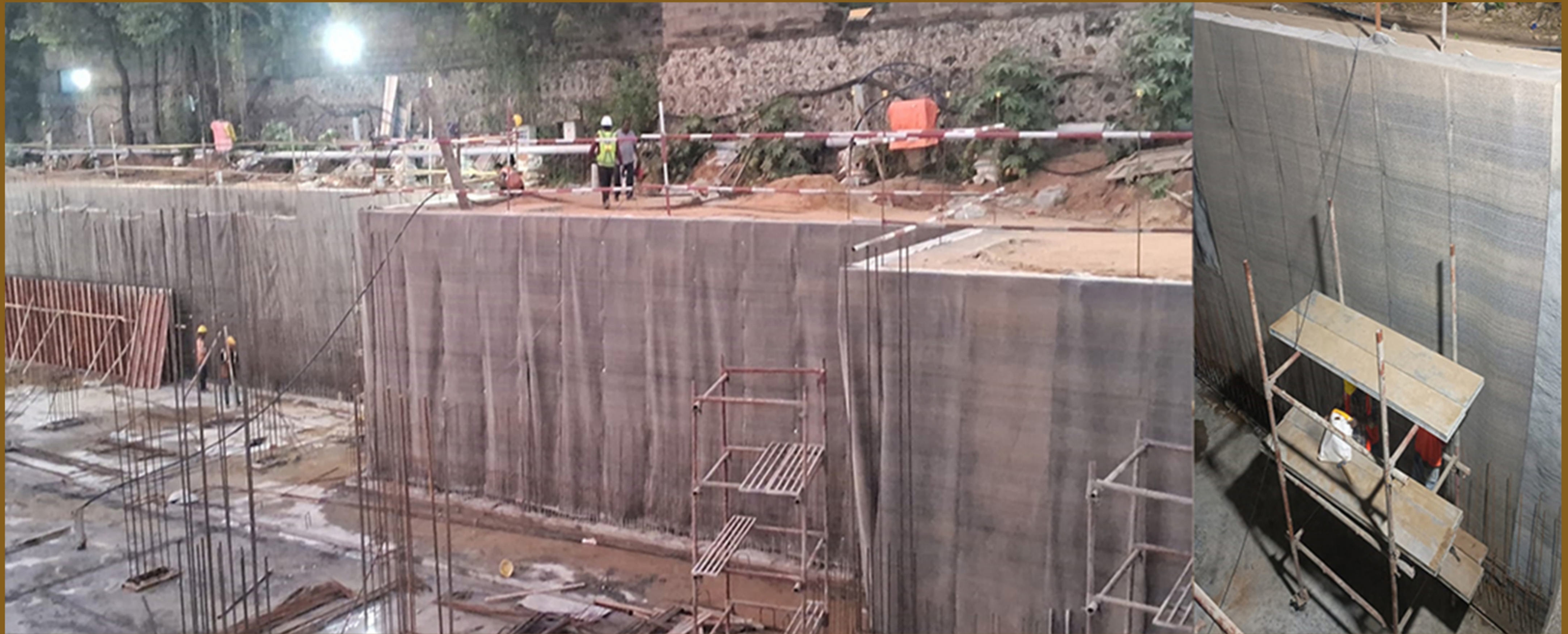
Block B RC-wall water Proofing work
