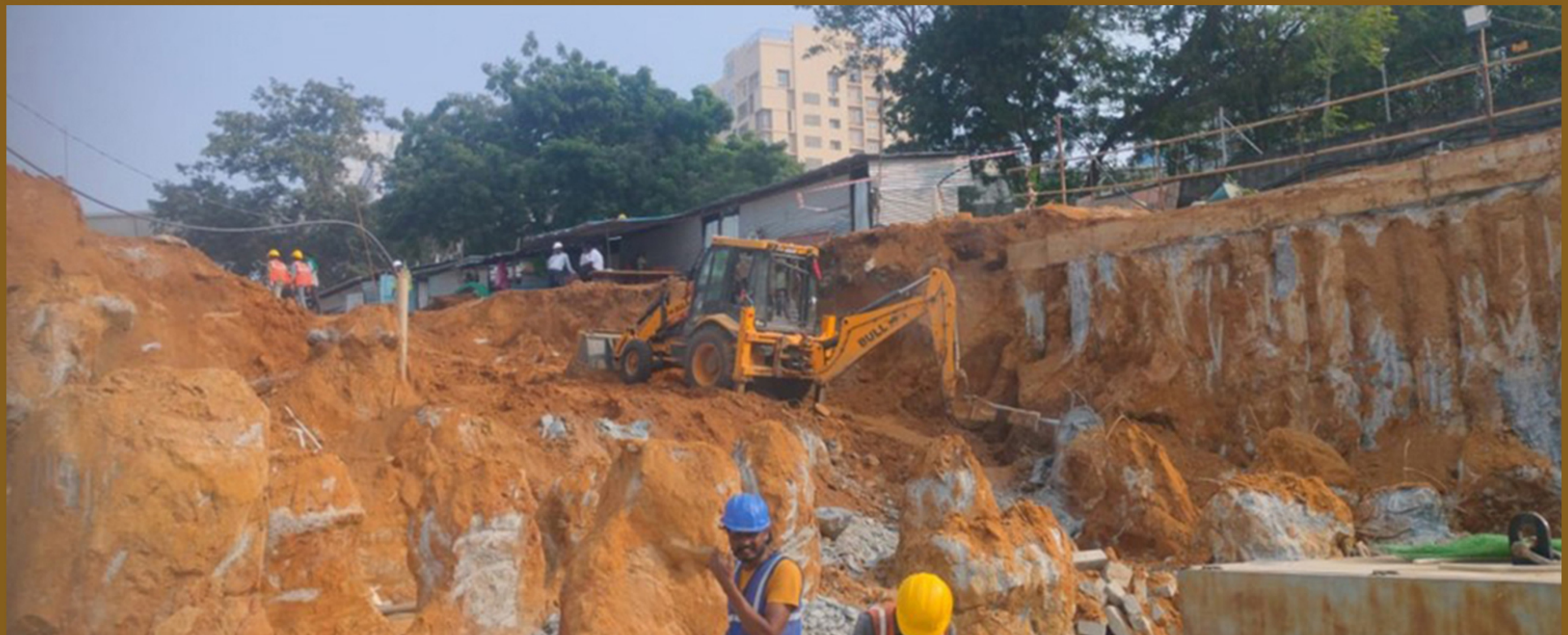
Block B short creating work
