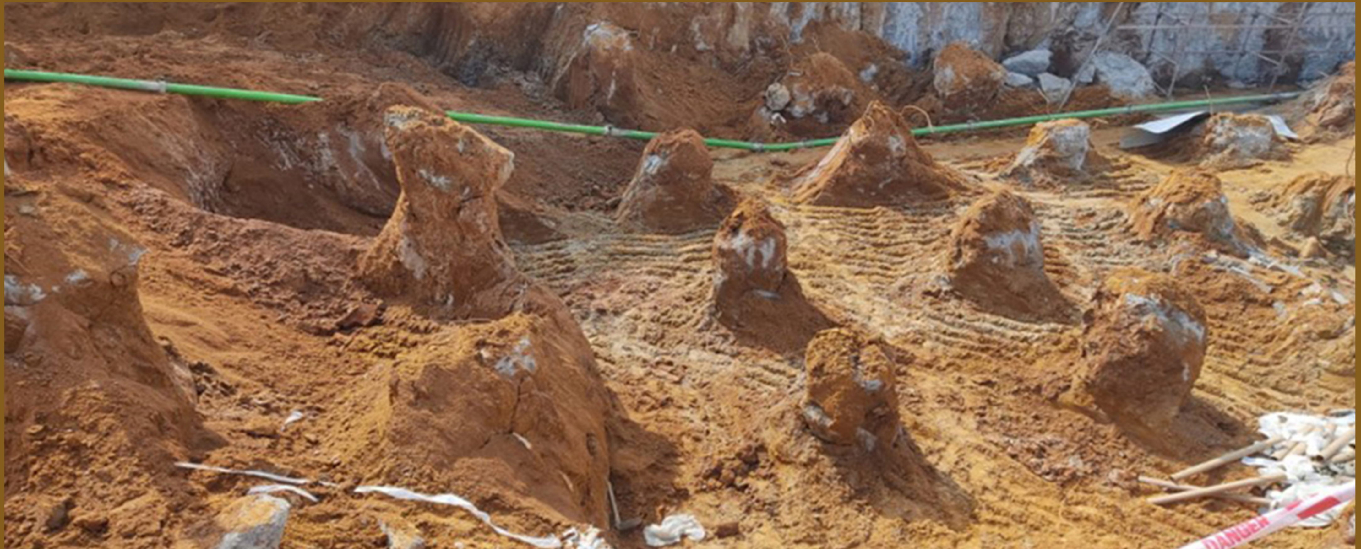
Block B stitch pipe area earth excavation works
