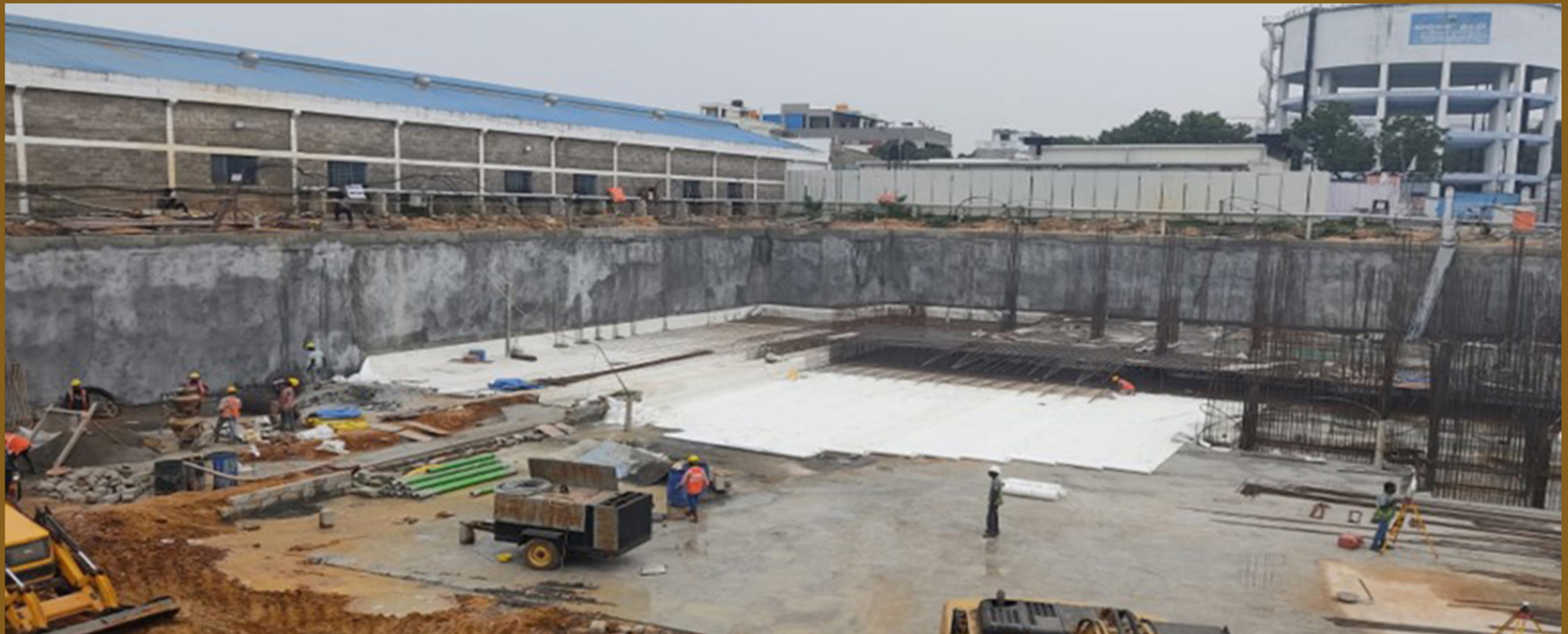
Block B raft water Proofing work
