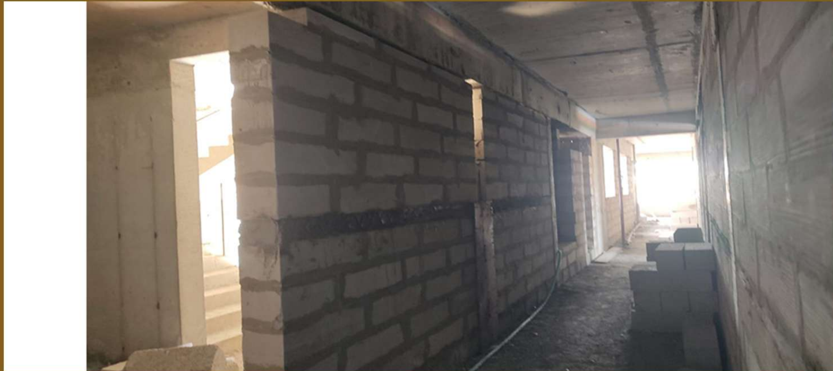
Block B –3rd Floor Block Work
