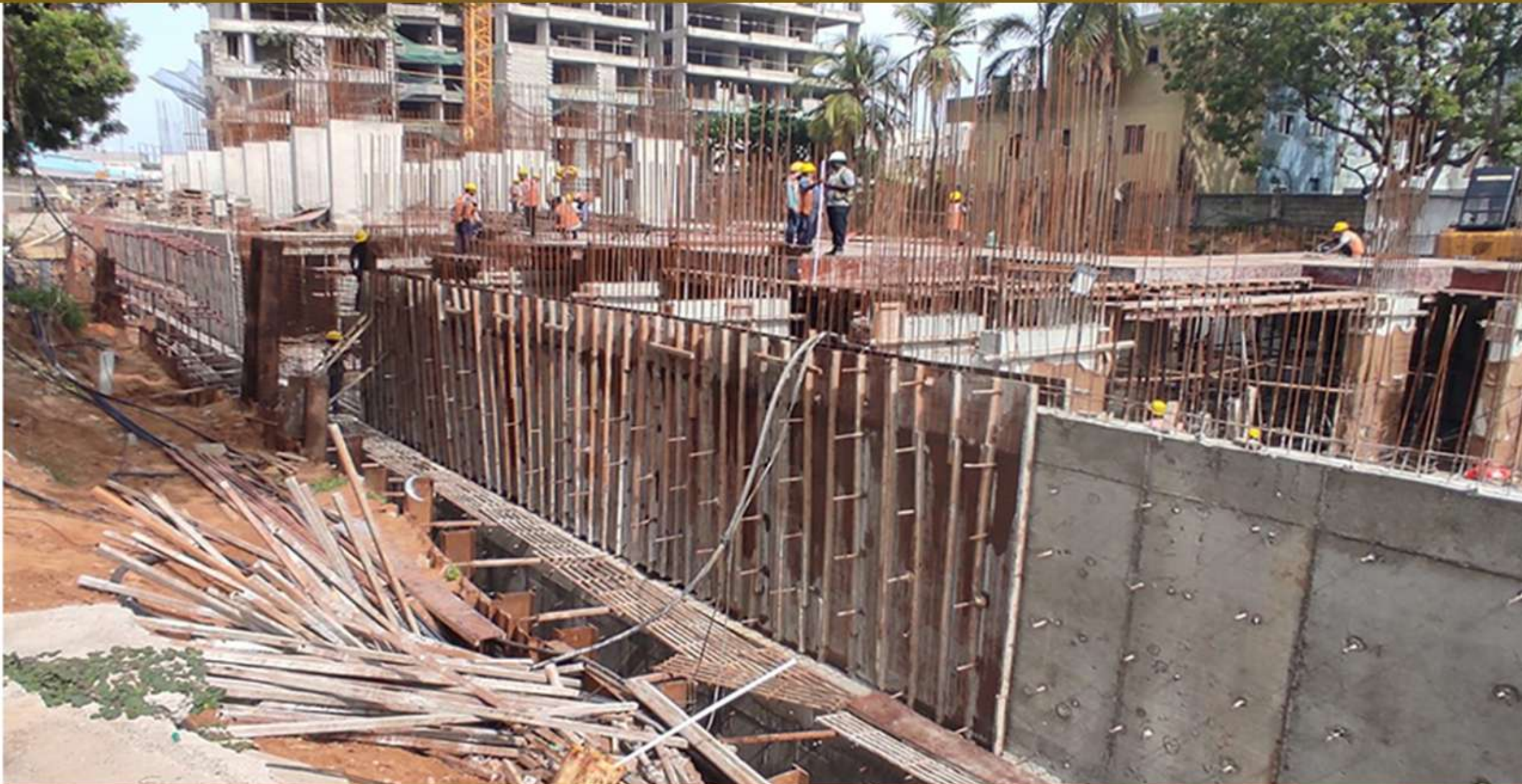
Block A – Upper Basement RC Wall Concrete Work Pour-2
