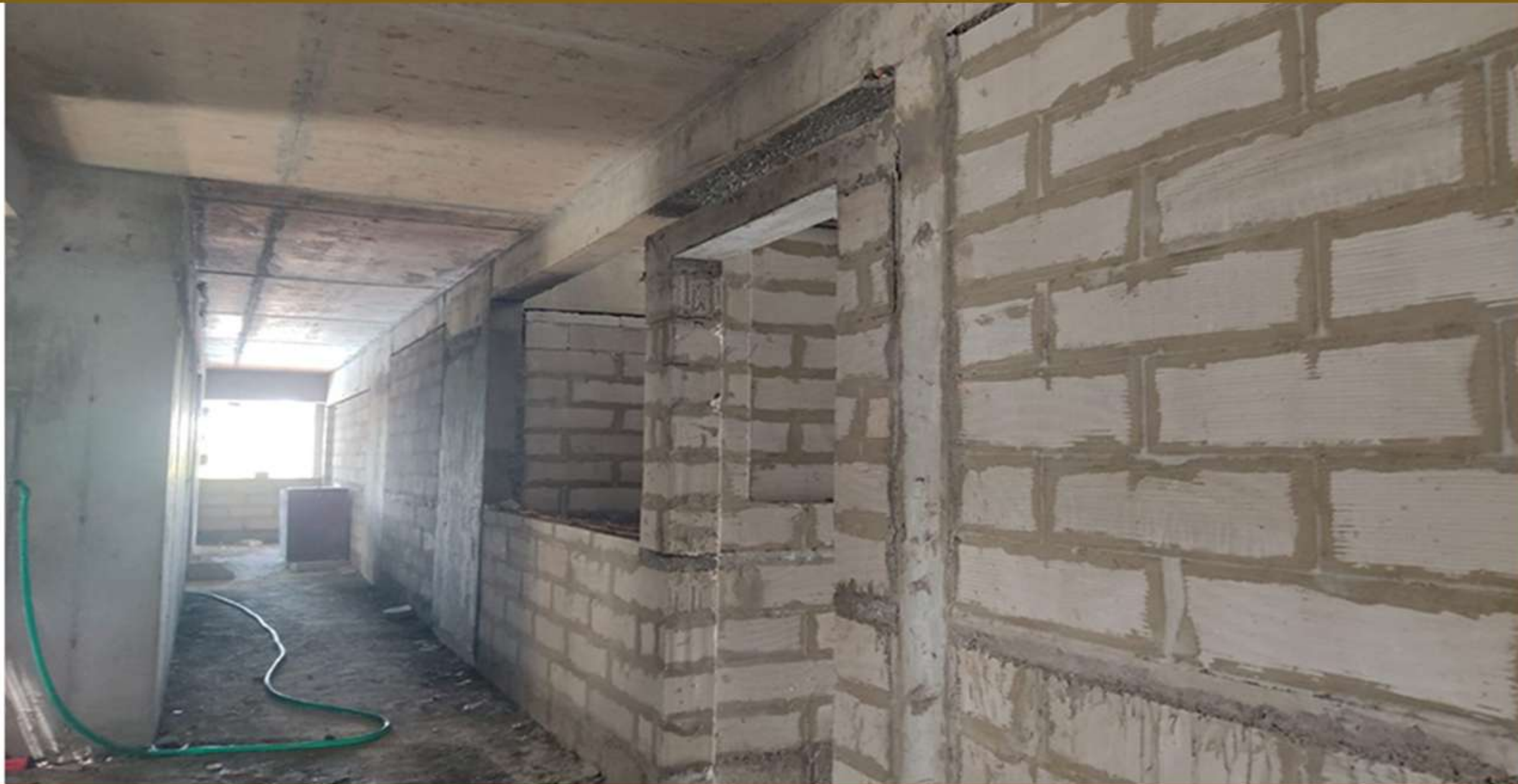
Block B –3rd Floor Block Work
