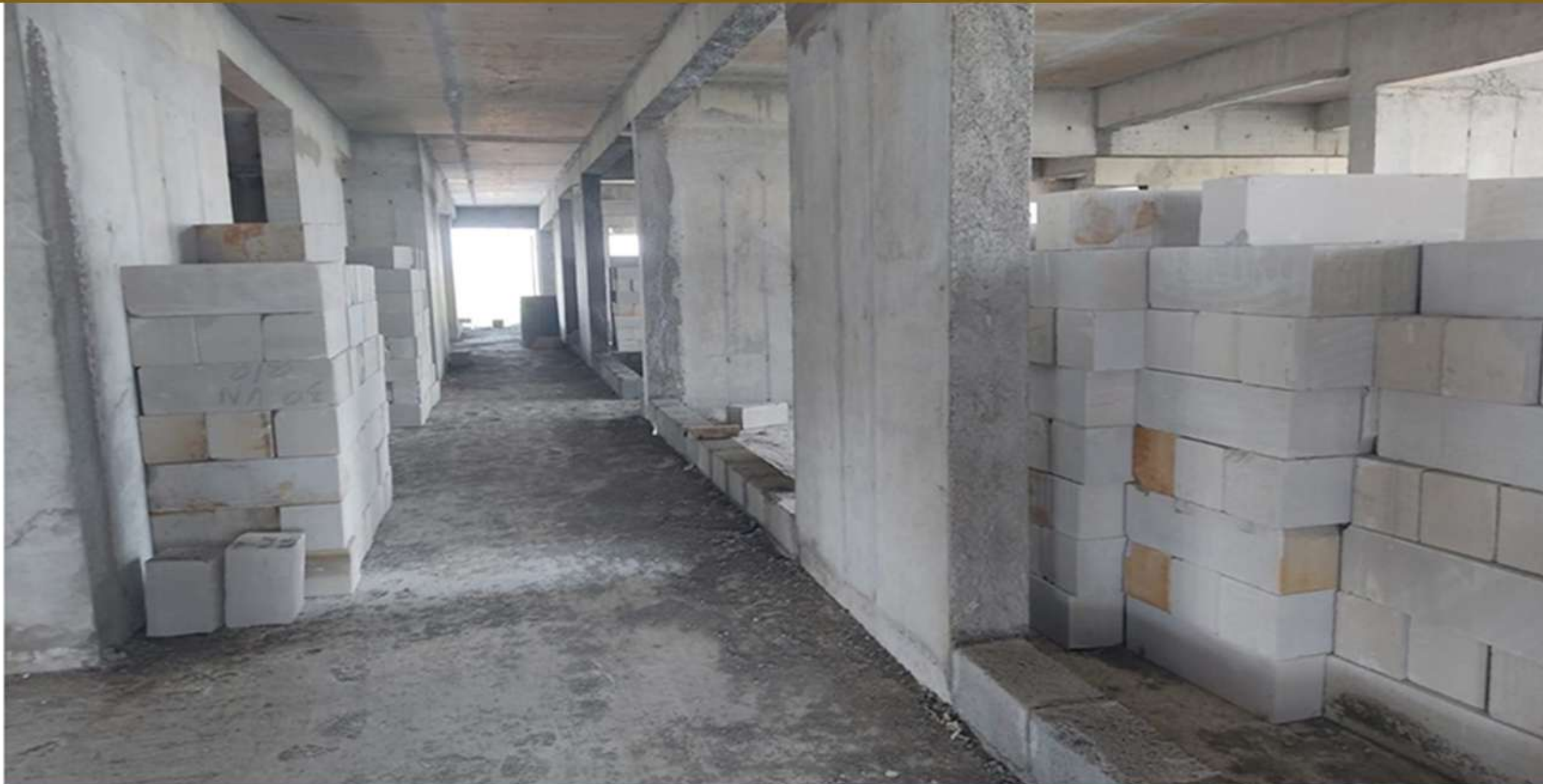
Block B – 4th Floor Block Work
