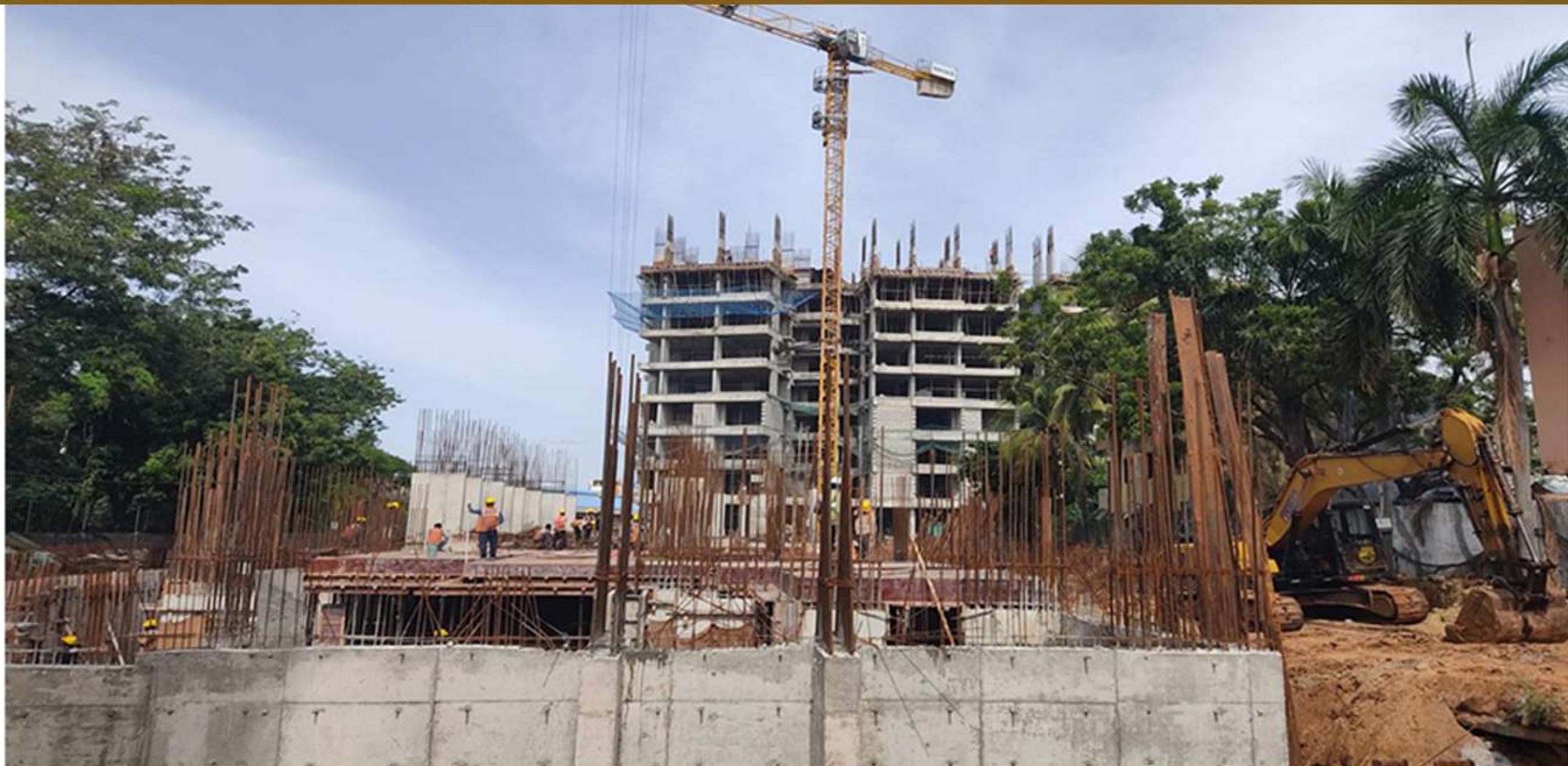
Block-A Front View
