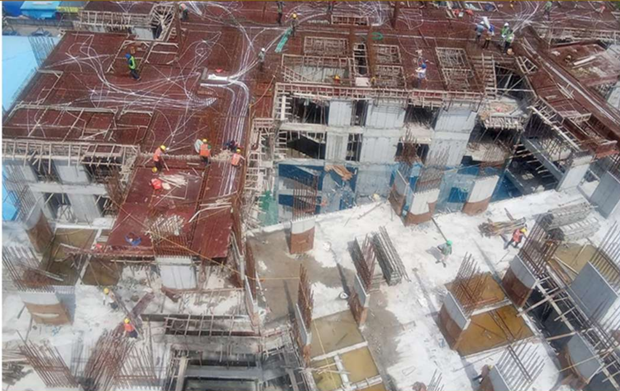
Block-B 8th Floor Roof Slab Work Pour-1
