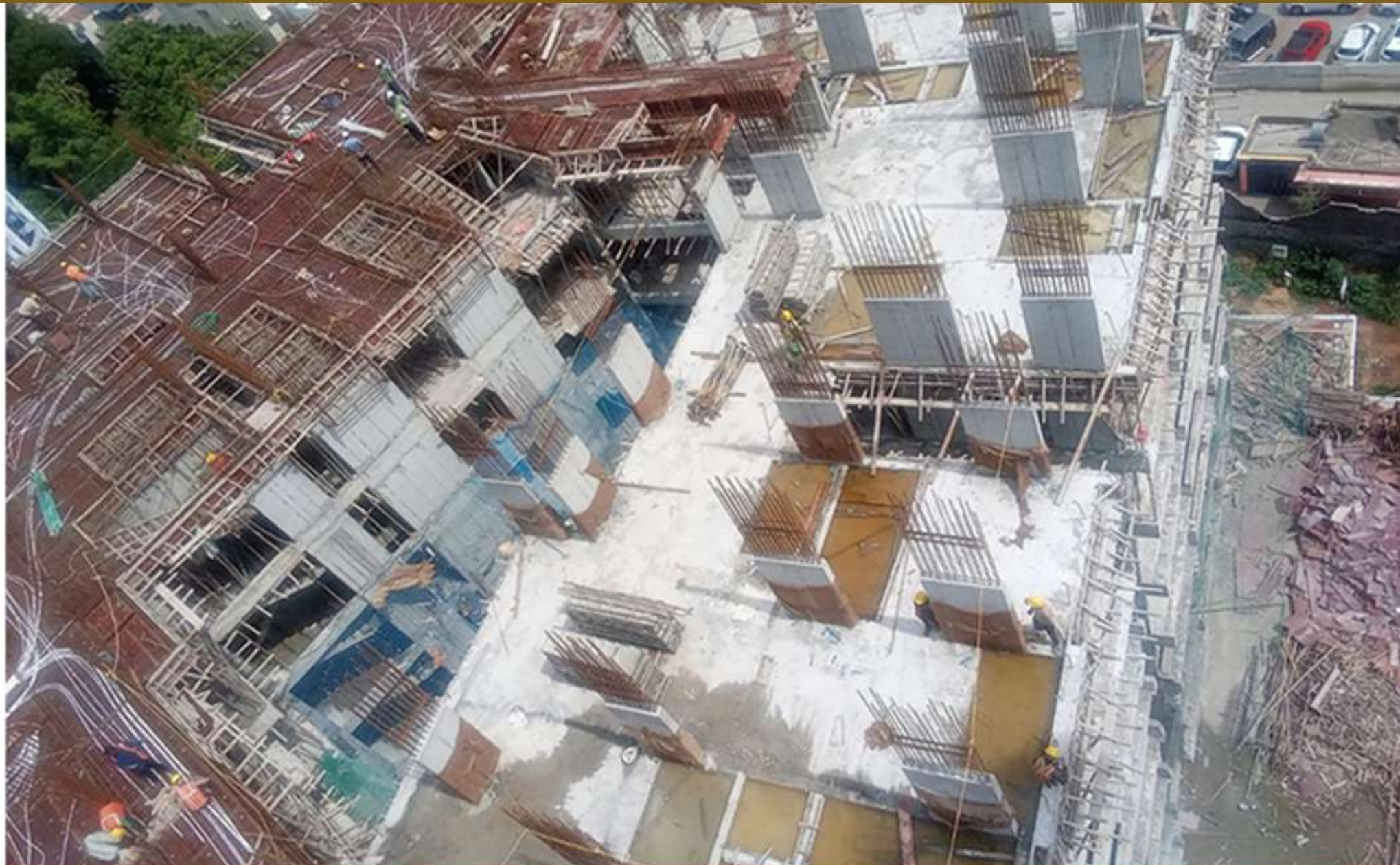
Block-B 8th Floor Column Concrete Work Pour-2
